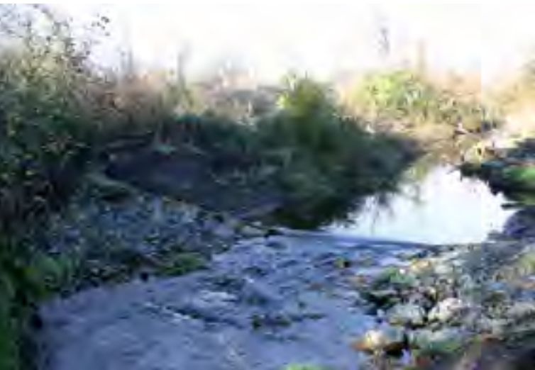
Water control structure on the outlet of Lake Rotomanuka North. Photo courtesy of Environment Waikato.
