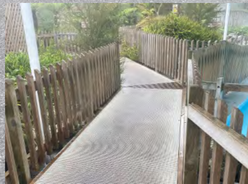
DECKING MATERIAL: FRP MICRO MESH GRATING
