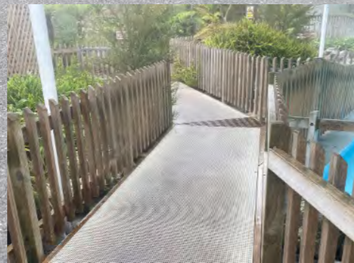
DECKING MATERIAL: FRP MICRO MESH GRATING
