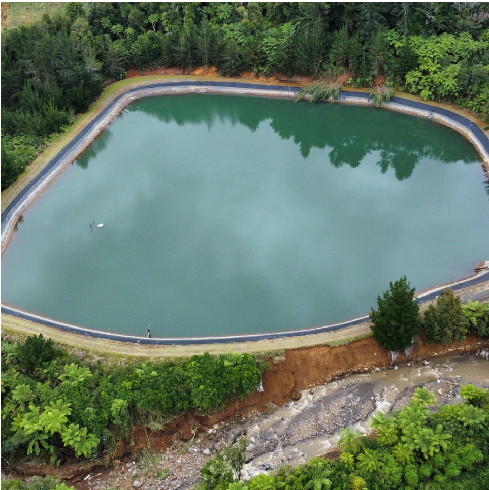
Pirongia's water supply, Te Tahi reservoir, as the draining process began.
