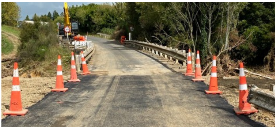
Mangauika Road bridge has reopened as of Friday, February 27.
