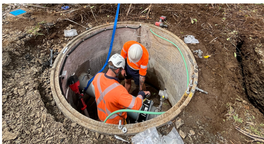
The team working on the new connection for Pirongia at Te Awamutu's Frontier Road.
