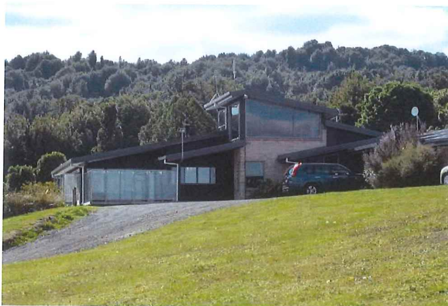
5. On site, viewing north to the Manu Tioriori Visitor Information Centre, and the lower rises of the Maungatautari reserve beyond.
