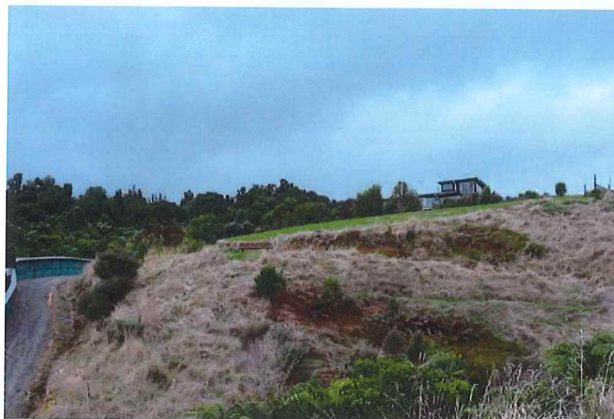
6. On site, viewing north-east from alongside Tuatara & Takahe enclosure. The proposed Education Centre is sited in the centre of the image against the planted bank. The Education Centre floor level is approximately 4.75 metres below the main floor level of Manu Tioriori (just visible).
