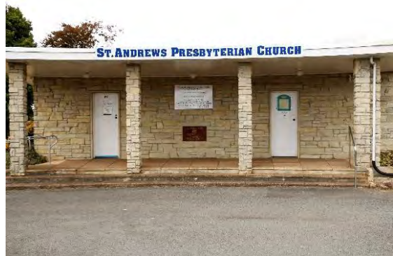
The old Administration Block
