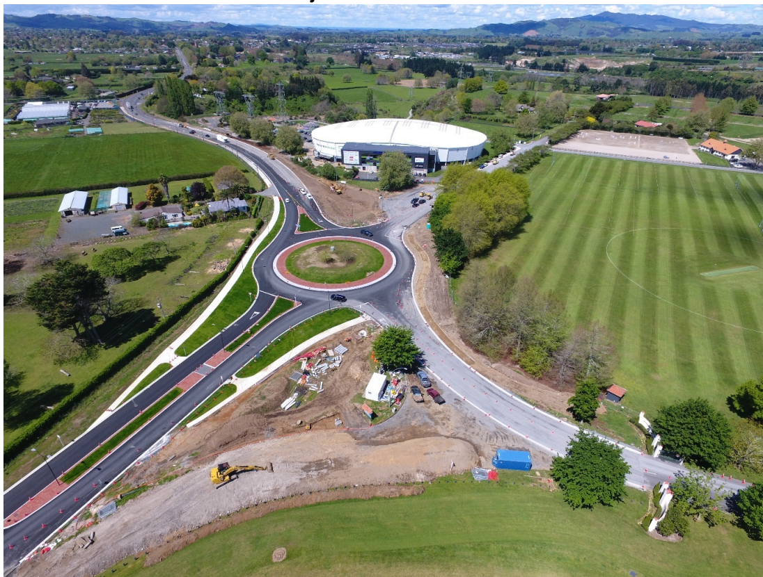
Hanlin Road 16 October 2020. Contractor is removing temporary roadway.
