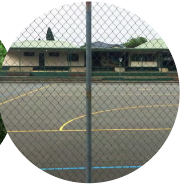
TE AWAMUTU NETBALL CENTRE
