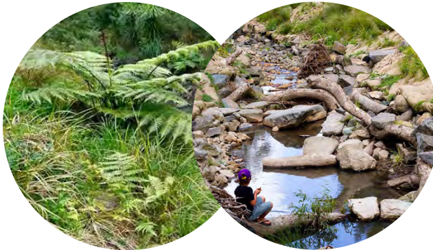
La Rosa Reserve Stream Daylighting. By Boffa Miskell.
