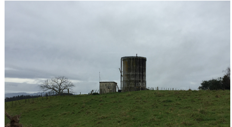
Open space adjacent to the village centre of Kihikihi
