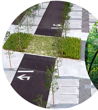
Multi-use Car Park Surface.
