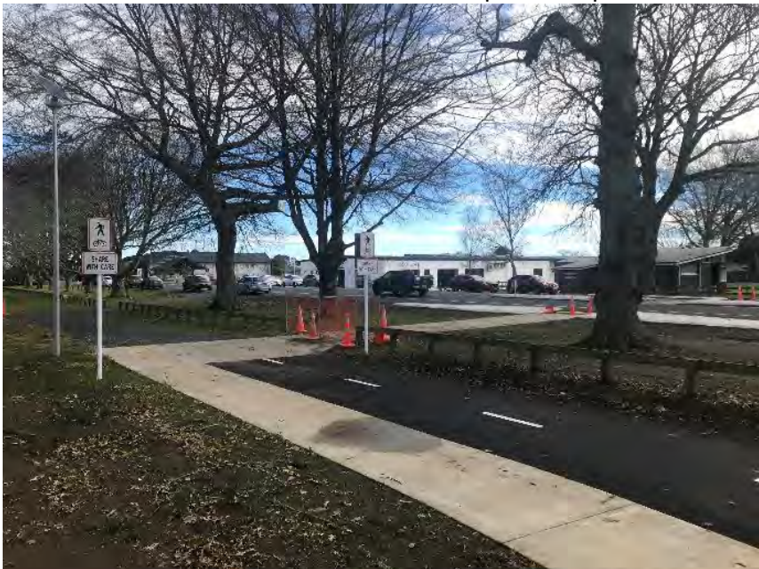
Current termination of path at point that recreational path crosses greenbelt. Paths cross Hamilton Road with new refuge islands.
