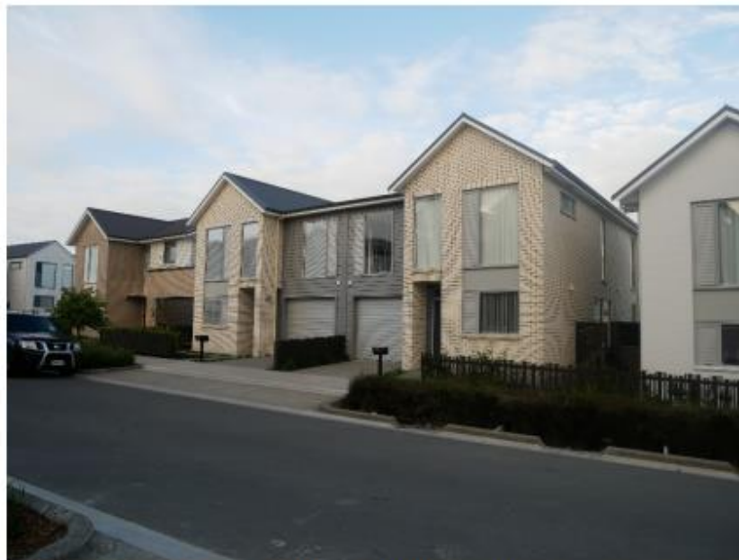
Figure 4 - Hobsonville Duplex Housing
