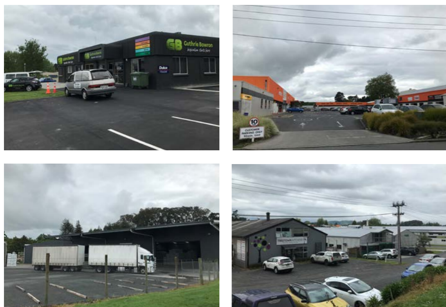
Figure 5. Existing built form and character
