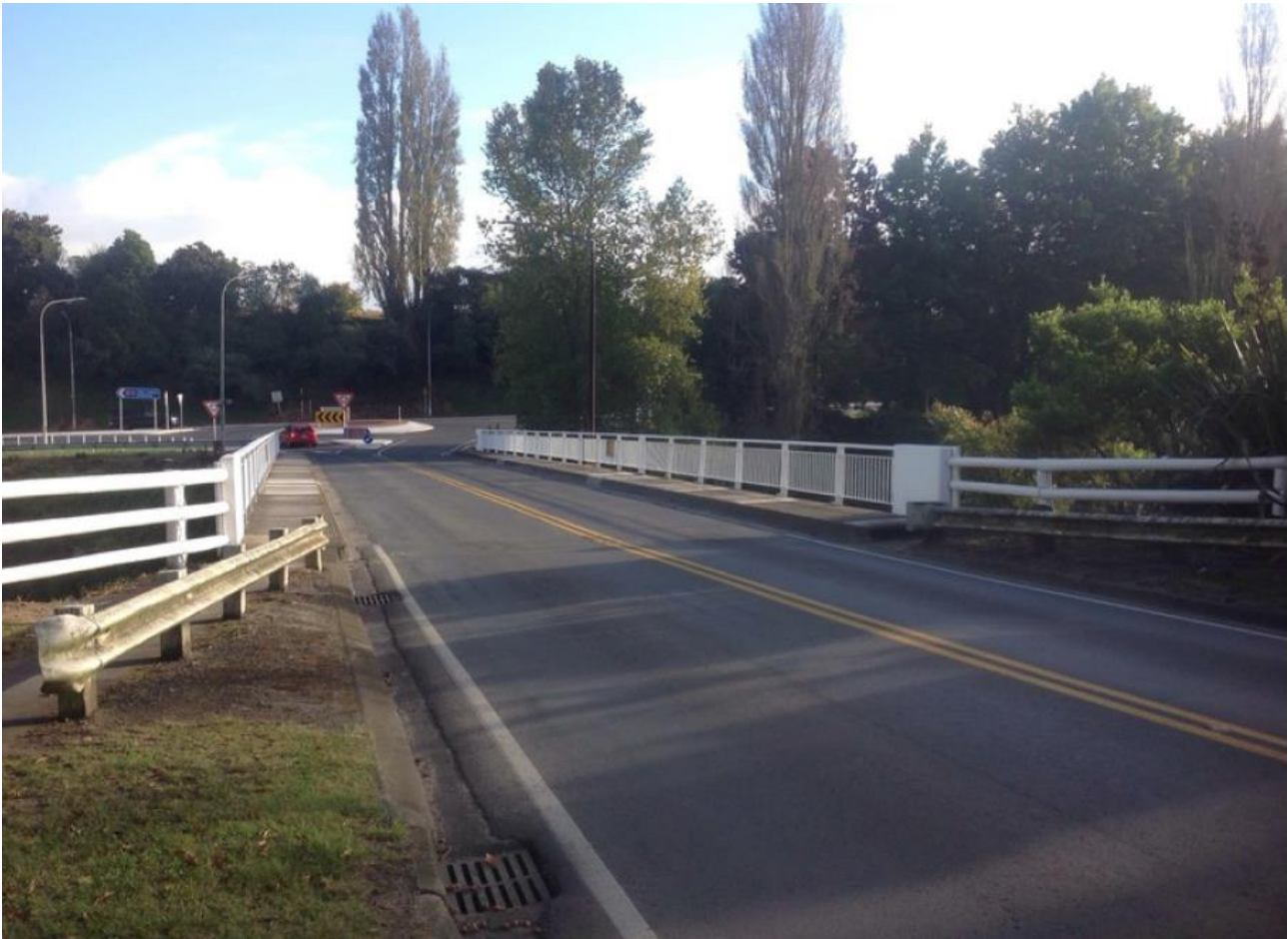
Figure 3: Shakespeare Street Bridge
