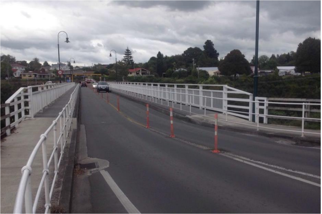
Figure 2: Victoria Street Bridge
