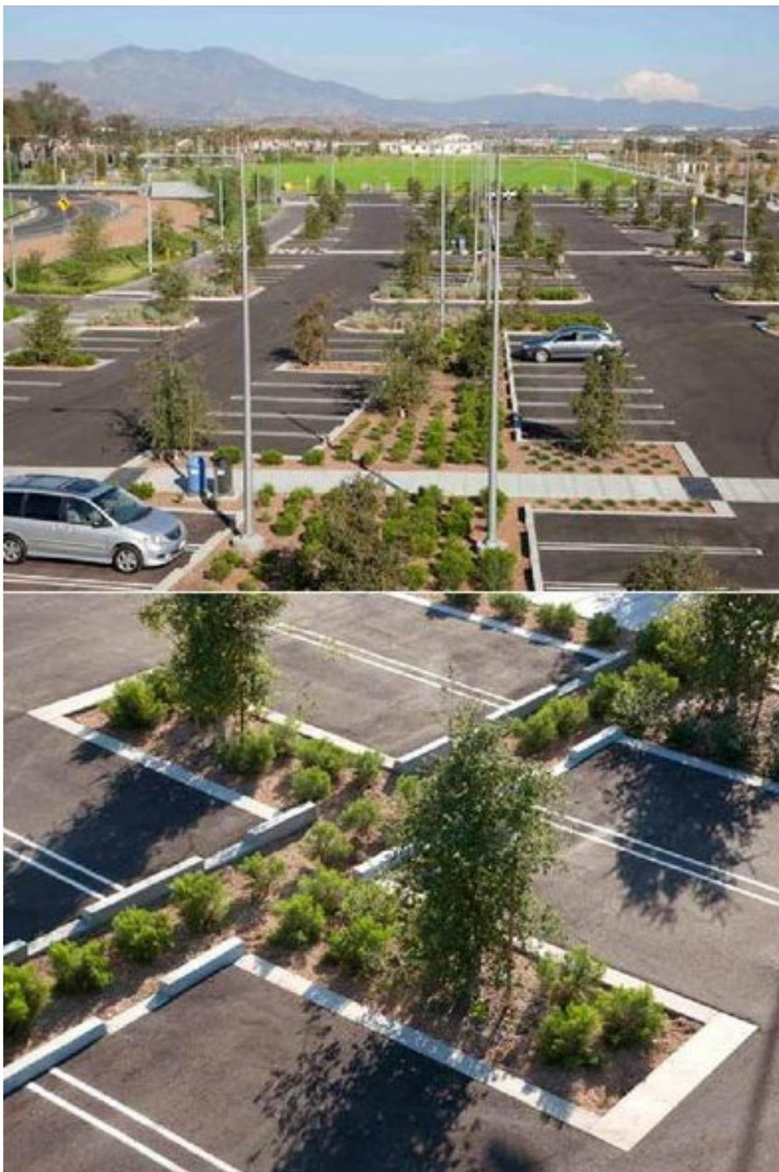
**Figure 7: Landscaping helps minimise the visual impact of the car park, breaking up the large areas of asphalt. Added environmental benefits include less storm-water runoff, increased amenity and shade for parked cars.**
