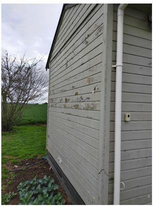
Photo 2: Cottage (feature 2), with paint in deteriorated condition
