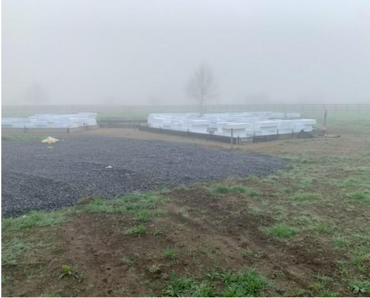
Photo 1: Proposed house building pad, prior to intended concrete pour, 2022.
