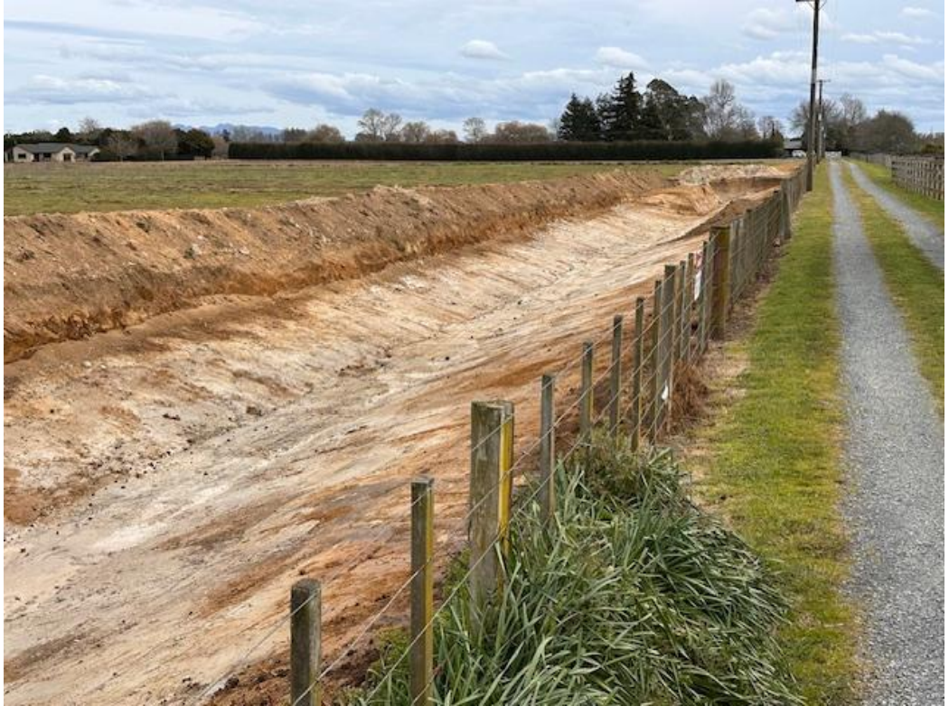
Figure 2: View down Gundesen driveway towards Peake Rd, showing the stormwater pond being formed on Area 6.
