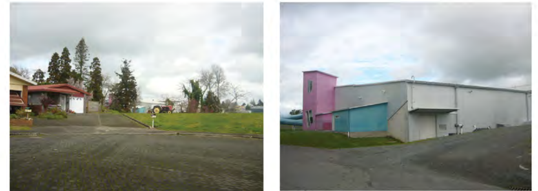
Figure 33: View looking towards the Mangaohoi Stream from Shanel Place and the back of the Events Centre facing on to the stream walkway. Future development facing the stream would raise the amenity and address CPTED issues.
