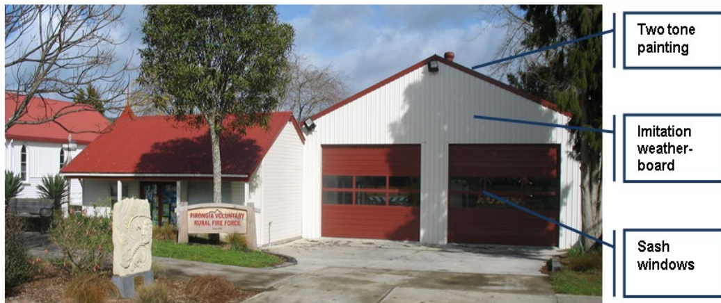
Photo 5: Continuation of architectural details in a modern addition to a historical building, Pirongia Voluntary Rural Fire Force, Franklin Road.
