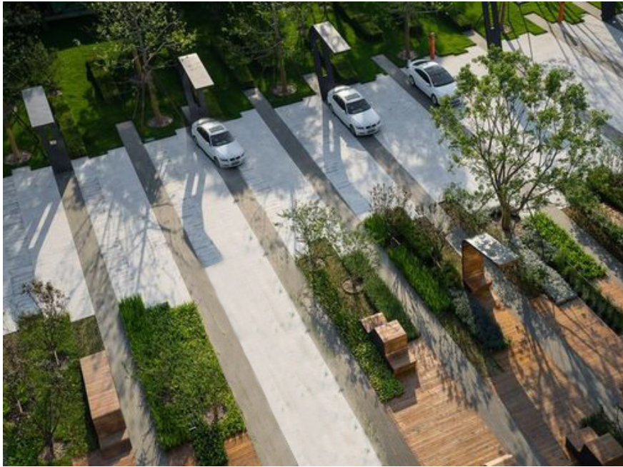
Image supporting S20.3.15.1(h) - Right: Image showing a carpark with charging stations for the use of electric cars.
