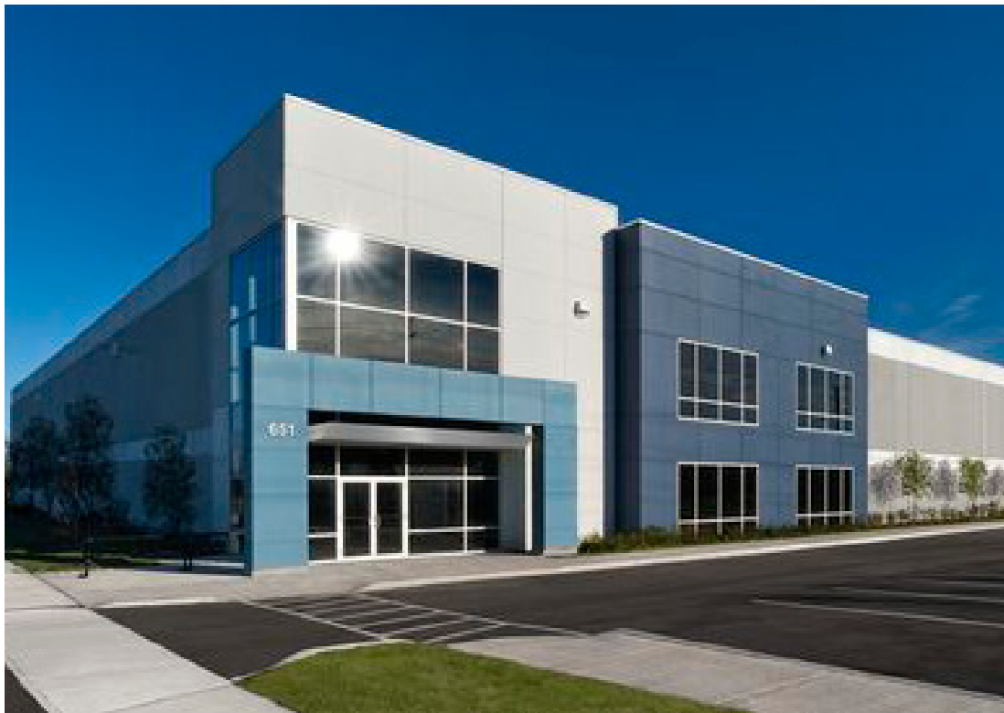
Figure 13 12: Varying setbacks and a mix of neutral coloured façades help reduce the dominance of the building.
