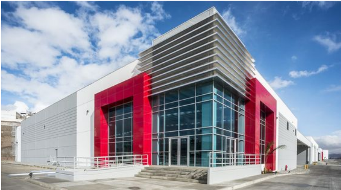
Figure 12 11: Coloured concrete panels and glazed facade help break up the scale of the building.
