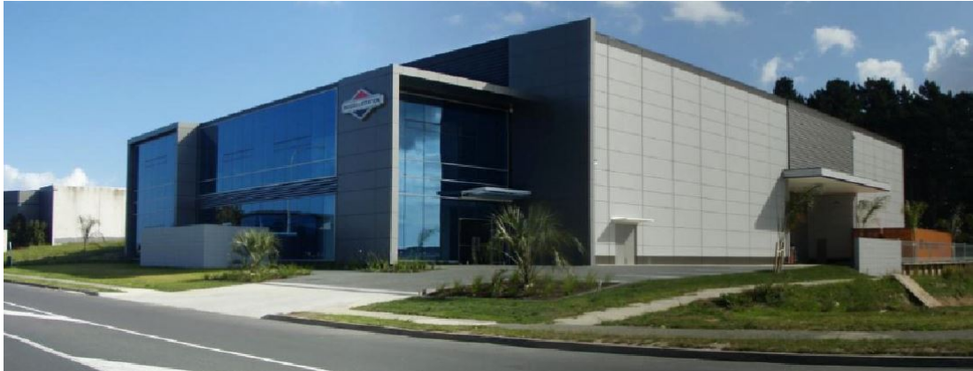
Figure 10 9: This development incorporates good pedestrian links, high quality amenity landscaping and good passive surveillance around the building.
