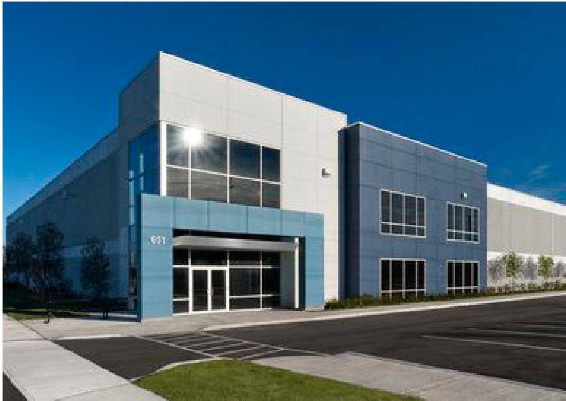
Figure 12: Varying setbacks and a mix of neutral coloured façades help reduce the dominance of the building.
