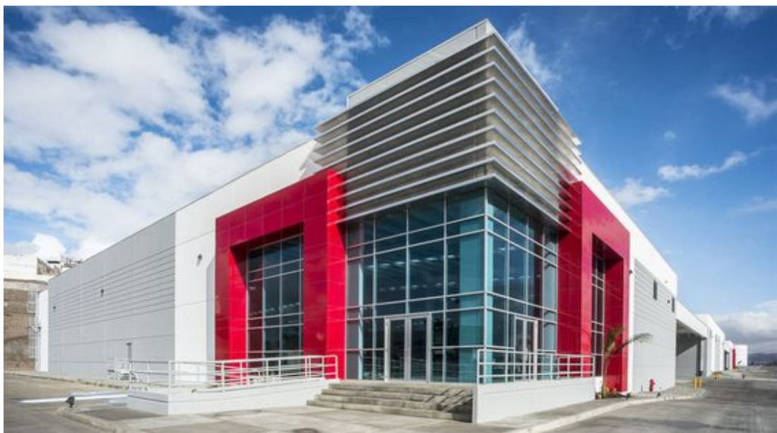
Figure 11: Coloured concrete panels and glazed facade help break up the scale of the building.
