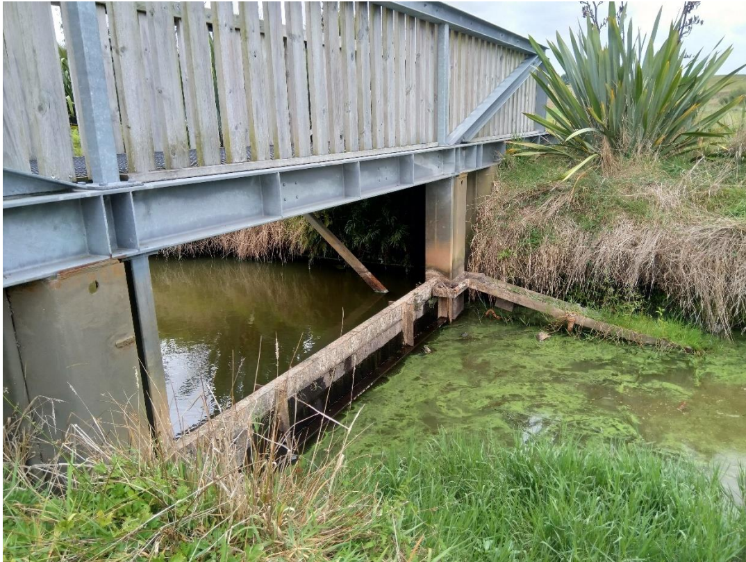
Figure 23: Fish ladder at the lake outlet weir overgrown with grasses and herbaceous weeds. Taken on 16 th March 2021.
