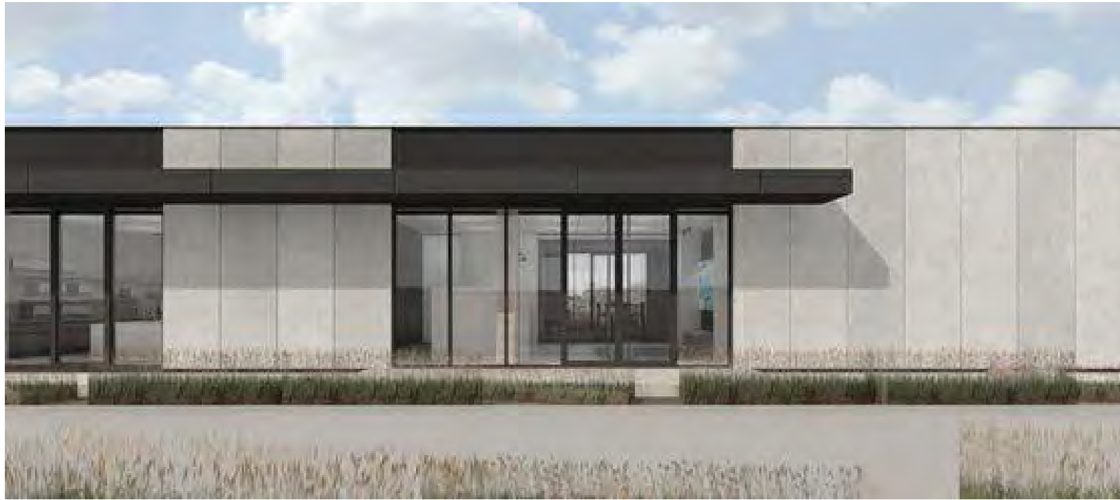
precast cladding (textured), glazed sliding entry doors and aluminium composite cladding + canopy
