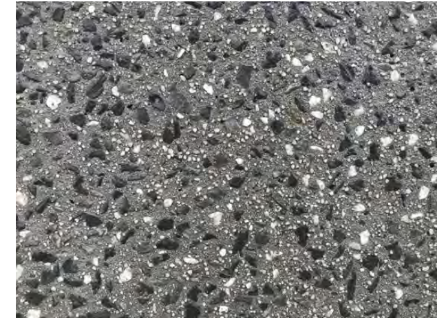
exposed aggregate exterior slab + steps
