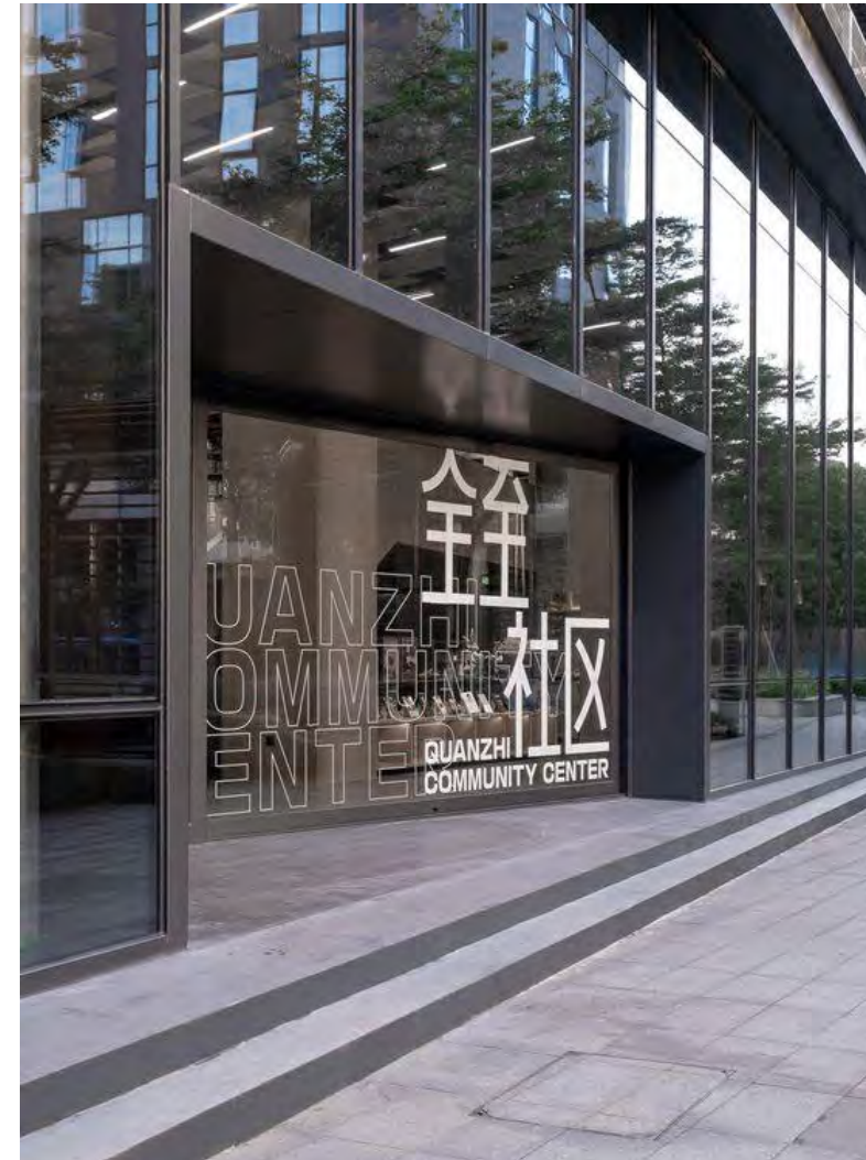
glazed facade, exposed aggregate exterior slab + steps, entry portals recessed back into building footprint
