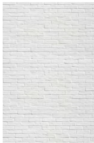
bagged brick cladding paint finish - (building C only)
