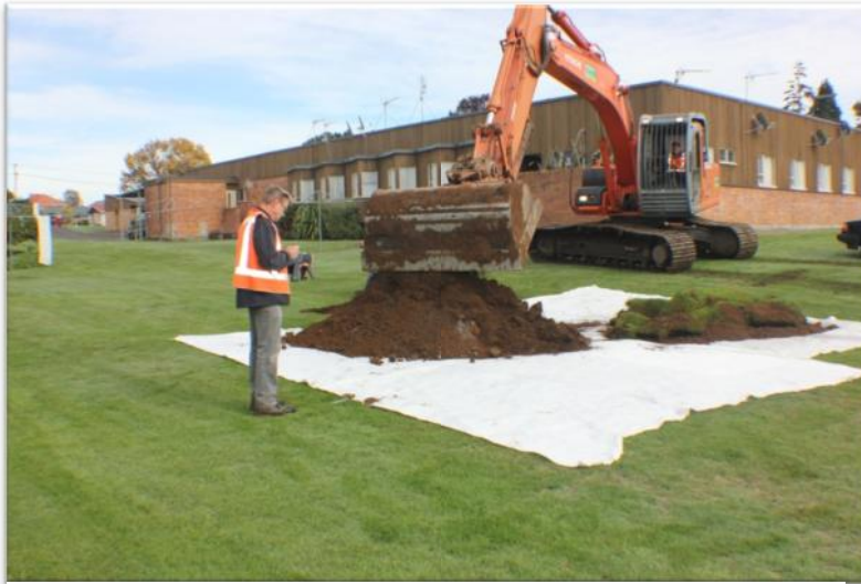
Figure 8 Sampling the anomalies found in the radargrams
