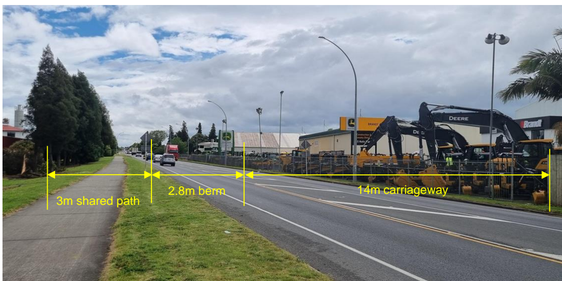
FIGURE 7: SH1C TYPICAL CROSS-SECTION LOOKING NORTH
