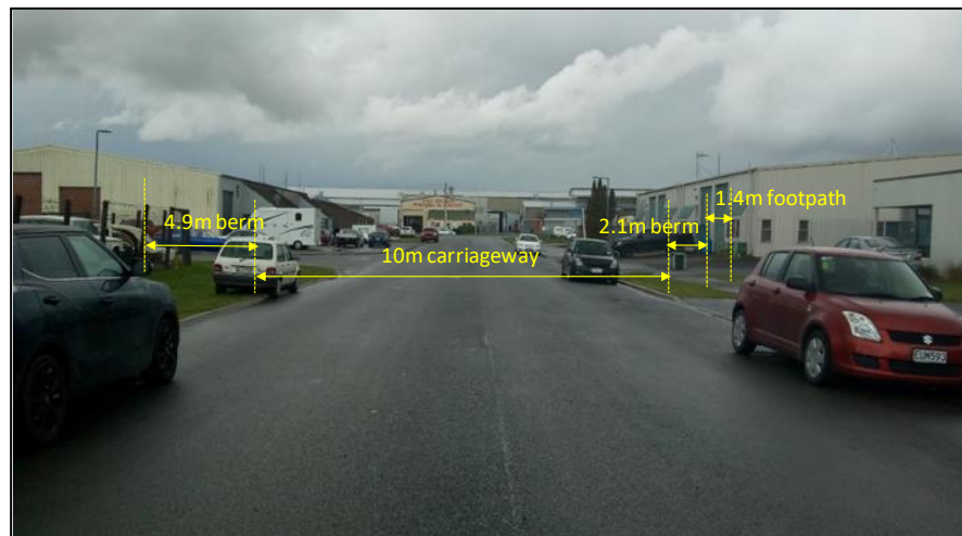
FIGURE 2: TYPICAL CROSS-SECTION OF WICKHAM STREET LOOKING NORTH
