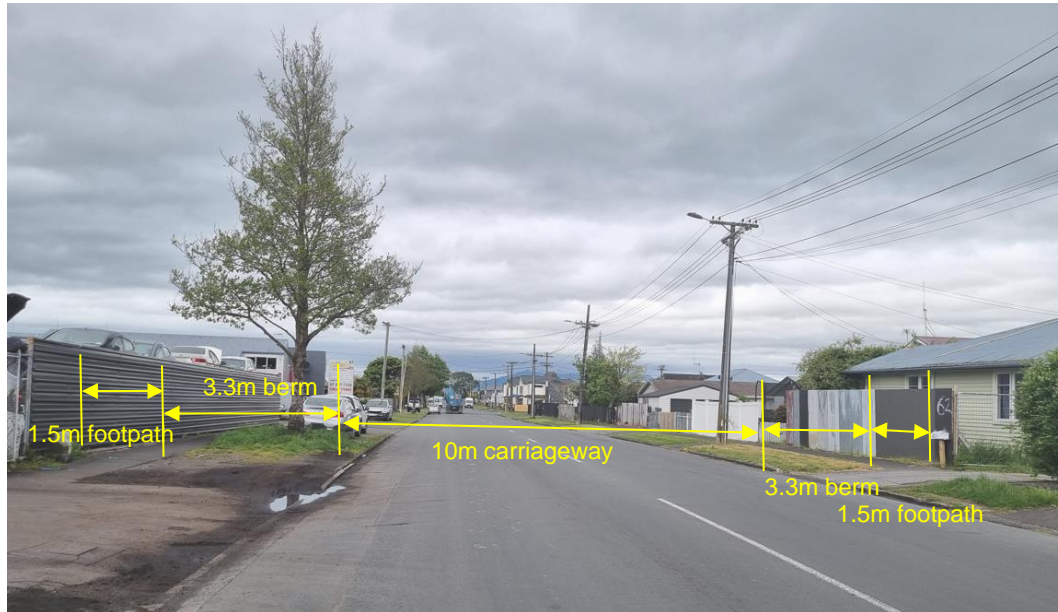
FIGURE 5: HIGGINS ROAD TYPICAL CROSS-SECTION LOOKING SOUTH
