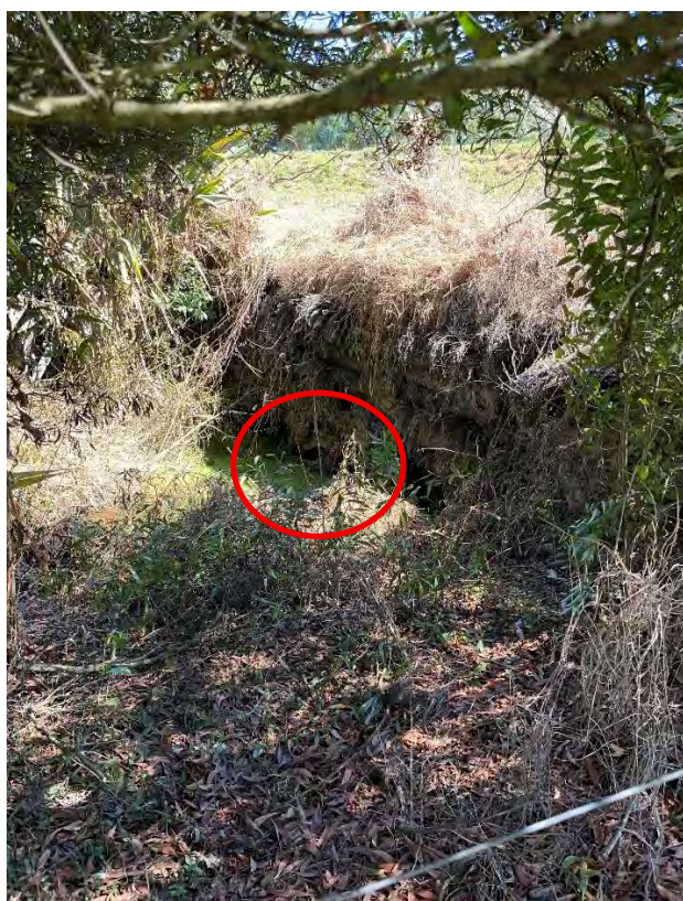
Figure 1: Culvert 3 Inlet – 29 Feb 2024
