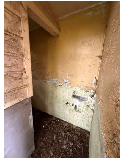
Toilet Block - Internal
