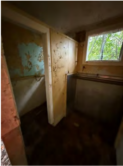
Toilet Block - Internal
