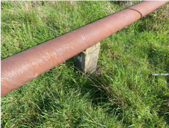
Southern pipeline with concrete pile (Type 5 (2))
