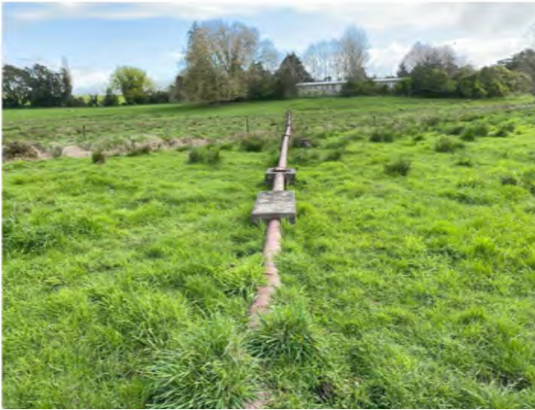
Southern pipeline with concrete casing (Type 3 (2))
