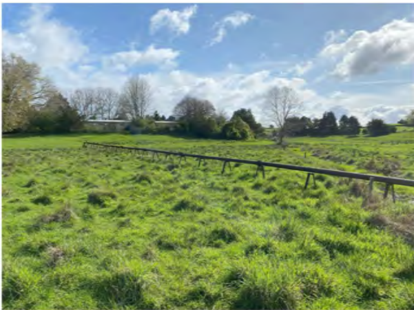
Southern pipeline with footings (Type 6)
