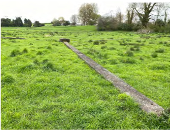
Eastern pipeline within concrete chamber (Type 3)
