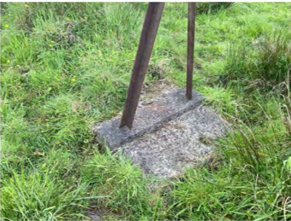
Pipeline situated on concrete foundation (Type 6)
