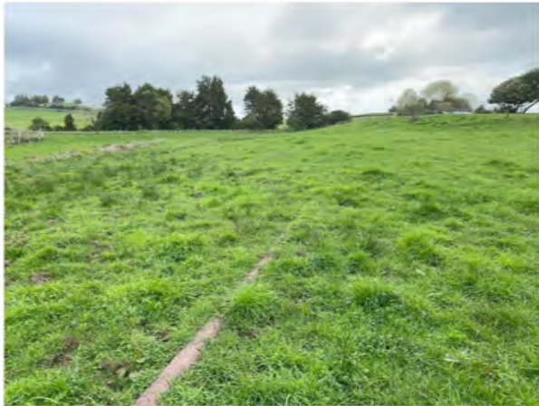
Westernmost pipeline below ground level (Type 2)
