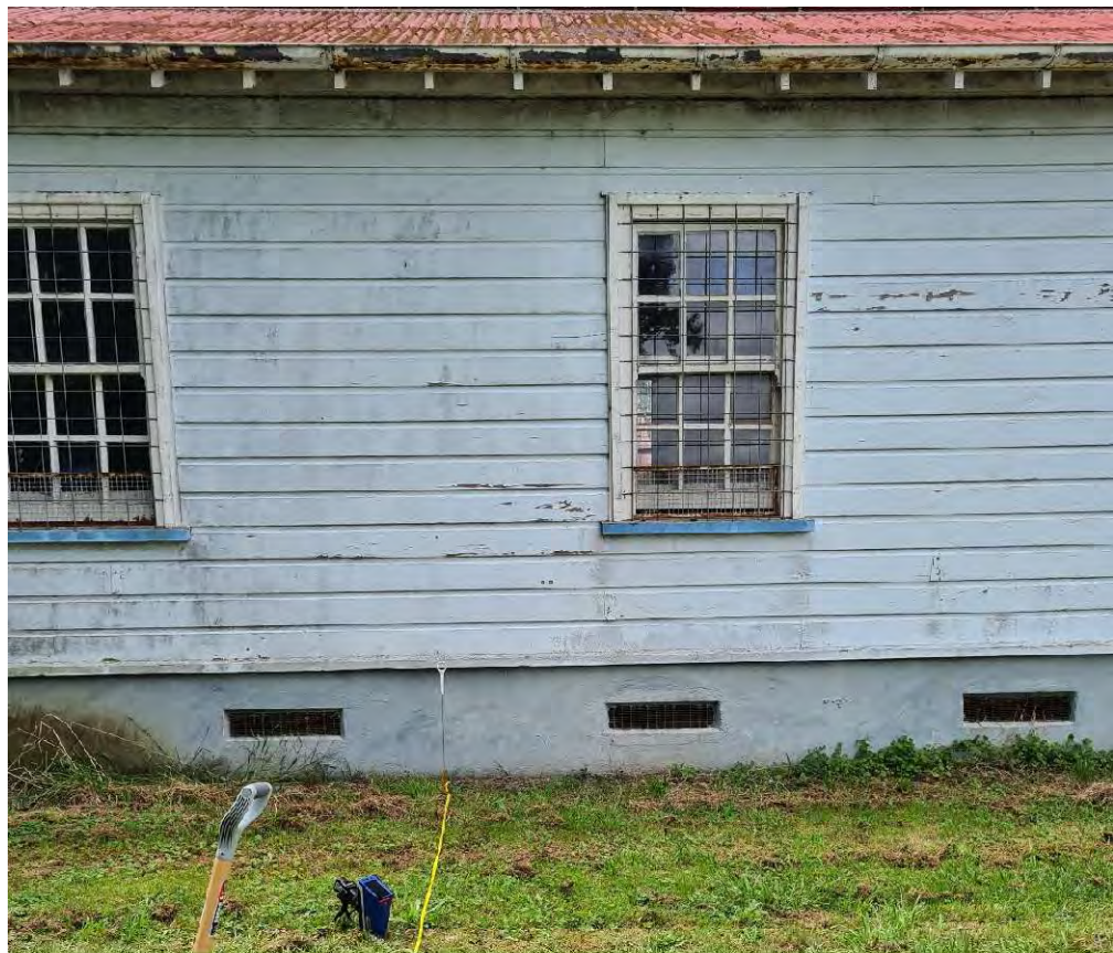
Plate X14: Looking east towards western wall of B15.
