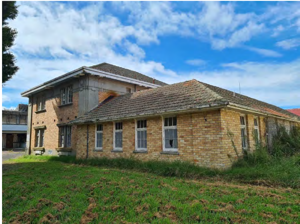
Plate X10: Looking southeast towards northwest corner of B10.
