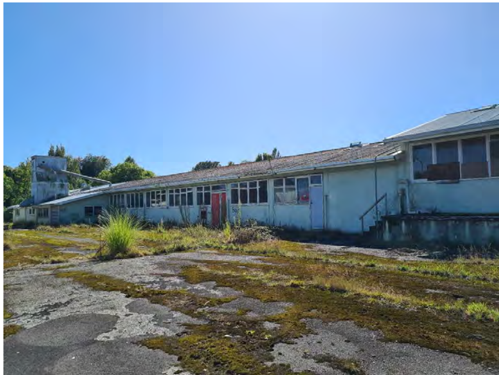
Plate X46: Looking north towards B63.
