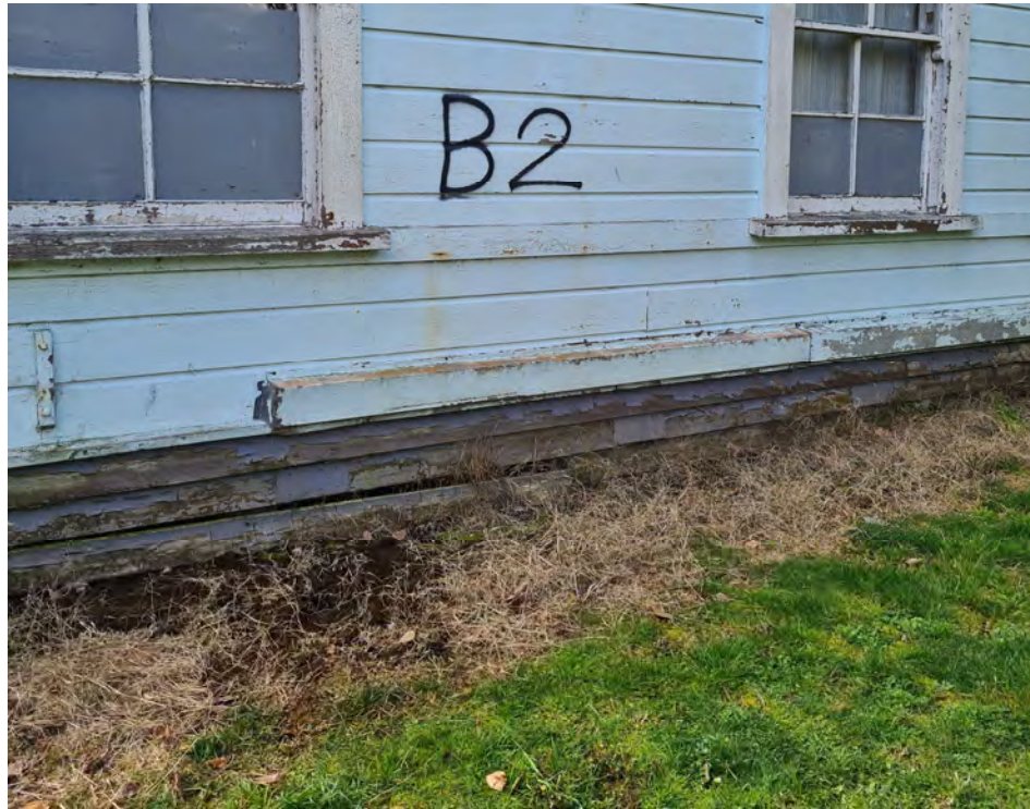
Plate X1: Looking towards northwest corner of building B2
