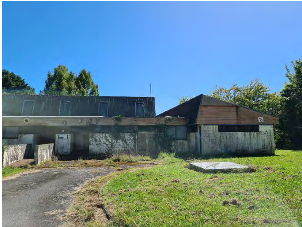
Plate X37: Looking north towards B50.
