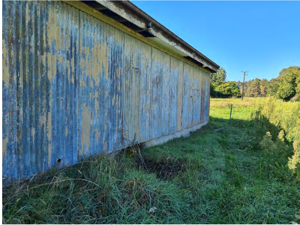
Plate X3: Looking towards southwest corner of building B59
