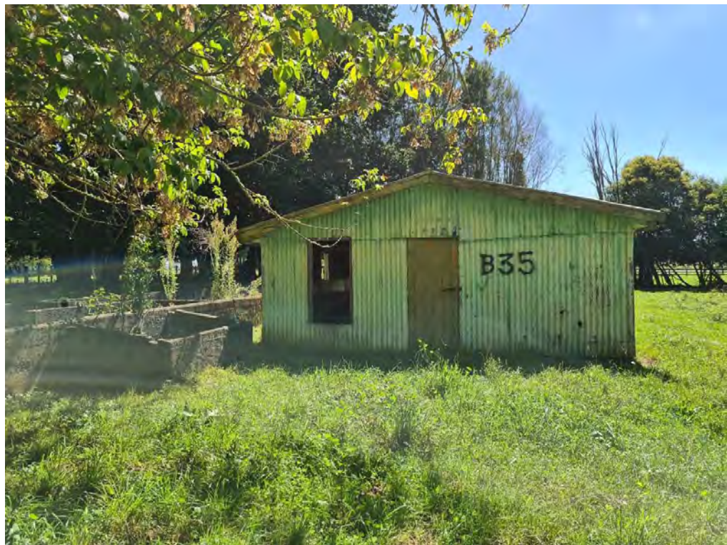
Plate X28: Looking north towards B35.
