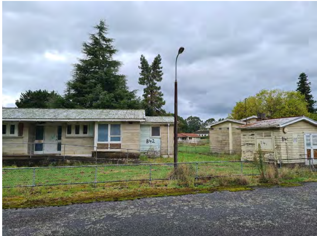
Plate X31: Looking north towards B41 and B42.
