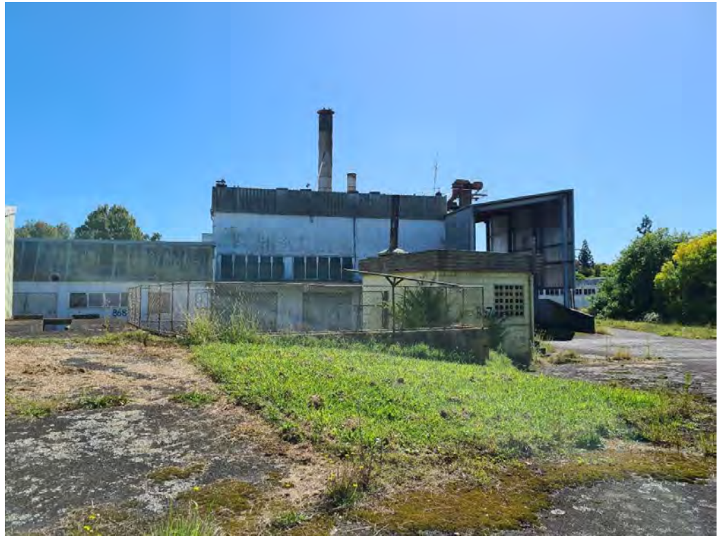
Plate X49: Looking north towards B67 and B68.
