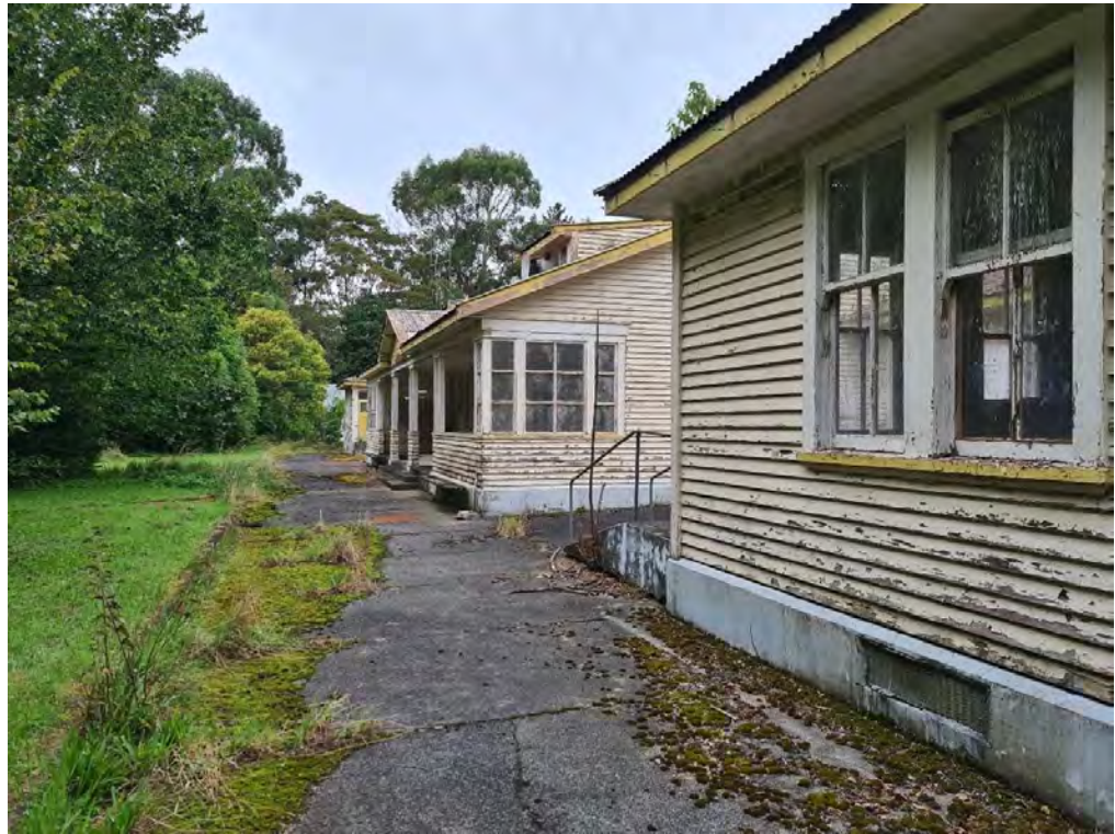
Plate X21: Looking southwest from northwest corner of B23.
