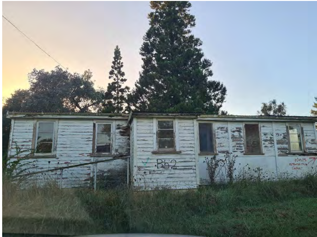
Plate X39: Looking east towards B52.
