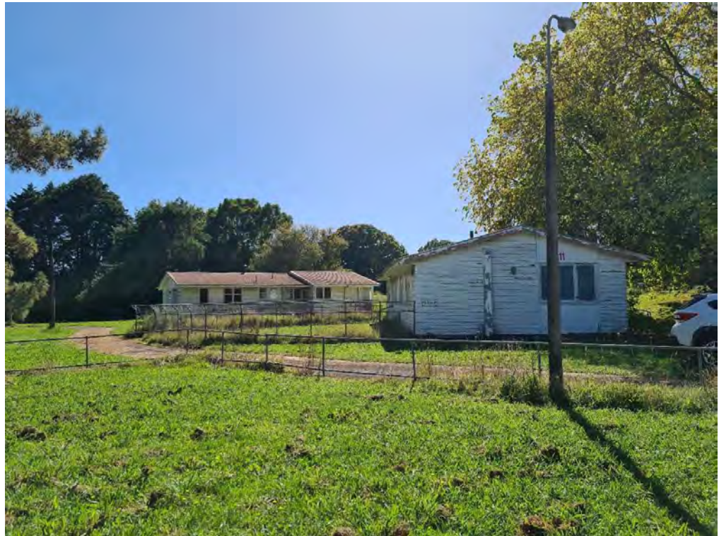
Plate X33: Looking north towards B45 and B46.
