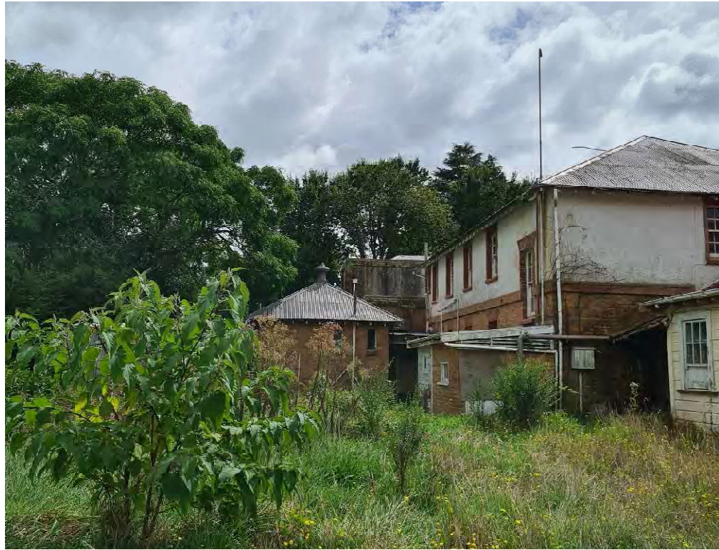
Plate X13: Looking north towards southwest corner of B12.
