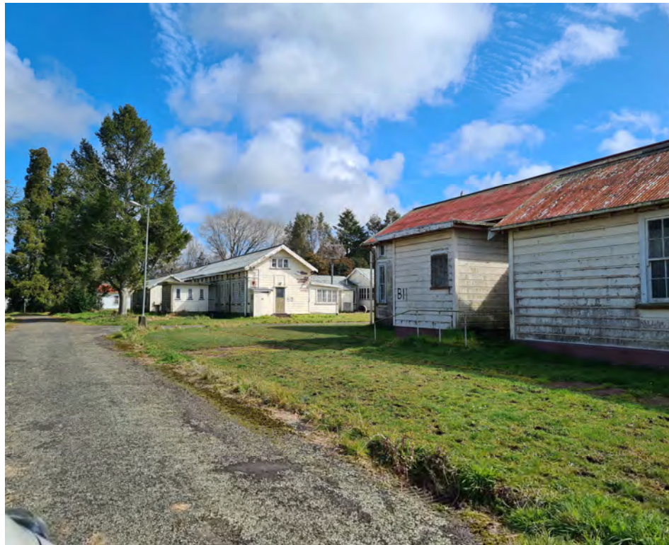
Plate X2: Looking towards southwest corner of building B11
