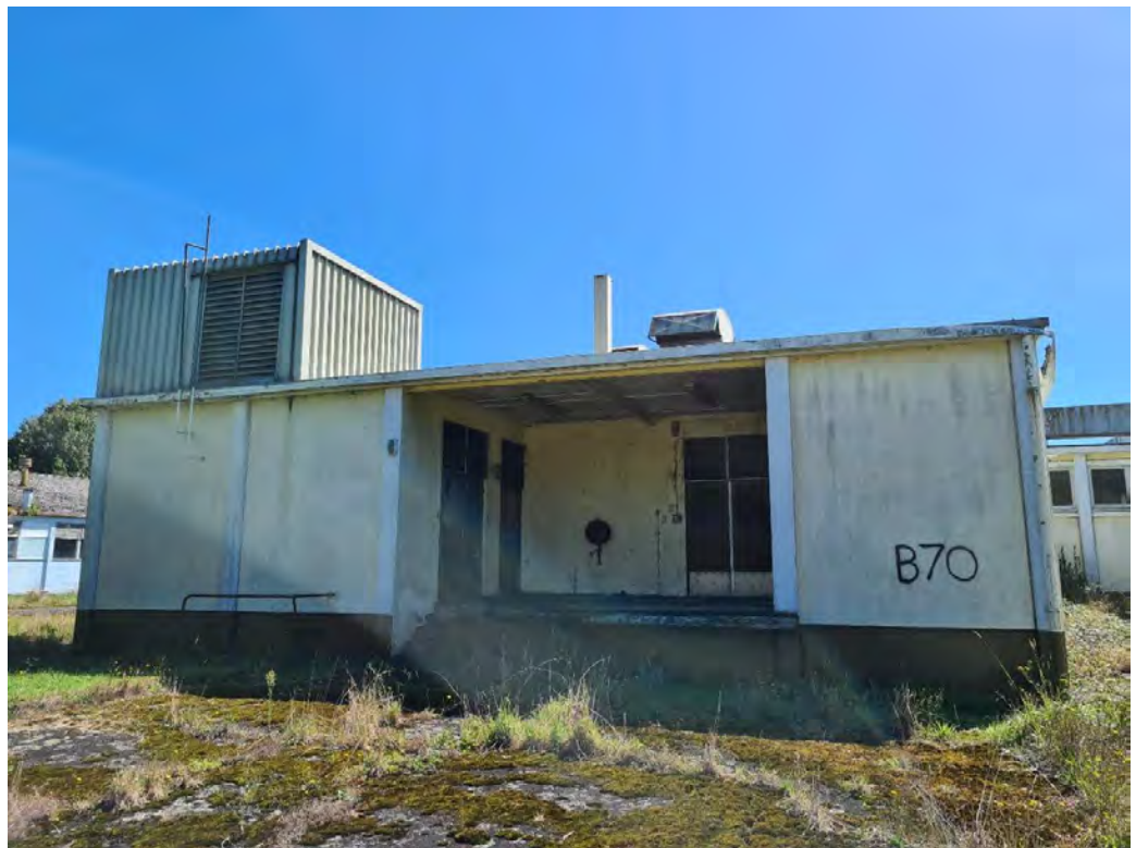
Plate X50: Looking north towards B70.
