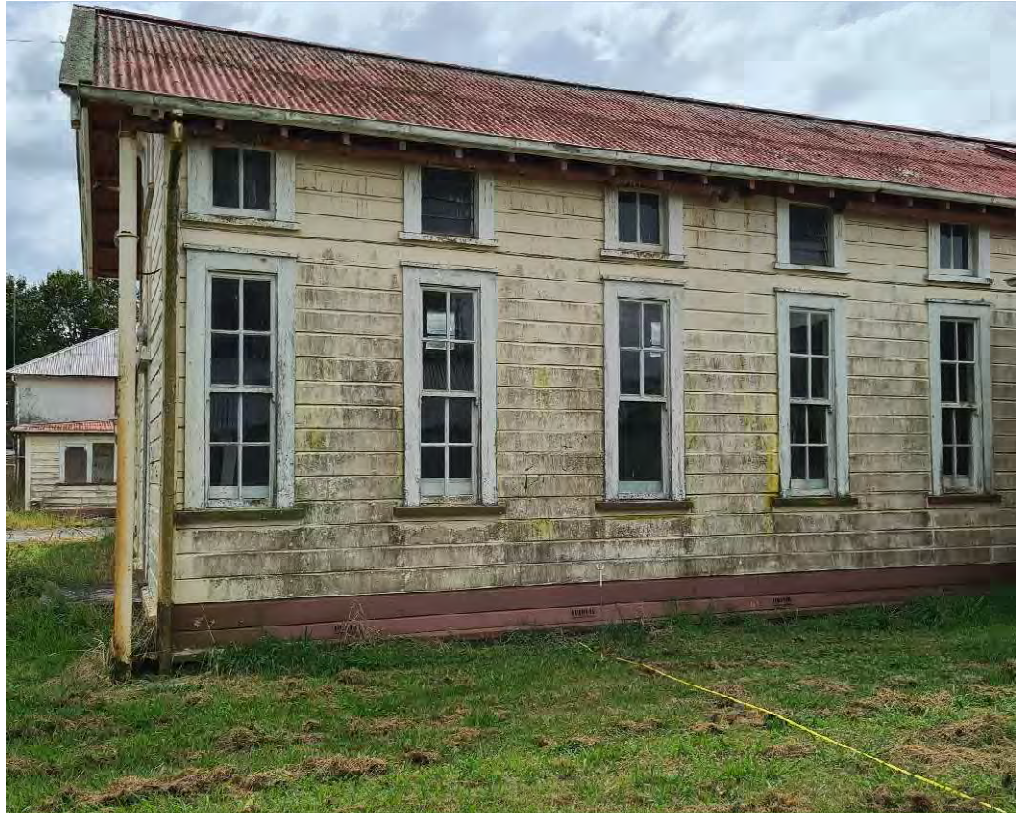
Plate X11: Looking north towards southwest corner of B11.
