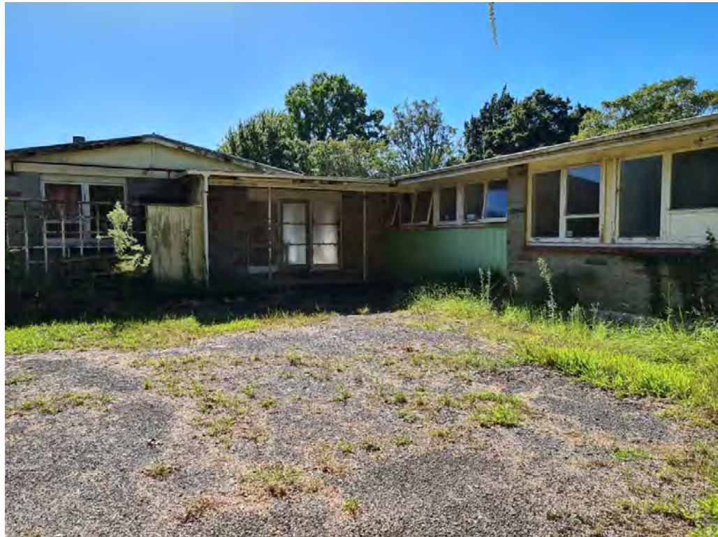
Plate X50: Looking north towards B75.
