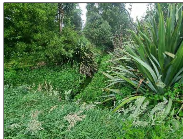
Photo 10: Upstream of Culvert 3.
