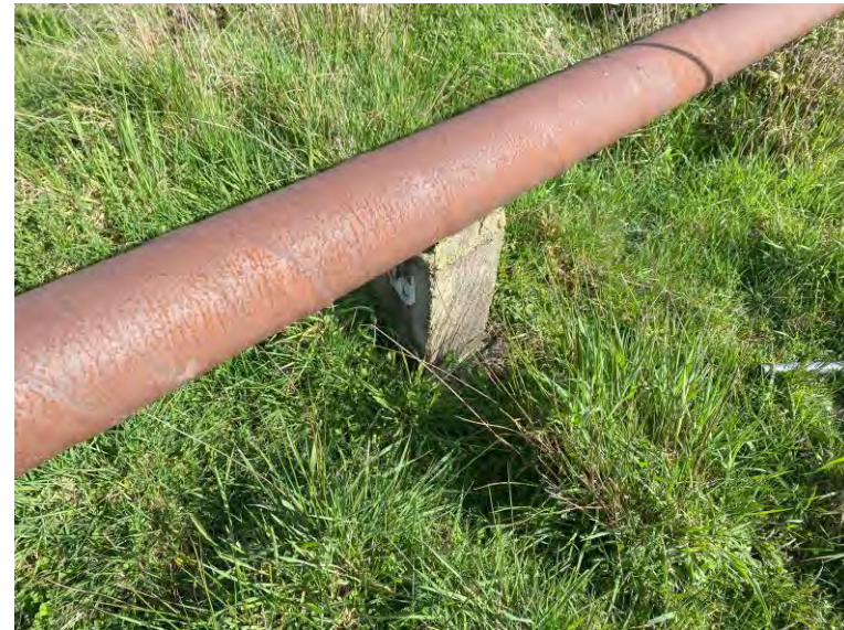
Southern pipeline with concrete pile
