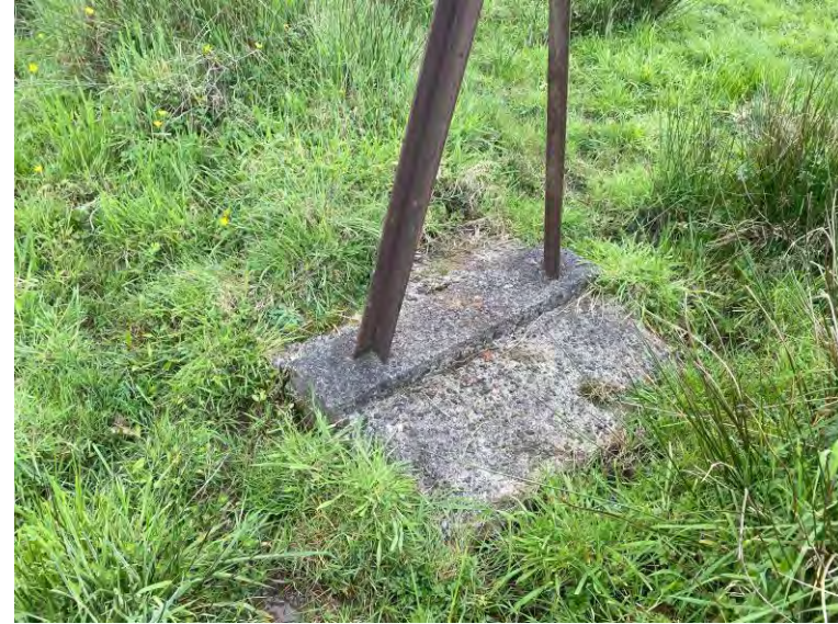
Southern pipeline footings and concrete foundation
