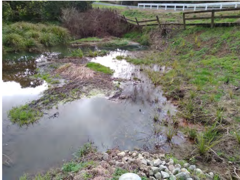
Culvert 1 Inlet – showing signs of bank slumping/ subsidence
