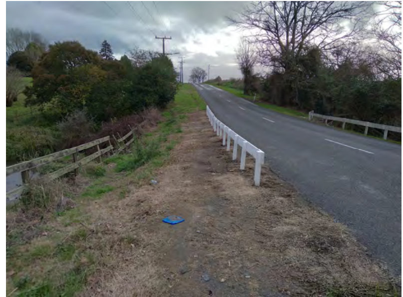
Culvert 1, looking along Te Mawhai Rd
