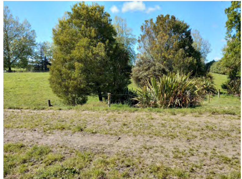
Farm Track @ Culvert 3
