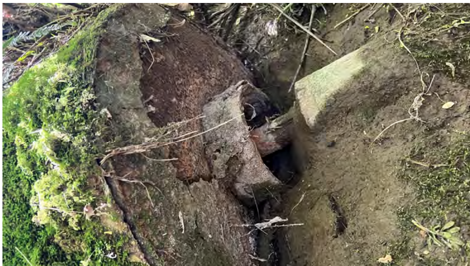
Unidentified feature at western bank - Culvert 3 Outlet
