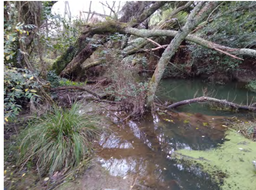
Culvert 1 Outlet, looking further downstream
