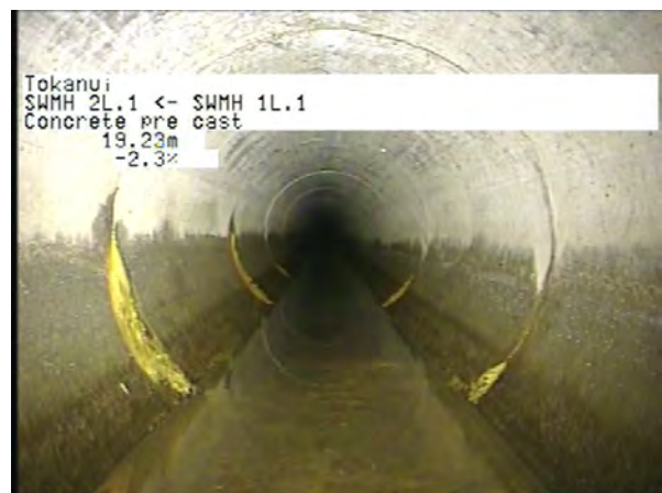
MH 1L.1 To MH 2L.1_f0e82095-1b62-4dac-8fc4-cca58a9d07c5_20230404_12 5904_777.jpg, 00:05:40, 19.23m
