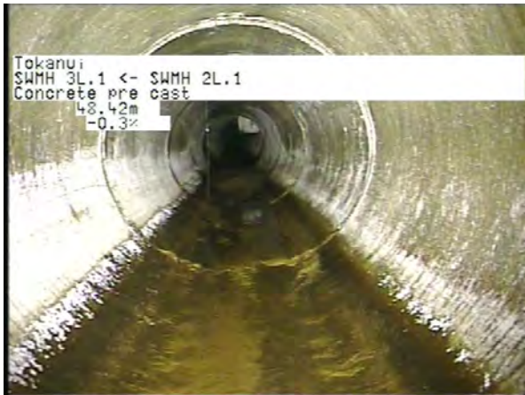
MH 2L.1 To MH 3L.1_e554e0b9-0110-479f-99d1-f1319bec53e9_20230406_12 1327_666.jpg, 00:15:29, 48.42m
