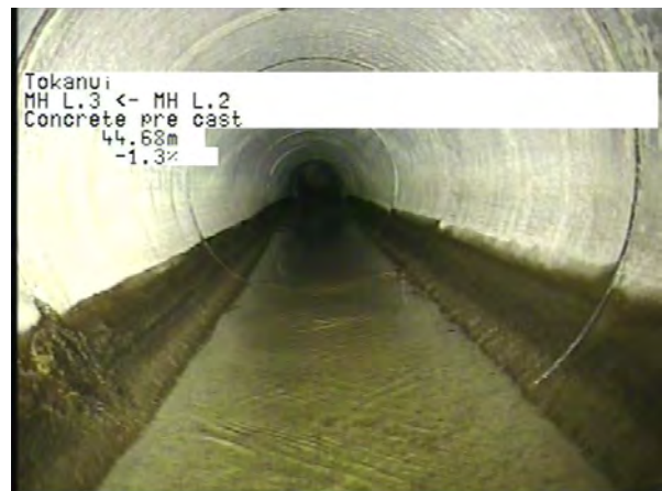
MH L.2 To MH L.3_d4aa0fbd-a310-427e-bb5c-b73b1572e744_20230328_140554_236.jpg, 00:14:00, 44.68m
