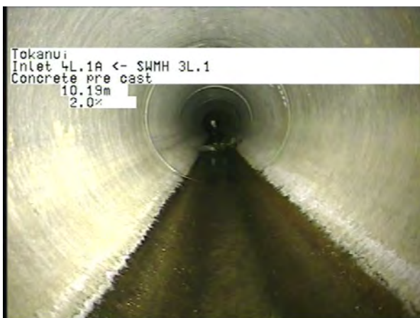
MH 3L.1 To 4L.1A Inlet_27d76b44-1329-4185-a445-6a22b89150e4_20230406_1 42804_766.jpg, 00:03:16, 10.19m
