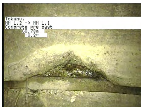
MH L.2 To MH L.1_efb44499-721b-4229-8c4f-42665233aa51_20230328_115 911_584.jpg, 00:18:10, 60.78m
