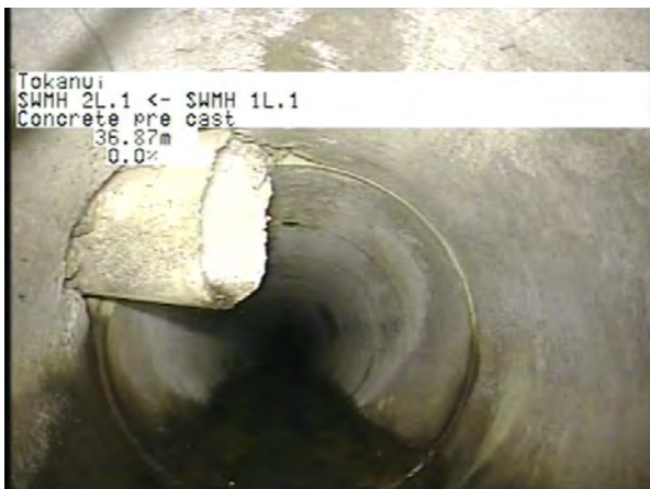
MH 1L.1 To MH 2L.1_c2db88c6-bce0-402e-beac-0c8459e6653a_20230406_1 33236_184.jpg, 00:11:21, 36.87m
