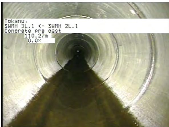
MH 2L.1 To MH 3L.1_8e5a35ef-e81f-4f5f-8d3e-c46288c65d89_20230406_123 319_889.jpg, 00:32:44, 110.27m
