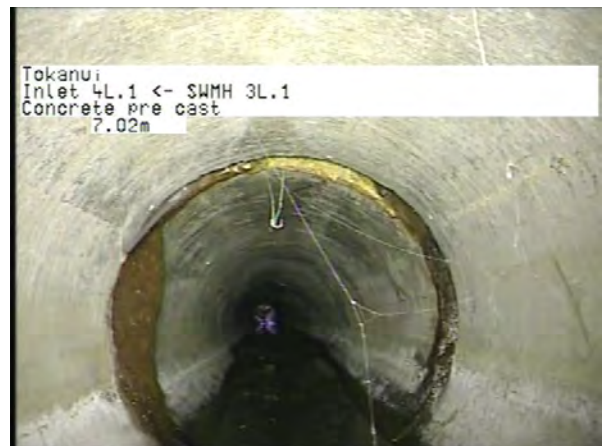
MH 3L.1 To Outlet 4L.1_8a036046-8af3-45b3-84a4-b02f39ee56aa_20230406_12 4659_854.jpg, 00:01:58, 7.02m
