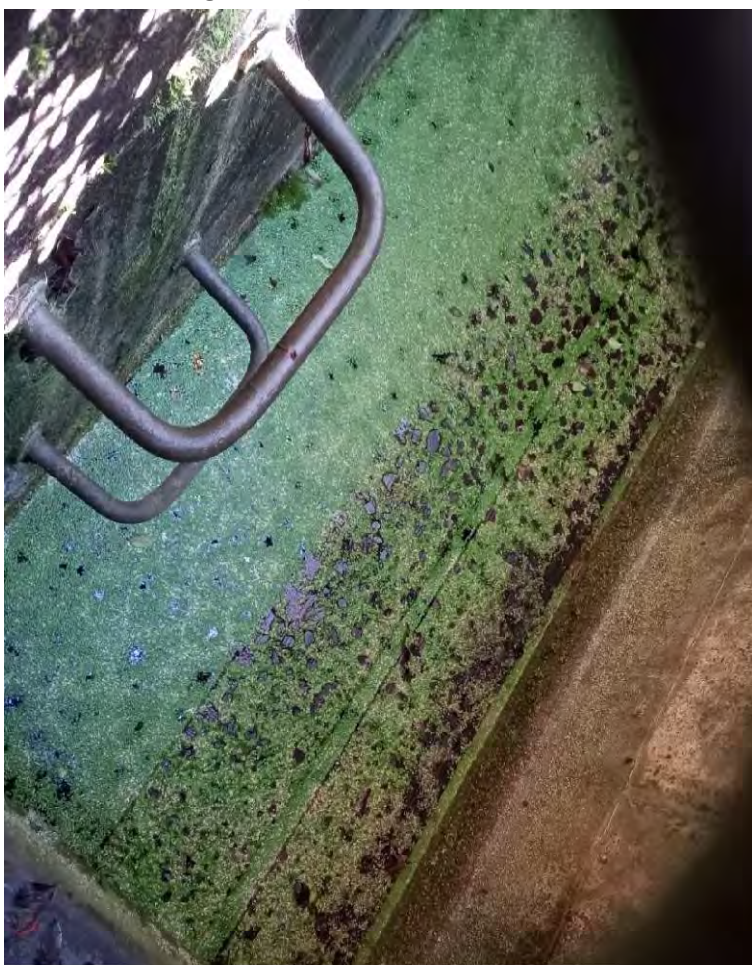
Figure 28: Inside of grit chamber
