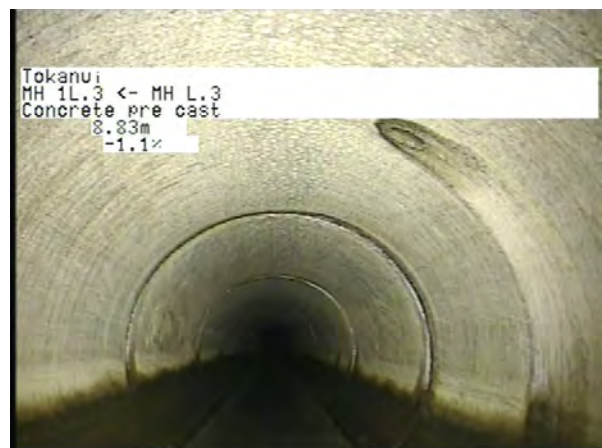
MH L.3 To MH 1L.3_752af1d2-ad7e-493d-9bd1-af300831cc88_20230404_10 3303_226.jpg, 00:04:00, 8.83m
