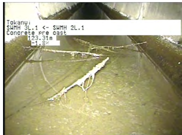
MH 2L.1 To MH 3L.1_94e435f8-c298-4f98-a11a-c86148ee5e35_20230406_12 3602_149.jpg, 00:35:20, 123.31m
