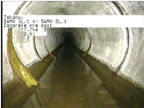
MH 2L.1 To MH 3L.1_25a9d203-42bf-4094-b32a-dc82147c3bdd_20230406_1 20335_143.jpg, 00:06:12, 17.74m
