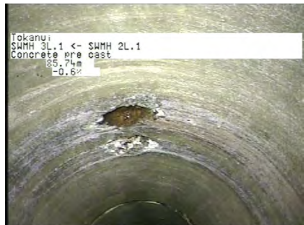
MH 2L.1 To MH 3L.1_72767a2a-11d7-4fb3-a775-4c123d77f17e_20230406_12 2646_970.jpg, 00:26:51, 85.74m
