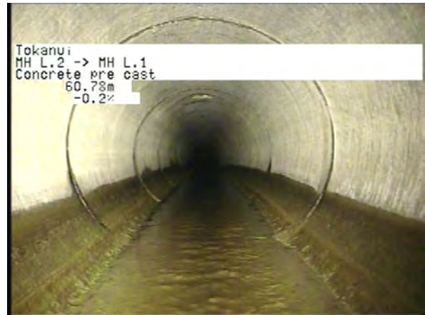
MH L.2 To MH L.1_871192d3-4982-43f0-86ab-6d695a16e812_20230328_120028_336.jpg, 00:18:44, 60.78m
