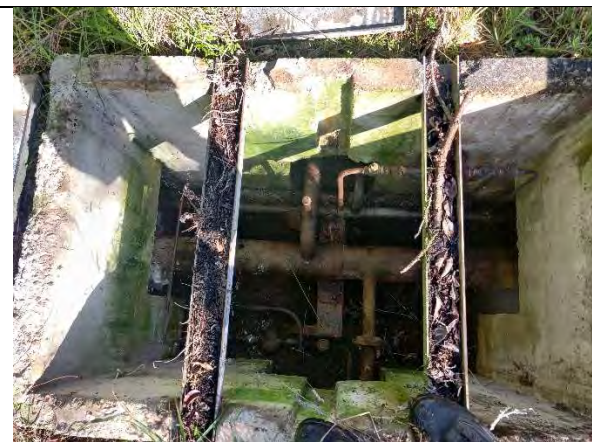
Chamber H08 located at B48 Ward 16
