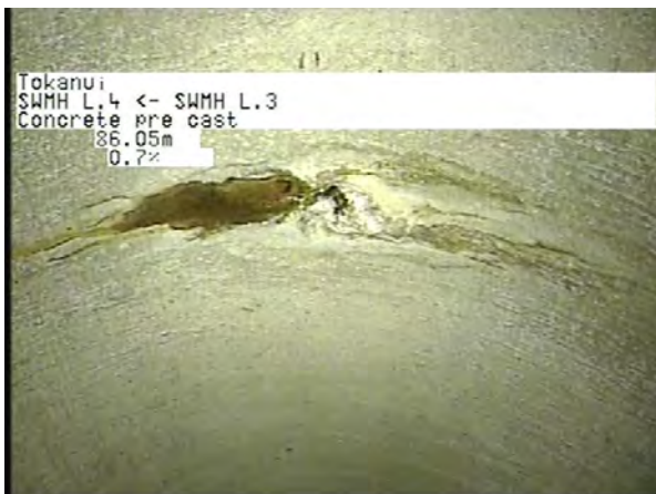
MH L.3 To MH L.4_1145e1e5-58c4-4518-9f96-9c7287b2e87d_20230404_09 5212_284.jpg, 00:20:52, 86.05m
