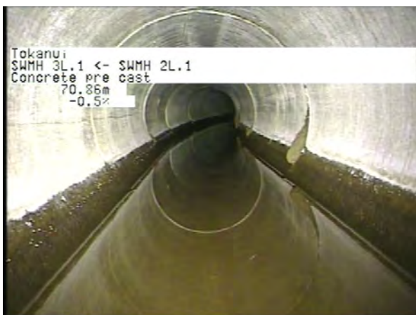
MH 2L.1 To MH 3L.1_136818a2-df21-4a67-ac6d-4a4953e24792_20230406_1 22231_453.jpg, 00:22:57, 70.86m
