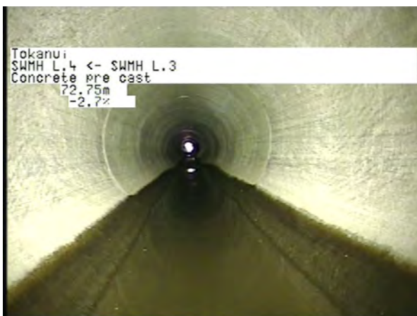
MH L.3 To MH L.4_00c0760c-1fa4-4709-9b65-66771ccc44d4_20230404_094827_863.jpg, 00:18:00, 72.75m
