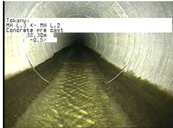
MH L.2 To MH L.3_20816295-8f31-4580-ae7c-6c200e2ecbbd_20230328_140247_469.jpg, 00:11:54, 38.30m
