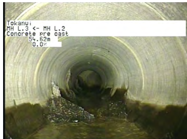
MH L.2 To MH L.3_50faec17-9592-40c3-b72e-967ba7ed3250_20230328_141021_428.jpg, 00:17:18, 54.62m
