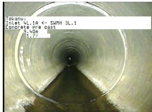
MH 3L.1 To 4L.1A Inlet_47aebede-4187-4981-a74e-e369e4ee9c31_20230406_1 42704_666.jpg, 00:02:26, 9.40m
