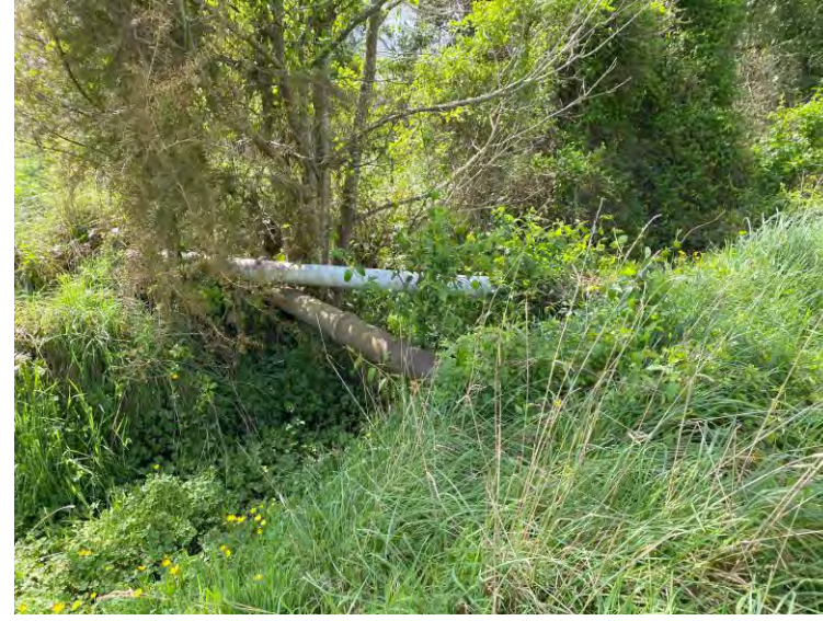
Additional pipeline underlying eastern pipeline
