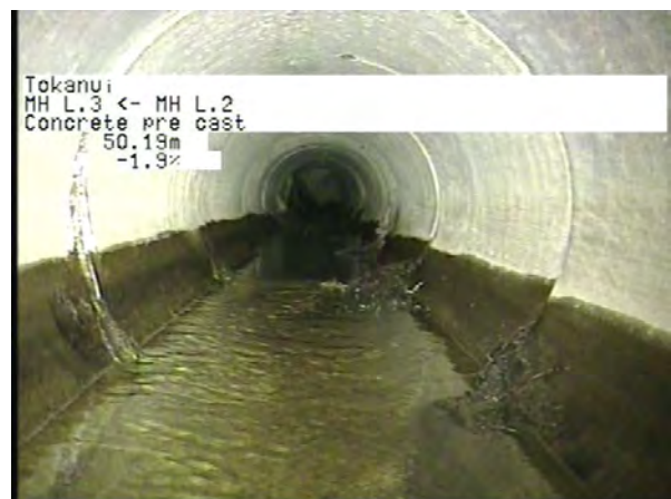
MH L.2 To MH L.3_7a485f99-6caa-477c-ae76-26ec77a4d9a1_20230328_140843_916.jpg, 00:16:16, 50.19m
