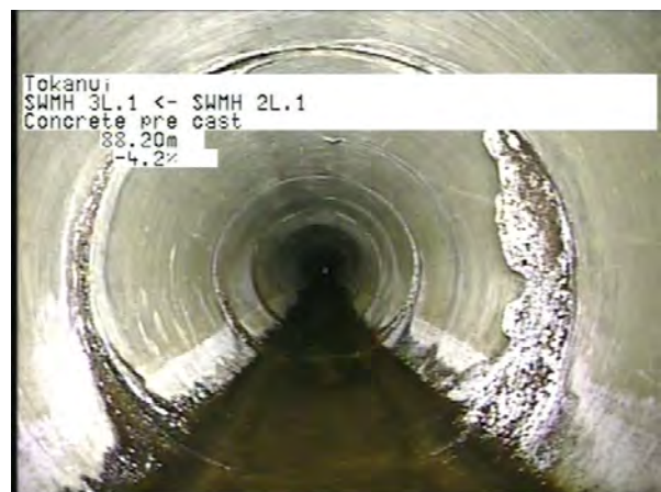
MH 2L.1 To MH 3L.1_bd9683a4-d2d6-45bd-a6f7-64a7ab74fe45_20230406_12 2742_049.jpg, 00:27:30, 88.20m
