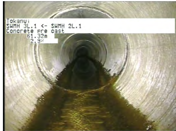
MH 2L.1 To MH 3L.1_0e2c1454-5656-4755-9c20-8dfd7c6bb14f_20230406_12 1910_280.jpg, 00:19:54, 61.32m
