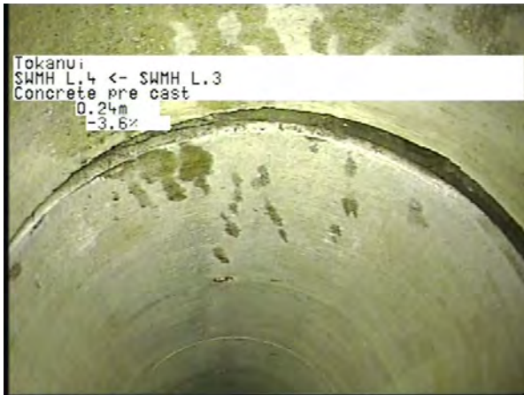
MH L.3 To MH L.4_9483e21f-fbf2-4525-84ac-cde70fca9a8b_20230404_0929 22_705.jpg, 00:01:33, 0.24m
