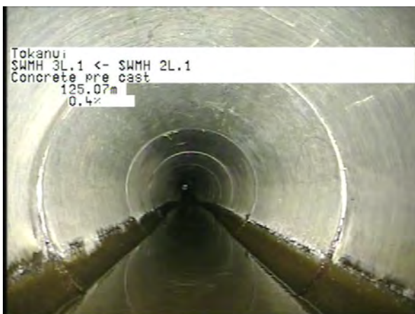
MH 2L.1 To MH 3L.1_b04a8d02-70fb-47fd-ac87-52fbed3a7acc_20230406_12 3636_380.jpg, 00:35:46, 125.07m
