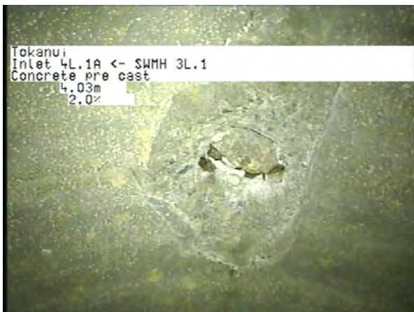
MH 3L.1 To 4L.1A Inlet_996a0ca0-0fb5-4ab1-8c77-3beade6c34b4_20230406_14 2602_793.jpg, 00:01:36, 4.03m
