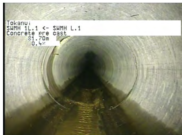
MH L.1 To MH 1L.1_42825bdf-2533-4d78-89c6-f464772da77f_20230404_12 2721_178.jpg, 00:22:41, 81.70m
