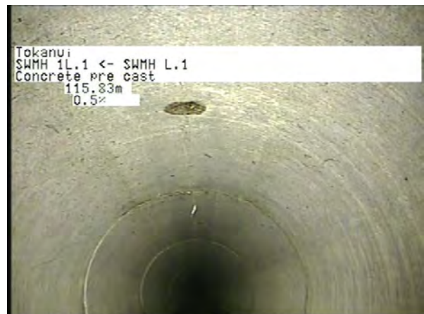
MH L.1 To MH 1L.1_8e9d2cae-b773-40b0-8ab7-475f3d2c9f91_20230404_12 3748_125.jpg, 00:31:23, 115.83m
