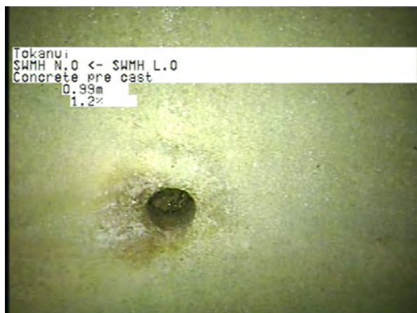
MH L.0 To MH N.O_d86cde5e-42e8-4368-8579-a99ad8755ca5_20230406_15 2537_334.jpg, 00:00:25, 0.99m
