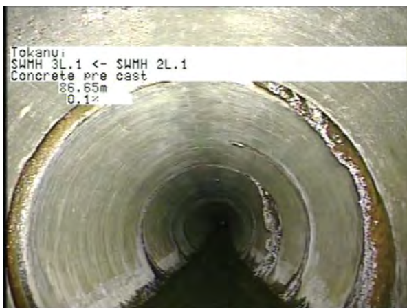
MH 2L.1 To MH 3L.1_8aa14d2c-8d03-4b5a-885b-c75f949e1c53_20230406_1 22710_190.jpg, 00:27:08, 86.65m
