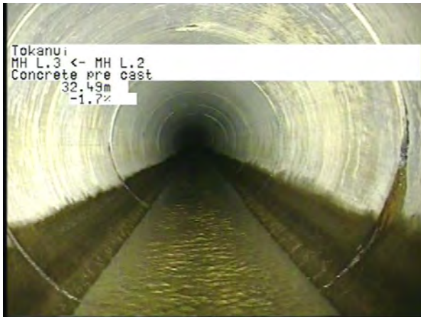
MH L.2 To MH L.3_568339f8-f189-43ca-bc6b-fe03ac71797e_20230328_14056_140.jpg, 00:10:10, 32.49m
