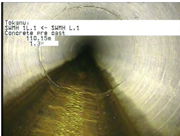
MH L.1 To MH 1L.1_2d00e69a-401a-4f6c-b68f-de18bc68fec6_20230404_12 3625_720.jpg, 00:30:08, 110.15m
