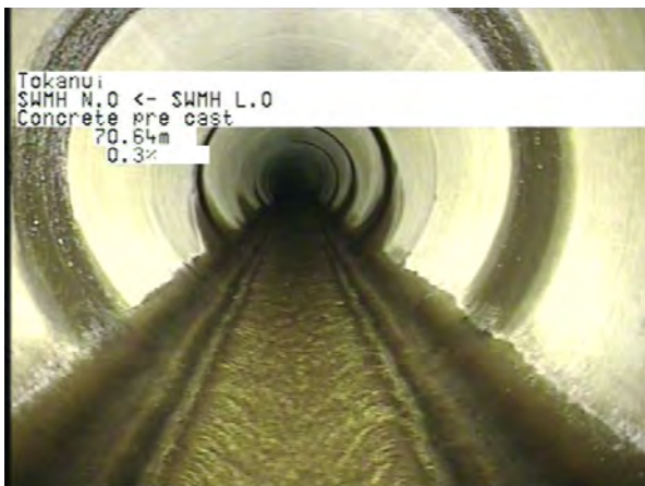
MH L.0 To MH N.0_6219bdfc-dab6-4dde-a1e5-6f34164f0dbe_20230406_153916_073.jpg, 00:12:16, 70.64m
