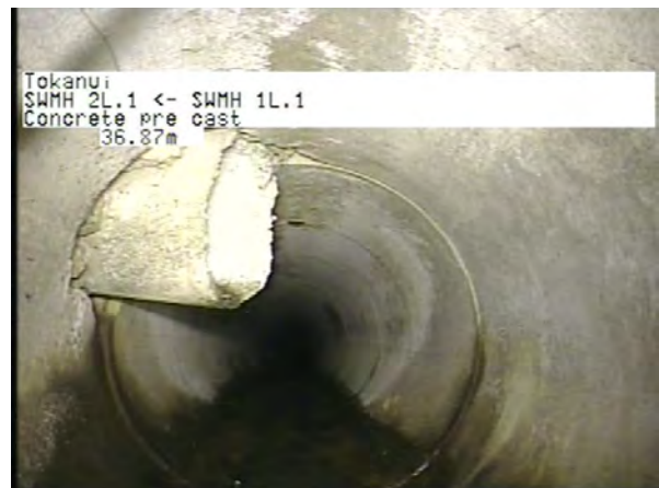
MH 1L.1 To MH 2L.1_fe839006-cb3a-4915-99b0-470c2130e1f0_20230406_13 3247_716.jpg, 00:11:25, 36.87m
