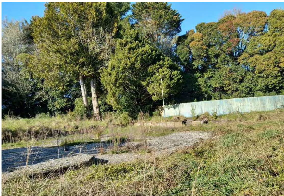
Figure 25: Remove trickling filter (circular tank in background) and stone media (item 7).
