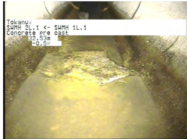
MH 1L.1 To MH 2L.1_9511c068-864d-4c84-9b94-0e42454dbf51_20230406_1 33107_242.jpg, 00:10:04, 32.53m
