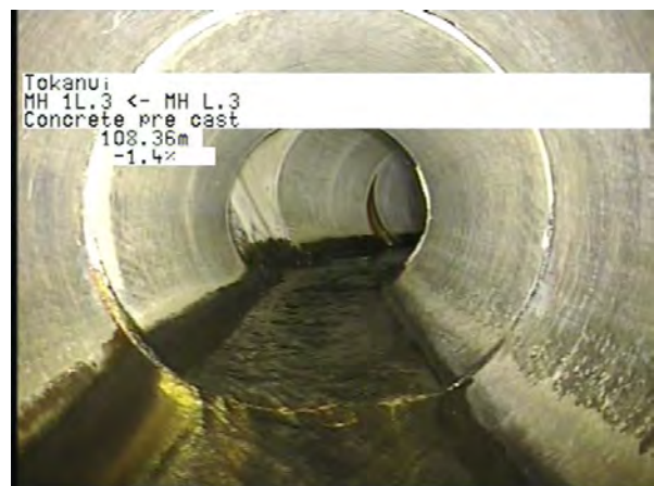
MH L.3 To MH 1L.3_0e402055-9531-471c-a05a-3fd09f339a5d_20230404_11 0136_057.jpg, 00:28:35, 108.36m
