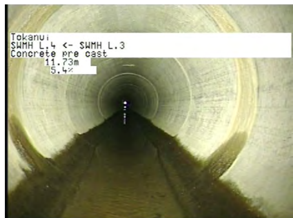
MH L.3 To MH L.4_d6136215-d14d-4474-84f1-c046939e6261_20230404_09 3413_023.jpg, 00:05:15, 11.73m
