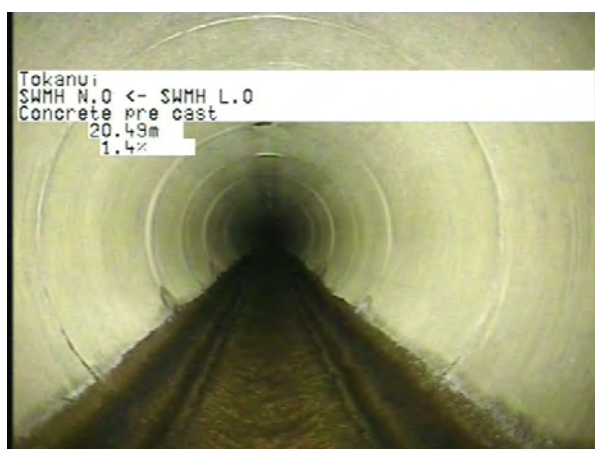
MH L.0 To MH N.O_d65ad6a2-e3ab-4f0f-81eb-6eaac14ceb03_20230406_15 3109_779.jpg, 00:05:17, 20.49m
