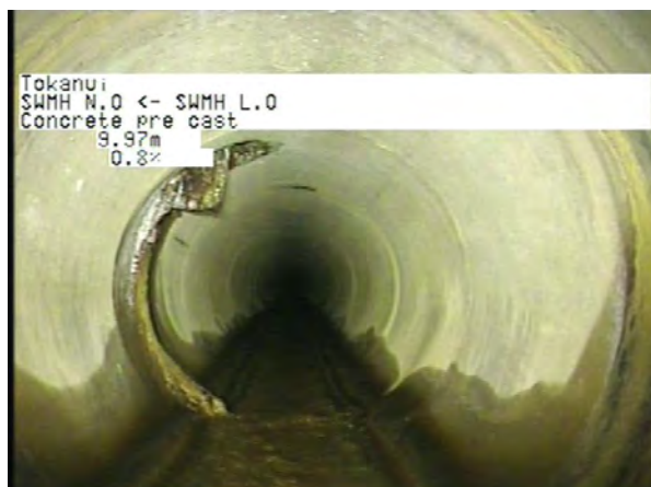
MH L.0 To MH N.O_7dc38427-e264-4876-8582-31f10e6f1f74_20230406_152 828_461.jpg, 00:03:00, 9.97m
