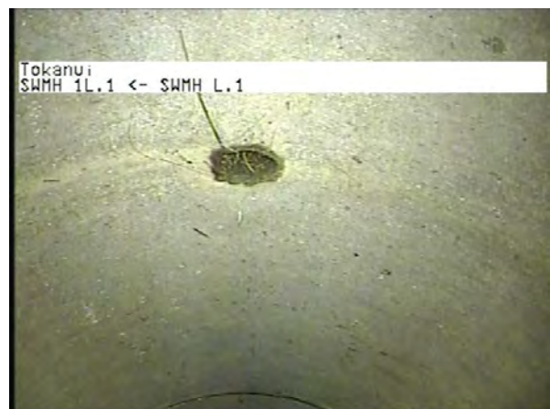
MH L.1 To MH 1L.1_7328faf1-e9fd-4b70-b36d-d89065e11fd0_20230404_120 532_852.jpg, 00:05:09, 13.68m
