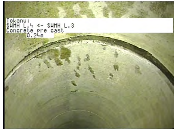
MH L.3 To MH L.4_acd751df-e779-47b3-9dc6-eb01e40c7129_20230404_09 2932_514.jpg, 00:01:35, 0.24m
