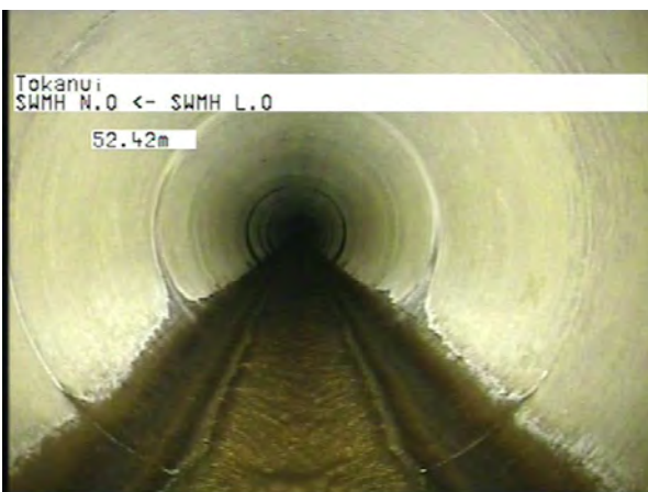
MH L.0 To MH N.0_beed4716-67b9-4cb7-8f97-55b4515aa116_20230406_15 3547_675.jpg, 00:09:23, 52.42m
