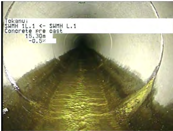
MH L.1 To MH 1L.1_ddeb10f3-b577-4669-8edd-7efe4b96e1f7_20230404_12 0653_052.jpg, 00:06:21, 15.30m
