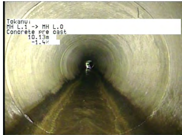
MH L.1 To MH L.O_fbfb21c-d50d-4f33-9bf1-b65d759c40e9_20230328_1220 48_867.jpg, 00:02:39, 10.13m
