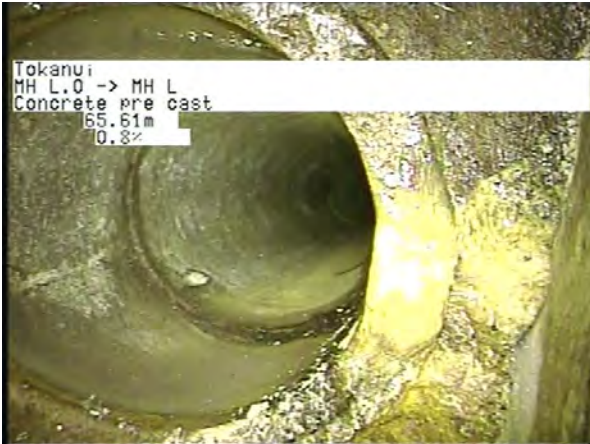
MH L.0 To MH L_1ab9717d-4439-4e6c-a20a-3a59d6fb6d44_20230328_124355_554.jpg, 00:14:59, 65.61m
