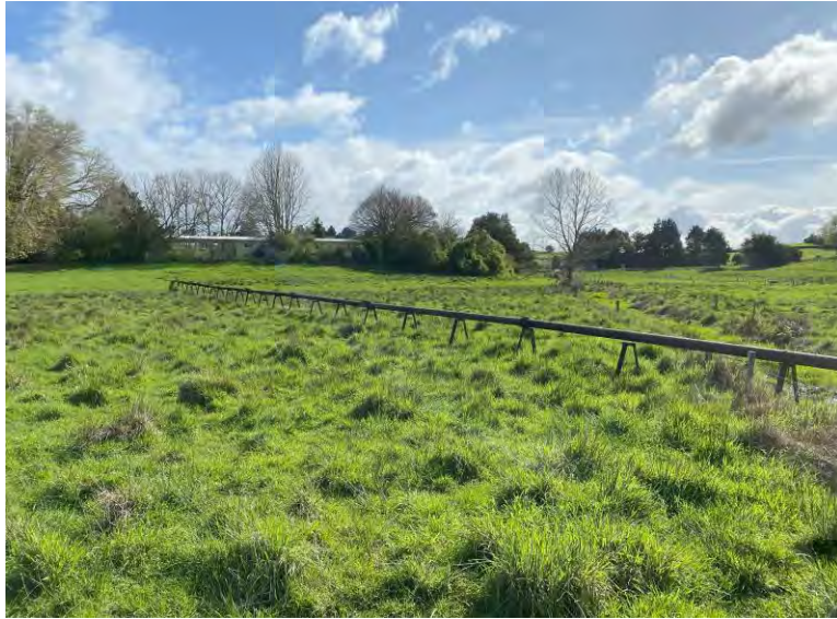
Southern pipeline with footings
