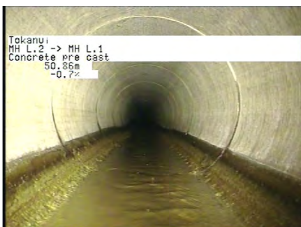
MH L.2 To MH L.1_5c75dd65-c56b-47f9-96e8-593603864276_20230328_11 5552_877.jpg, 00:15:01, 50.86m
