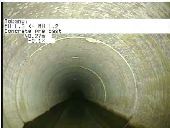
MH L.2 To MH L.3_64599a16-9a20-4a6e-8d0f-d6710a681735_20230328_140454_459.jpg, 00:13:08, 40.27m
