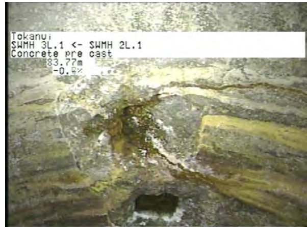
MH 2L.1 To MH 3L.1_3158cbc6-51db-4f0b-a441-ad166bbff3c_20230406_122 533_243.jpg, 00:25:35, 83.19m
