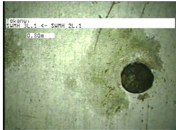
MH 2L.1 To MH 3L.1_f3e577a9-28ba-4560-b89e-0da46a5d7ccd_20230406_1 15700_124.jpg, 00:00:19, 0.80m
