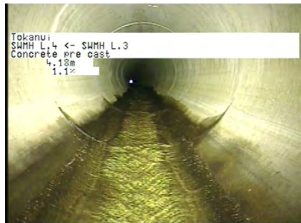
MH L.3 To MH L.4_95ba27fa-0b01-46ac-bbcb-ec2fe721d773_20230404_093 219_100.jpg, 00:03:51, 4.33m
