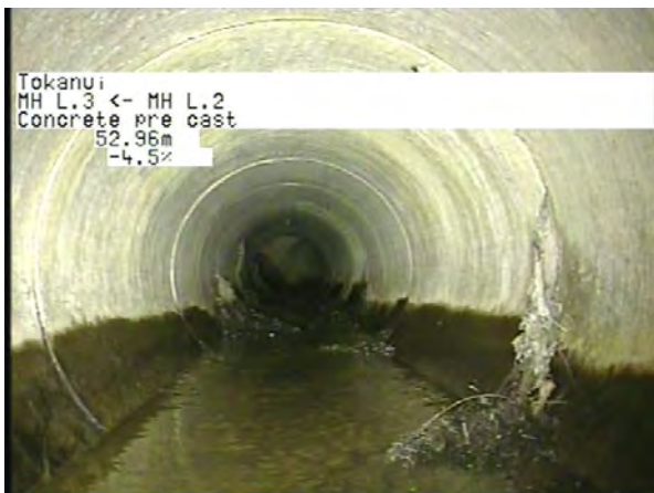
MH L.2 To MH L.3_29f251b6-5a99-48cb-8bd7-bfa904795369_20230328_140942_137.jpg, 00:16:55, 52.96m
