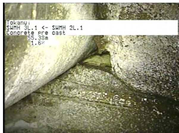
MH 2L.1 To MH 3L.1_f2f34aca-72da-436c-a029-ee3f67361e9f_20230406_121 642_298.jpg, 00:17:39, 55.38m
