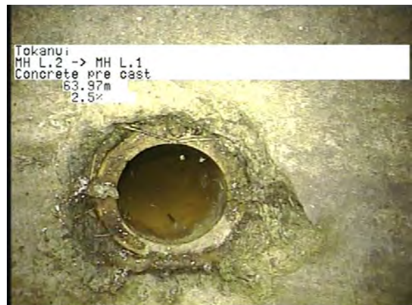
MH L.2 To MH L.1_68bb6ee9-5d17-4b5a-9c18-8d08dc184668_20230328_120226_030.jpg, 00:20:10, 62.90m
