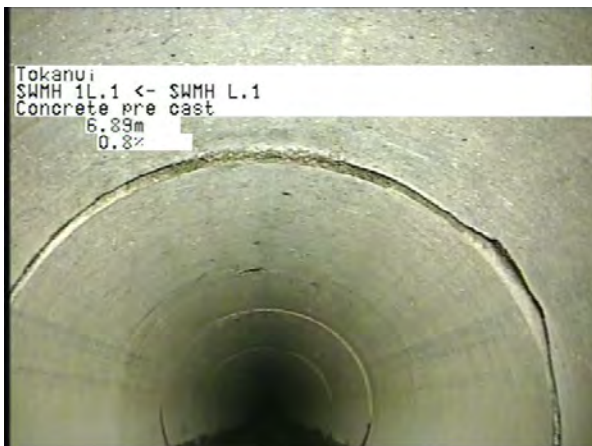
MH L.1 To MH 1L.1_d7ddc1f8-ff6b-4066-9a3e-e9ac1c07d5db_20230404_12 0247_678.jpg, 00:02:55, 6.89m
