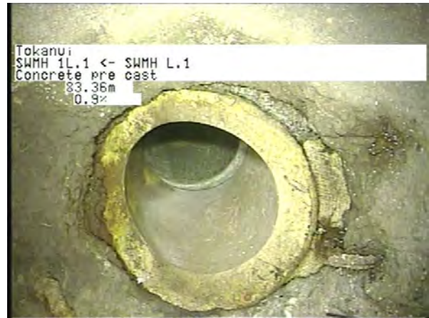
MH L.1 To MH 1L.1_8c992c4c-160a-43ed-8d8e-4f000d7d3860_20230404_1 22808_826.jpg, 00:23:11, 83.36m
