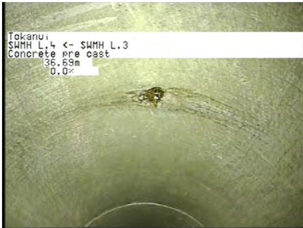
MH L.3 To MH L.4_63eaba63-f480-494e-adec-0f2d2e46468f_20230404_094020_895.jpg, 00:10:29, 36.69m
