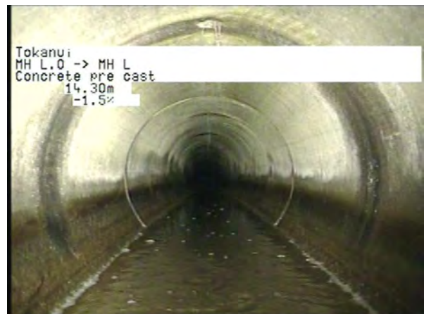
MH L.0 To MH L_194c1efd-790c-4c0f-ac9c-e8a3ff83501b_20230328_123141_927.jpg, 00:04:28, 14.32m
