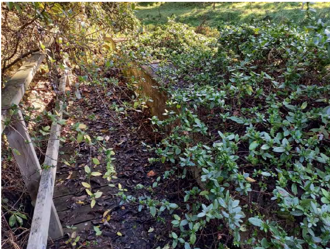
Figure 27: Closeup of grit chamber showing concrete blockwork construction and grated metal lid (largely hidden under vegetation)
