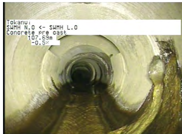
MH L.0 To MH N.O_06c0ac44-61fe-4108-831f-b021c789ebf6_20230406_154 615_108.jpg, 00:17:47, 107.69m
