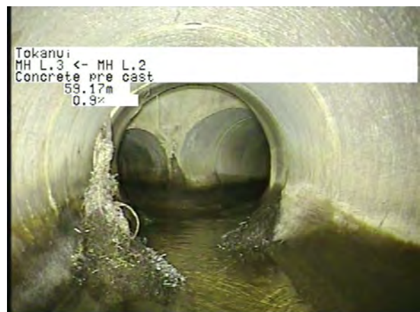
MH L.2 To MH L.3_8bfc9669-19e9-44fe-be56-2918c2d705ac_20230328_141218_604.jpg, 00:18:46, 59.17m
