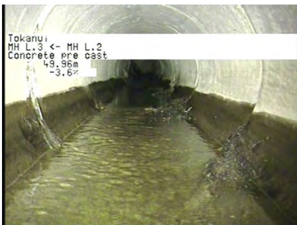
MH L.2 To MH L.3_e372af21-6ca6-4a1f-ac4a-0894e8a8c844_20230328_140718_267.jpg, 00:15:12, 49.96m
