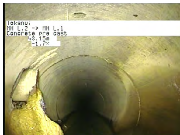
MH L.2 To MH L.1_2b036aa8-bd7c-4b10-ac49-301e16fa4047_20230328_11 5220_452.jpg, 00:12:53, 48.15m
