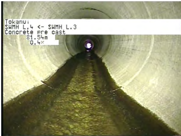
MH L.3 To MH L.4_104e6884-0071-49e3-9eb9-a2205b0c45ce_20230404_09 5100_027.jpg, 00:20:03, 81.54m
