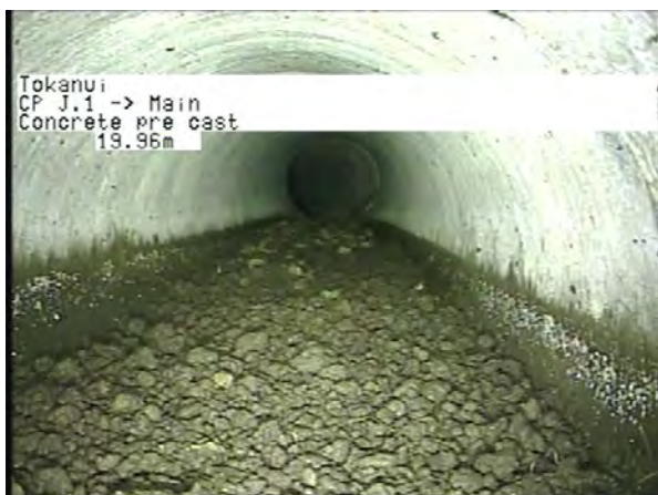
CP J.1 To Main_2371c38a-bcb7-4626-a41b-950699dc0b05_20230327_1 30504_662.jpg, 00:07:18, 19.96m
