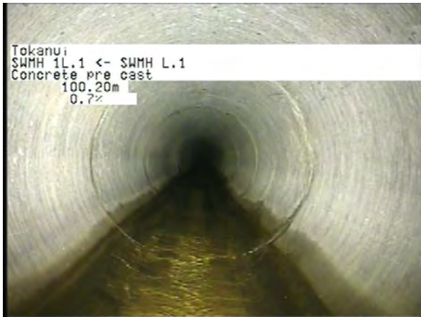
MH L.1 To MH 1L.1_1d7f7522-ff45-4bc8-8e34-c083bc55e52d_20230404_12 3338_682.jpg, 00:27:40, 100.20m
