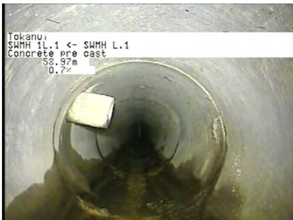
MH L.1 To MH 1L.1_35d0d170-0f81-4417-84fc-51ead01dbb7a_20230404_12 1828_648.jpg, 00:16:02, 58.97m
