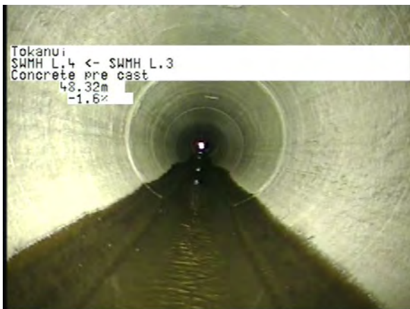
MH L.3 To MH L.4_f287f16f-eca9-47be-a283-cfe61ffd1641_20230404_094323_061.jpg, 00:13:15, 48.32m
