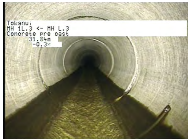
MH L.3 To MH 1L.3_3f0952e8-055a-47f2-98e7-9af1672a533b_20230404_10 4050_803.jpg, 00:10:19, 31.84m
