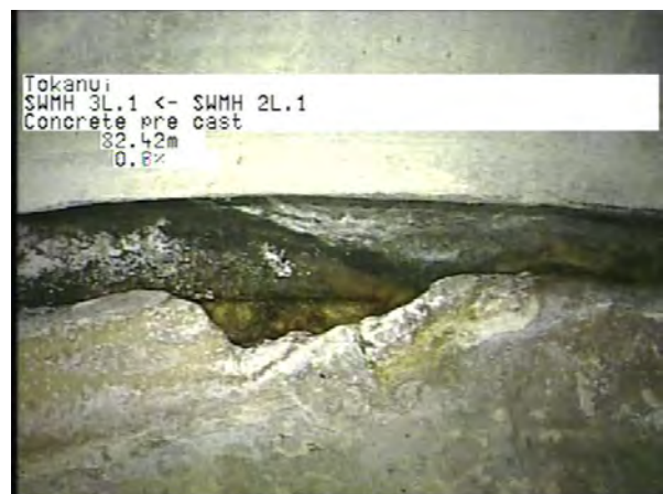
MH 2L.1 To MH 3L.1_076b8fb5-4238-4183-b4a1-5861ccafb161_20230406_12 2456_980.jpg, 00:25:16, 82.42m
