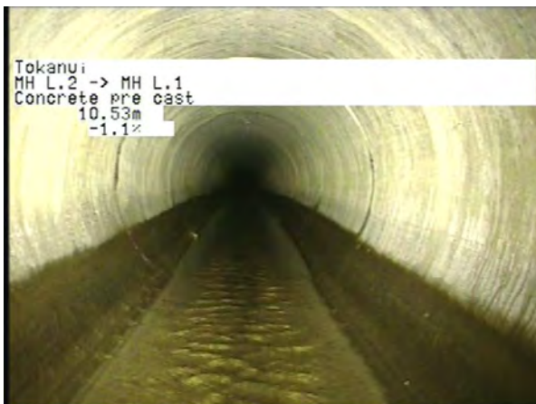
MH L.2 To MH L.1_5de9122a-2035-4069-bf26-f079979d5ad5_20230328_114157_754.jpg, 00:03:55, 10.53m
