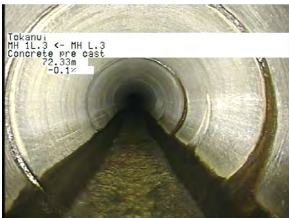
MH L.3 To MH 1L.3_a86f57e8-f424-4cfb-9c0b-d81d8fead7d5_20230404_105 058_071.jpg, 00:19:20, 72.33m
