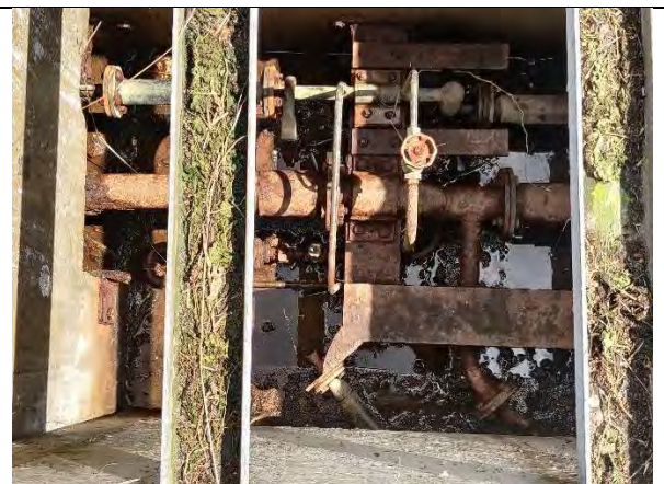
Chamber 925 located at B29 Ward 7
