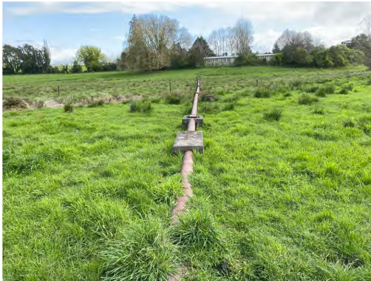
Southern pipeline with concrete casing
