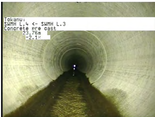
MH L.3 To MH L.4_da1d5de0-ffa4-4fbd-9279-2b5495244872_20230404_093 709_030.jpg, 00:07:46, 23.76m
