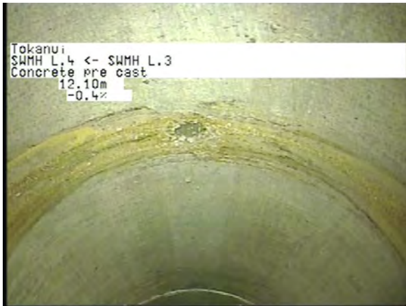
MH L.3 To MH L.4_4eba152a-e6ac-4849-9cd8-310ac2841de4_20230404_09 3436_287.jpg, 00:05:26, 12.10m
