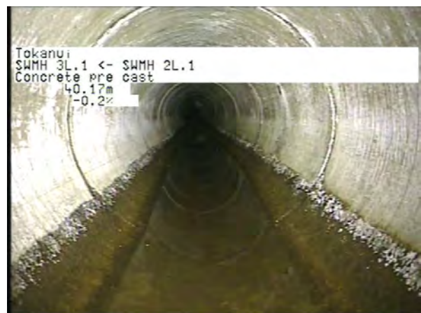
MH 2L.1 To MH 3L.1_ca357b35-9e6c-4f01-9f87-4f16c5b942b2_20230406_12 1137_810.jpg, 00:13:47, 40.17m
