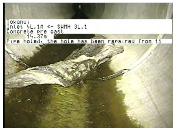
MH 3L.1 To 4L.1A Inlet_0a5fc193-8175-4f24-b7fc-62fa2161c2dc_20230406_142 911_003.jpg, 00:03:51, 14.37m
