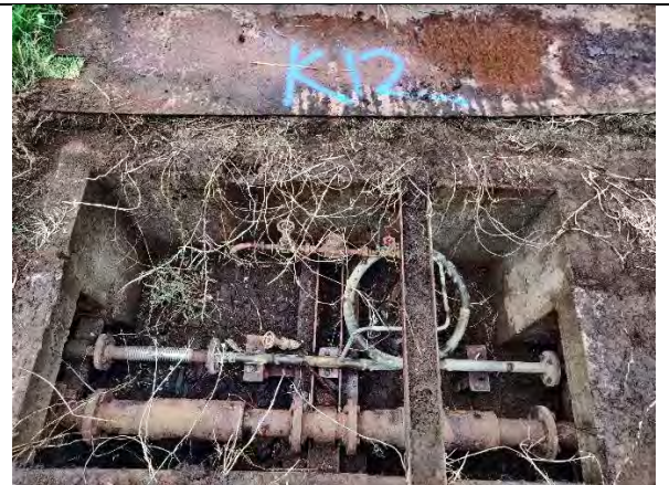
Chamber K12 Located NW of the site
