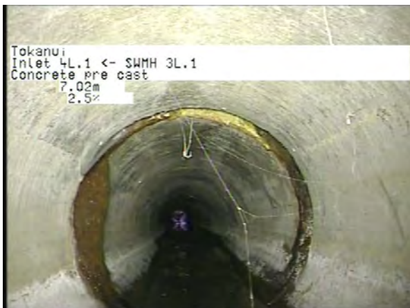
MH 3L.1 To Outlet 4L.1_e4161afd-e948-44e2-a649-42ff507c516a_20230406_12 4650_316.jpg, 00:01:54, 7.02m
