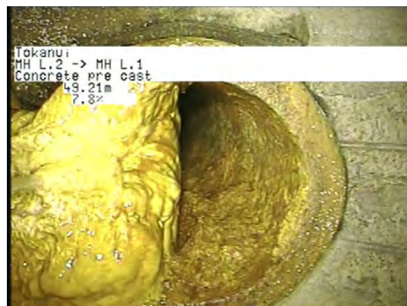
MH L.2 To MH L.1_f1743155-69ae-4a14-957b-195c700051c6_20230328_11 5338_028.jpg, 00:13:47, 49.21m
