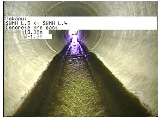
MH L.4 To MH L.5_c014e1cd-ee90-404a-9d96-e6b505e72d05_20230404_095955_739.jpg, 00:02:30, 10.36m
