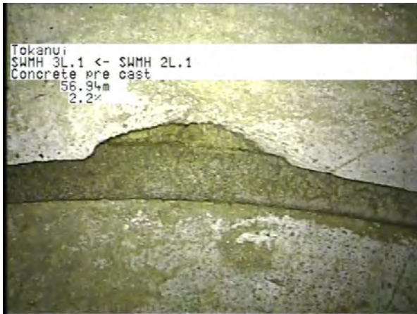
MH 2L.1 To MH 3L.1_61a6279a-f437-4444-93b9-dfccaec0b7e_20230406_12 1716_659.jpg, 00:18:08, 56.94m
