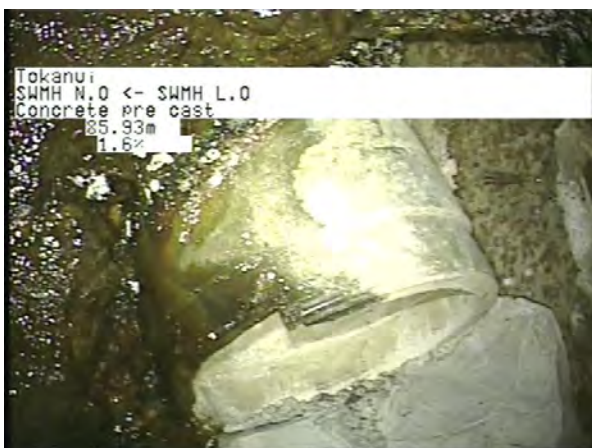
MH L.0 To MH N.0_e4918654-d695-4254-a153-06d53a8b685d_20230406_154149_638.jpg, 00:14:26, 85.93m
