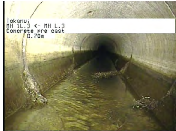
MH L.3 To MH 1L.3_69bcc7ab-8059-4ba9-80e0-7c9783bc7058_20230404_1 02846_035.jpg, 00:00:26, 0.70m
