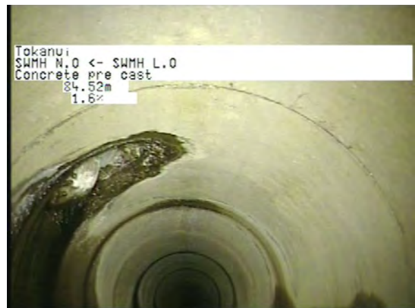
MH L.0 To MH N.0_c8ce0c33-58b0-487e-8ed6-a217ba6b1107_20230406_154114_388.jpg, 00:14:06, 84.52m
