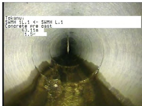
MH L.1 To MH 1L.1_217acfb7-81a1-48f4-9c33-f982301366d5_20230404_12 2102_027.jpg, 00:17:54, 63.11m
