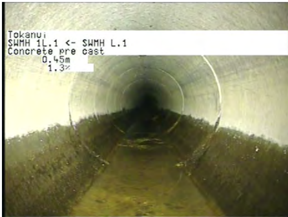
MH L.1 To MH 1L.1_a891dc14-e186-4d51-89eb-a05aef7b844c_20230404_1 20032_471.jpg, 00:01:06, 0.45m
