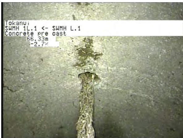
MH L.1 To MH 1L.1_418a2c01-9d84-4963-b087-1e3aebd9728b_20230404_1 22238_777.jpg, 00:18:41, 66.33m
