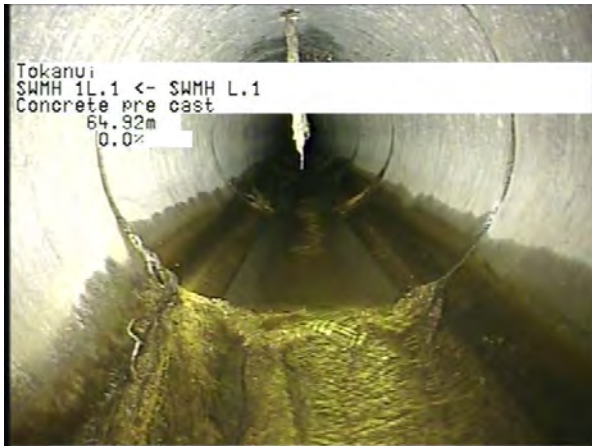
MH L.1 To MH 1L.1_e72c306c-649a-4164-91a8-1ecba2a48658_20230404_1 22145_992.jpg, 00:18:12, 64.92m
