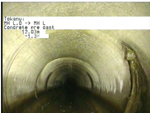
MH L.0 To MH L_f12a7810-30b6-4208-aef4-d6ce680feeb_20230328_123056_656.jpg, 00:03:51, 12.03m
