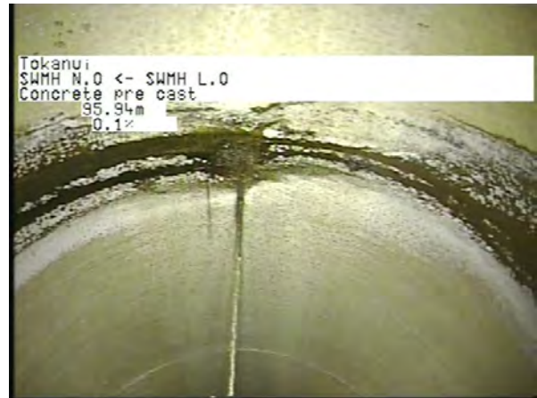
MH L.0 To MH N.O_5621bd13-0c32-42b2-a720-e078e0422212_20230406_1 54407_660.jpg, 00:16:14, 95.94m
