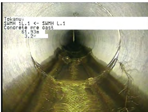
MH L.1 To MH 1L.1_3fb91a5d-147c-4c91-8f09-84a6609702d5_20230404_12 1955_441.jpg, 00:16:58, 61.93m
