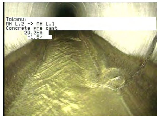
MH L.2 To MH L.1_16023d8f-7f34-4f61-87cd-a060305a2e5e_20230328_114430_558.jpg, 00:06:14, 20.26m
