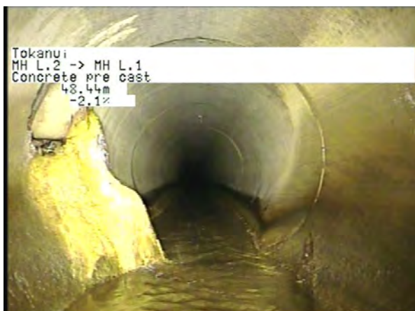
MH L.2 To MH L.1_d89c90f5-4912-4b08-a357-afea7510f596_20230328_115 456_292.jpg, 00:14:12, 48.44m
