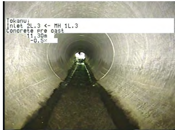
MH 1L.3 To Inlet 2L.3_8195242b-7ad1-4342-80fa-8380f7f9a542_20230404_11 0837_830.jpg, 00:03:00, 11.30m
