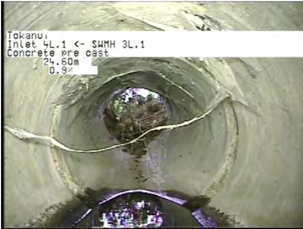
MH 3L.1 To Outlet 4L.1_11e4b69d-76b0-48b6-869b-82ee541d92a4_20230406_1 25256_863.jpg, 00:07:33, 24.60m
