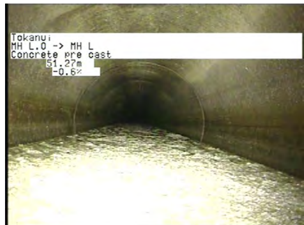
MH L.0 To MH L_8597e2b6-2e19-4c18-8e50-f8c2c716f355_20230328_124035_665.jpg, 00:12:19, 51.27m
