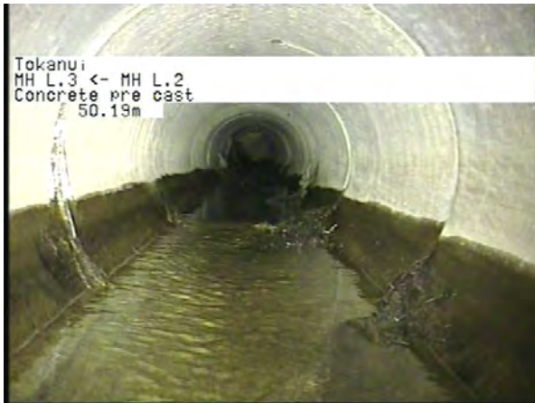
MH L.2 To MH L.3_a277394f-7fb6-450e-b345-6d2dd3481bd6_20230328_140854_849.jpg, 00:16:18, 50.19m
