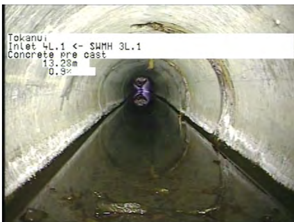
MH 3L.1 To Outlet 4L.1_034cb46f-8662-41f2-97a4-684fef888fe2_20230406_124 921_082.jpg, 00:04:12, 13.28m
