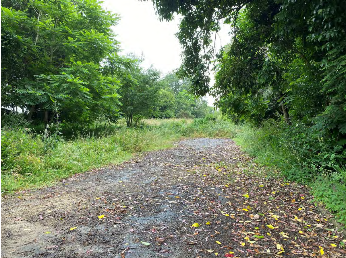
Figure 21: Site Photo of existing roading on site
