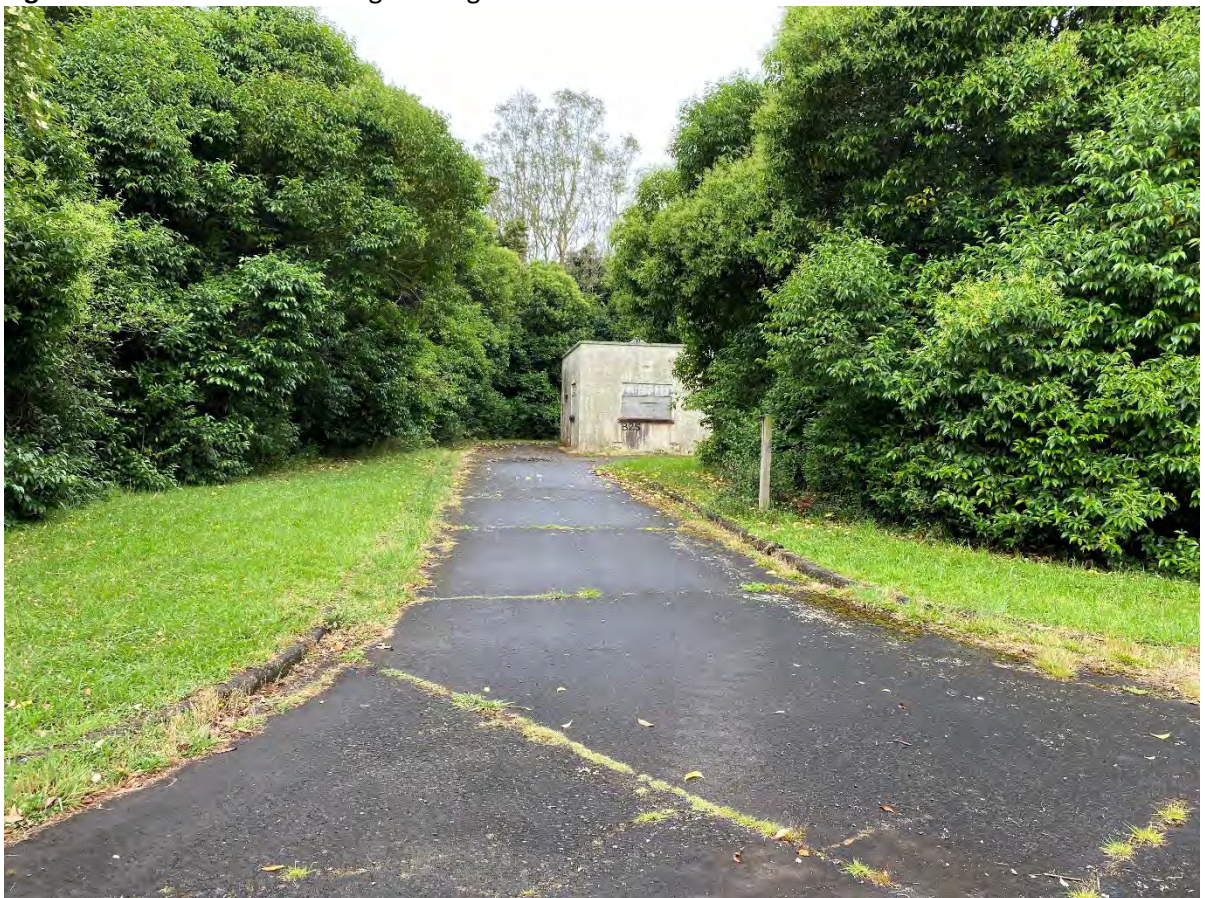
Figure 18: Site Photo of existing roading on site
