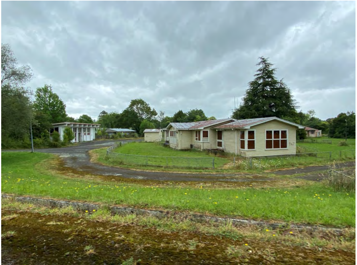
Figure 10: Site Photo of Existing Building on site
