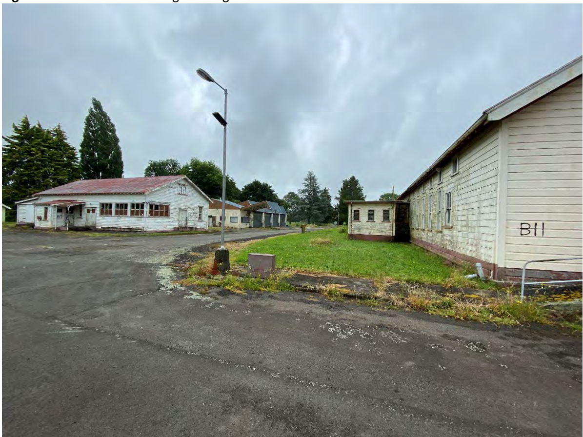
Figure 6: Site Photo of Existing Building on site
