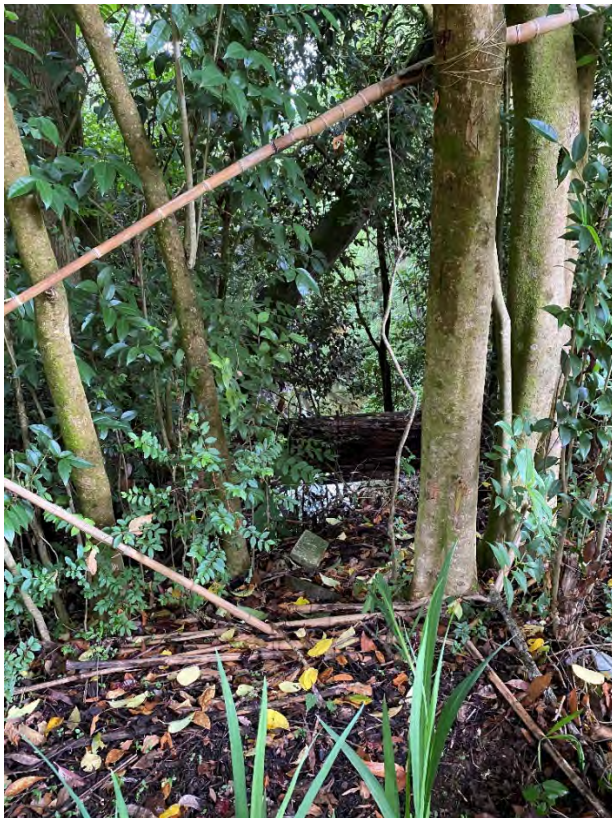
Figure 22: Site Photo looking towards Culvert 2
