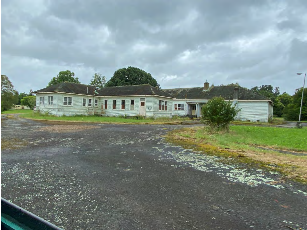
Figure 9: Site Photo of Existing Building on site
