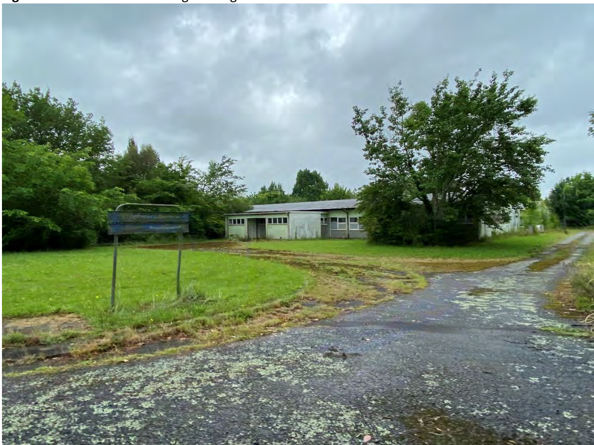
Figure 20: Site Photo of existing roading, including road signage, on site
