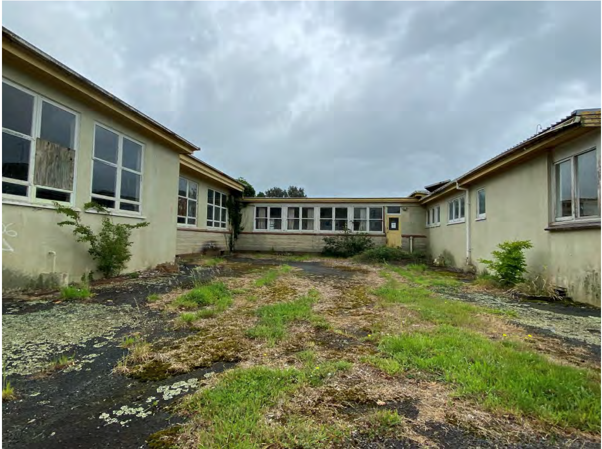
Figure 15: Site Photo of existing building on site
