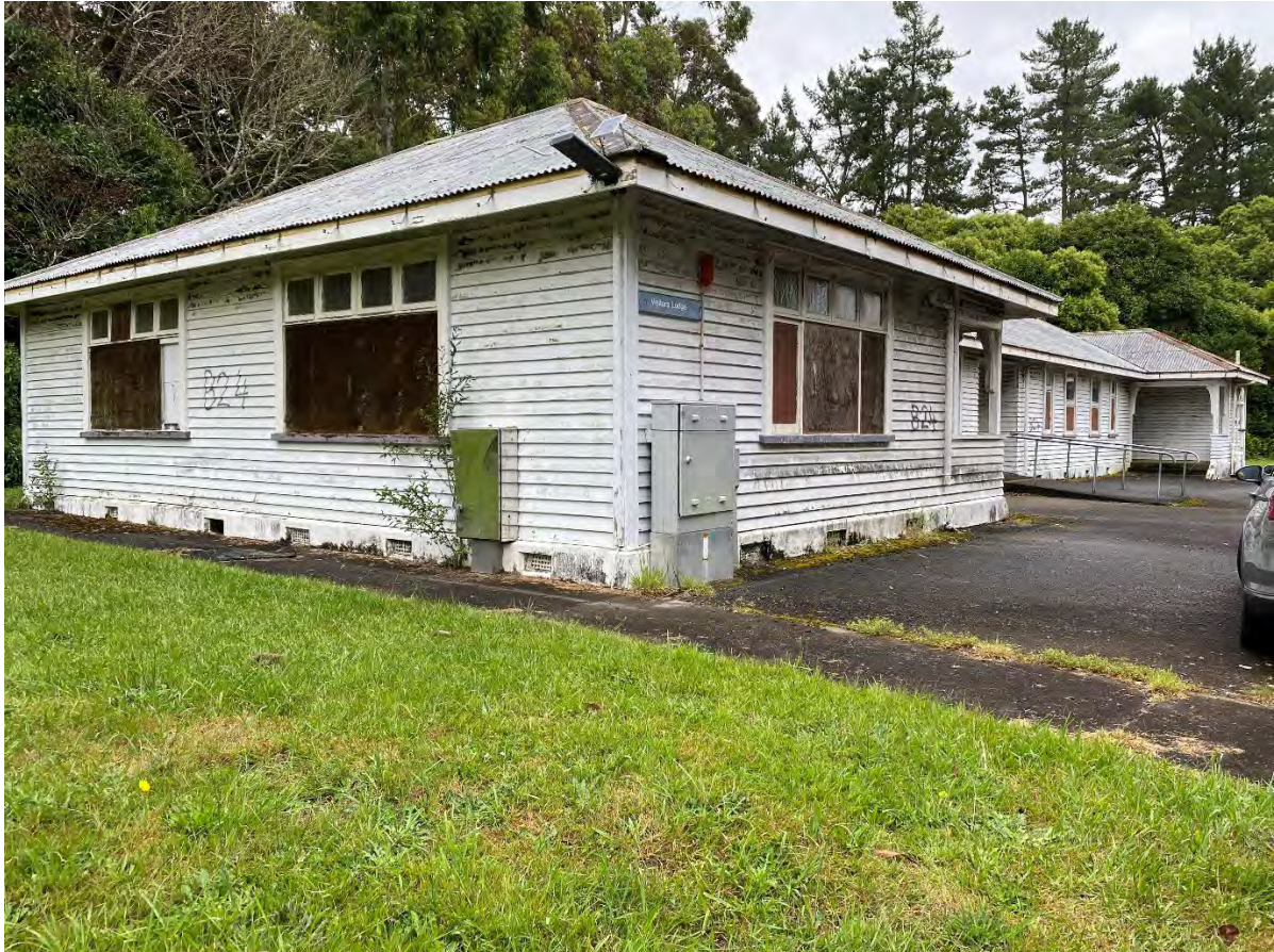
Figure 7: Site Photo of Existing Building on site
