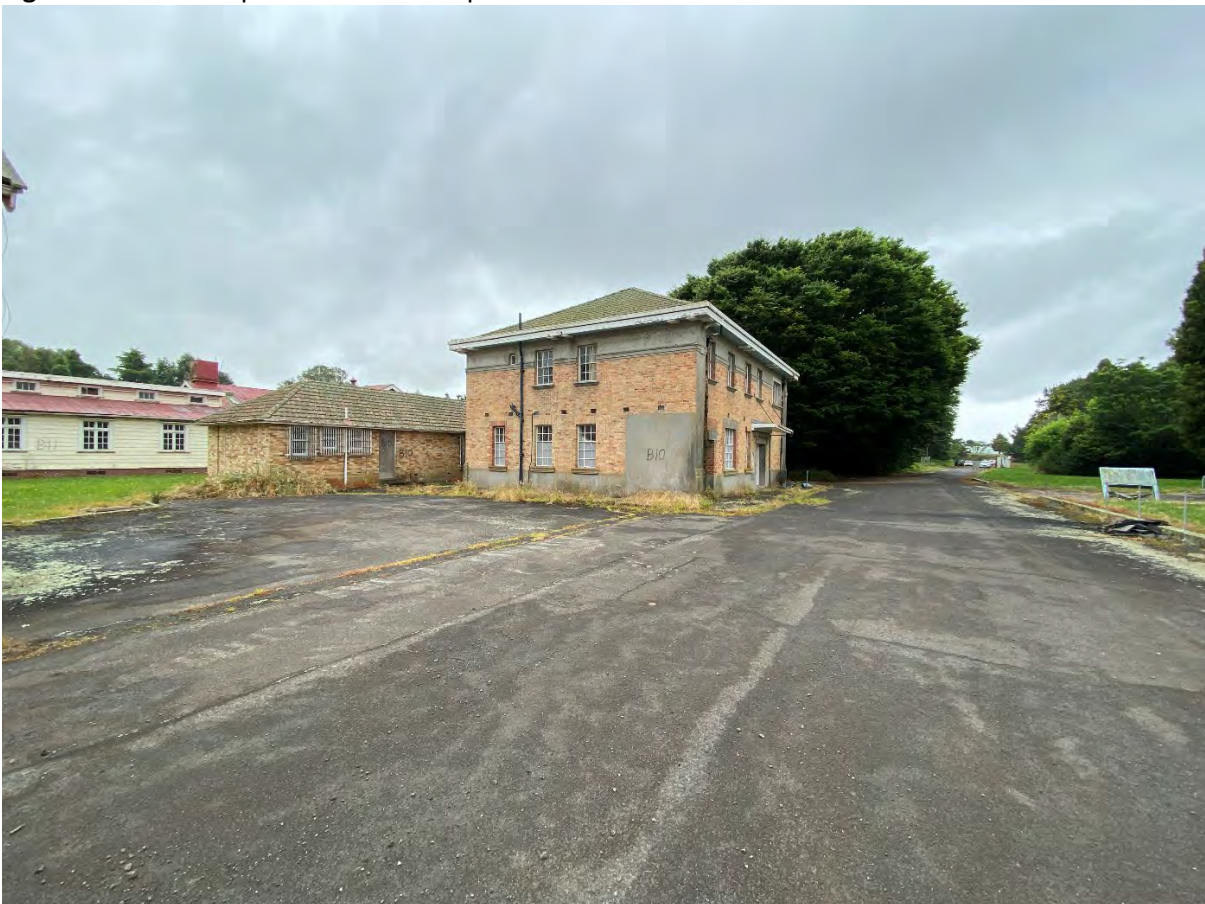
Figure 4: Site Photo of Existing Building on site
