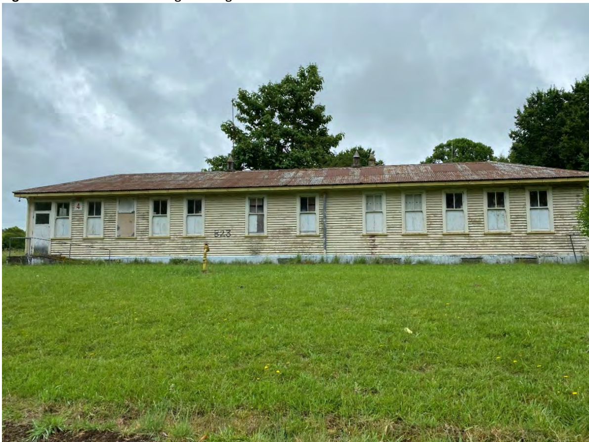
Figure 8: Site Photo of Existing Building on site
