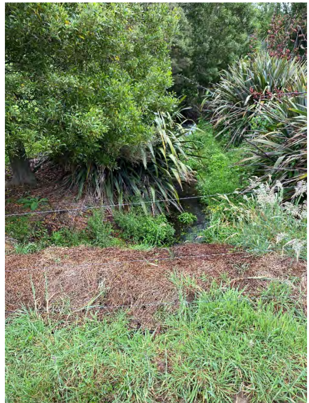
Figure 23: Site Photo looking towards Culvert 3
