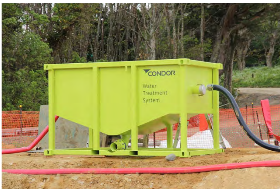
Figure 4: Example of Mobile Sediment Removal Device
