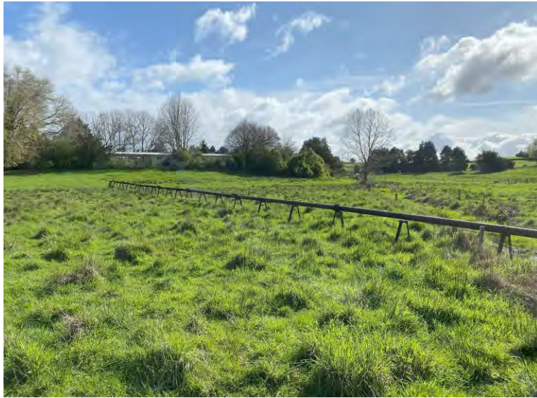
Southern pipeline with footings
