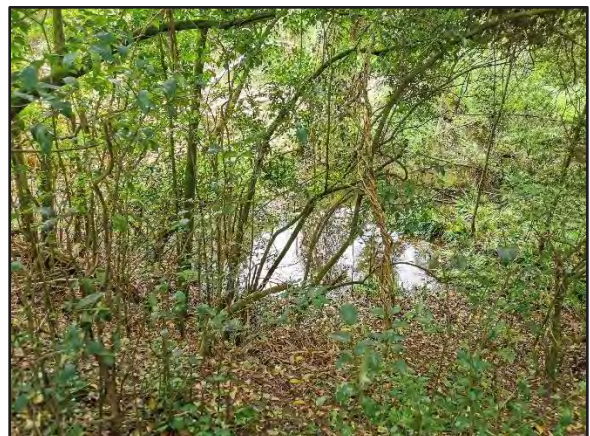
Photo 8: Upstream of Culvert 2, no flow evident.
