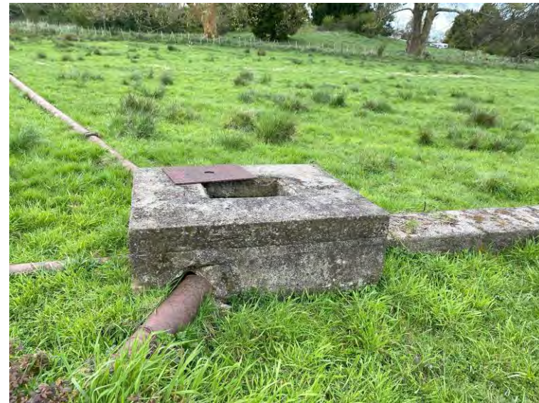
Concrete chamber connecting all four pipelines
