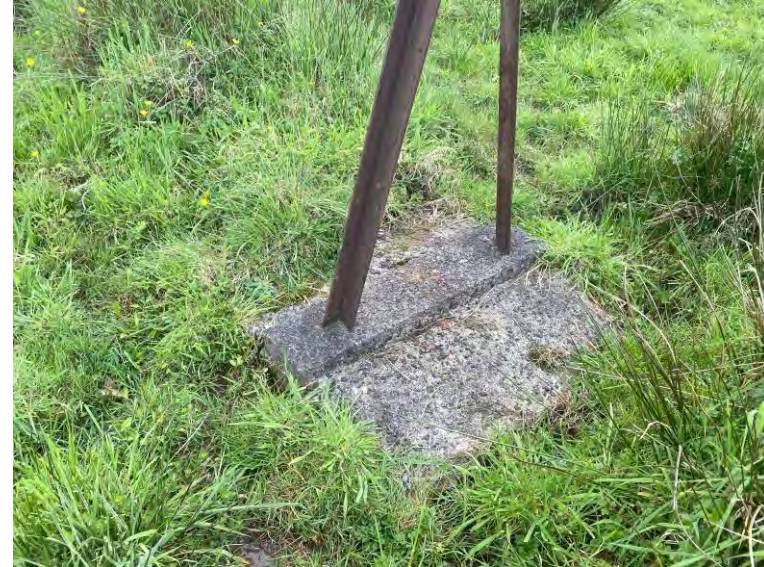
Southern pipeline footings and concrete foundation
