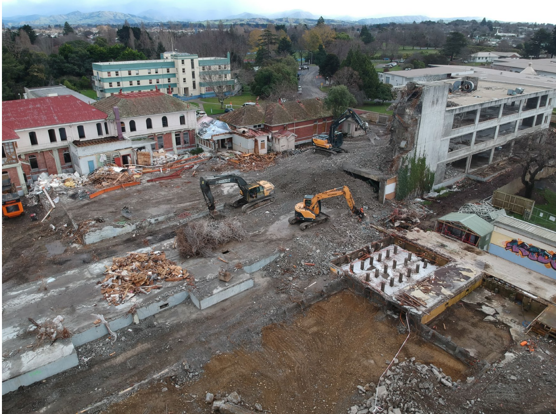
Image: Masterton Hospital Demolition
