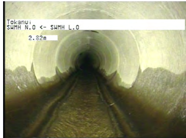
MH L.0 To MH N.O_bcd2da46-5308-4325-944e-bce3e7c063da_20230406_15 2657_067.jpg, 00:01:39, 2.82m
