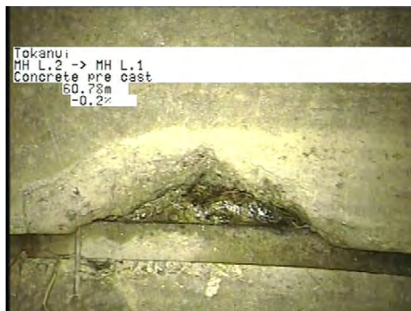
MH L.2 To MH L.1_efb44499-721b-4229-8c4f-42665233aa51_20230328_115 911_584.jpg, 00:18:10, 60.78m
