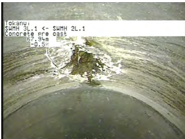
MH 2L.1 To MH 3L.1_03b9ea51-5a63-4fa5-8fff-331a83bb6ca2_20230406_122 114_253.jpg, 00:21:48, 67.94m
