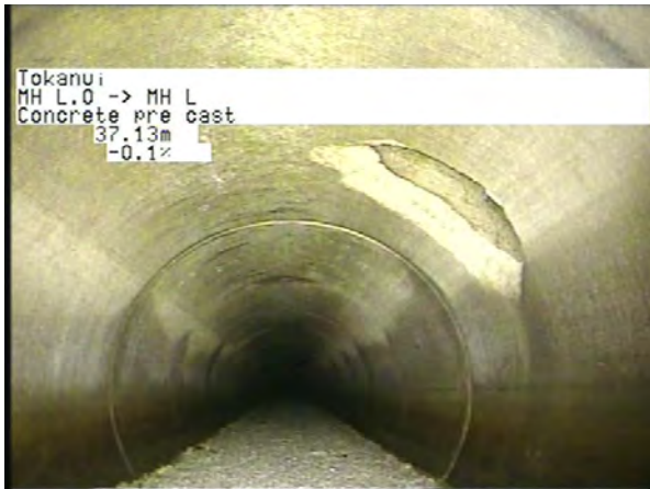
MH L.0 To MH L_058c85ea-b3dd-40c2-9b21-4372abf15b57_20230328_123653_311.jpg, 00:09:13, 37.13m
