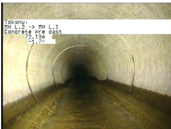
MH L.2 To MH L.1_05f56b3c-4af3-4120-90a2-48c31bdc07a0_20230328_120519_428.jpg, 00:23:16, 72.19m
