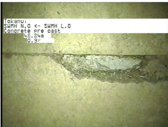
MH L.0 To MH N.0_bdf7bd39-fd77-4658-863c-e918b1a400a8_20230406_15 3452_225.jpg, 00:08:37, 48.84m
