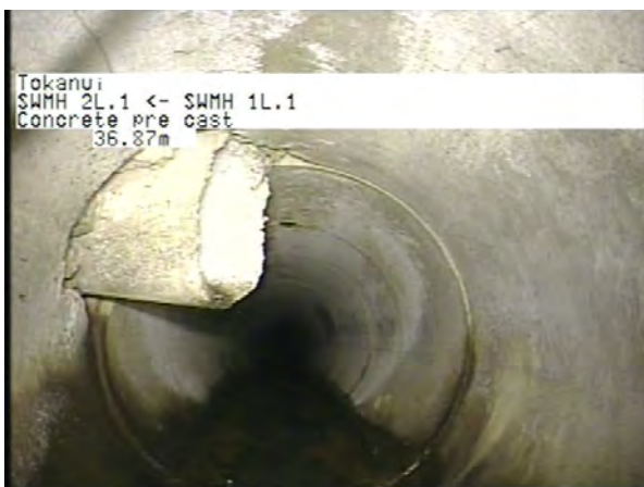
MH 1L.1 To MH 2L.1_38738545-3add-430d-b2eb-d071fc078472_20230406_1 33306_274.jpg, 00:11:26, 36.87m
