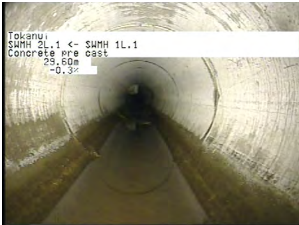
MH 1L.1 To MH 2L.1_67ad981e-242c-4808-939b-bc1a8066da8f_20230406_1 33036_044.jpg, 00:09:38, 29.60m
