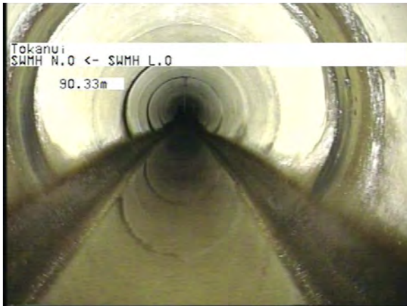
MH L.0 To MH N.0_69e208ac-ab81-40d5-bae9-4e431ffb17ef_20230406_154 329_172.jpg, 00:15:45, 90.33m
