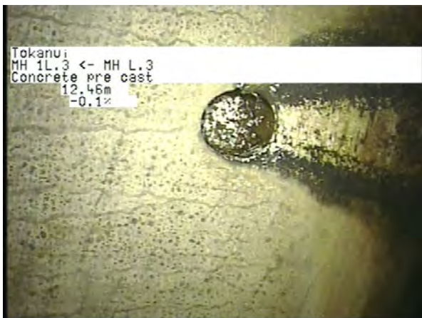
MH L.3 To MH 1L.3_0ecd87f5-1820-486d-8d32-f001d87cf676_20230404_10 3459_359.jpg, 00:05:33, 12.46m
