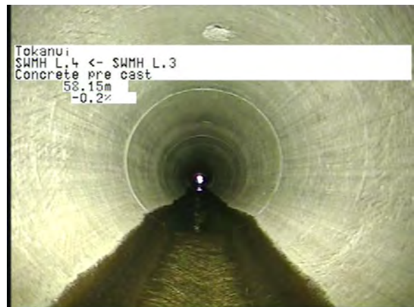
MH L.3 To MH L.4_1ab034b0-4456-4136-93f3-79203cee5797_20230404_09 4533_346.jpg, 00:15:13, 58.15m
