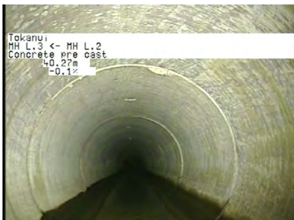
MH L.2 To MH L.3_64599a16-9a20-4a6e-8d0f-d6710a681735_20230328_140454_459.jpg, 00:13:08, 40.27m
