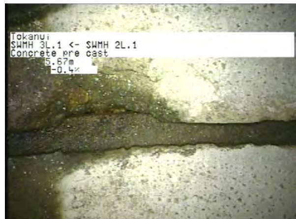
MH 2L.1 To MH 3L.1_e35f5190-348a-4a58-bd9f-28573eeeee306_20230406_11 5942_547.jpg, 00:02:41, 5.67m
