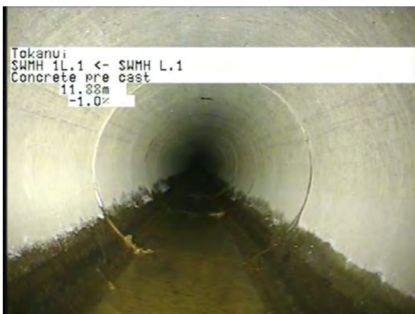
MH L.1 To MH 1L.1_a51cfb48-c721-495d-9475-12ef7ef4b782_20230404_12 0451_789.jpg, 00:04:48, 11.88m
