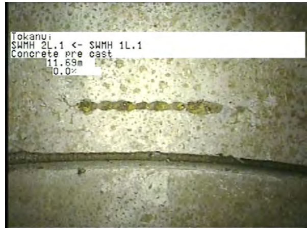
MH 1L.1 To MH 2L.1_9c730f4d-16b9-4017-8de4-735069fda835_20230404_12 5529_719.jpg, 00:02:51, 11.69m
