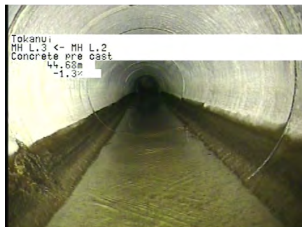
MH L.2 To MH L.3_d4aa0fbd-a310-427e-bb5c-b73b1572e744_20230328_140554_236.jpg, 00:14:00, 44.68m
