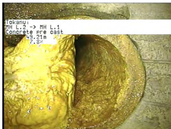
MH L.2 To MH L.1_f1743155-69ae-4a14-957b-195c700051c6_20230328_11 5338_028.jpg, 00:13:47, 49.21m
