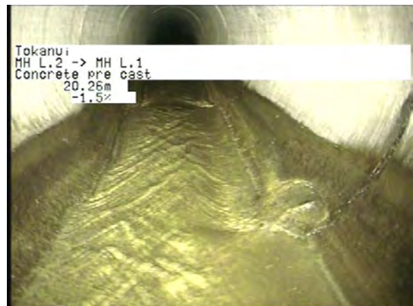
MH L.2 To MH L.1_16023d8f-7f34-4f61-87cd-a060305a2e5e_20230328_114 430_558.jpg, 00:06:14, 20.26m
