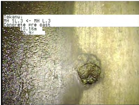
MH L.3 To MH 1L.3_660184ce-4980-4deb-ab86-f7affadb5d2a_20230404_10 3703_545.jpg, 00:06:59, 17.57m
