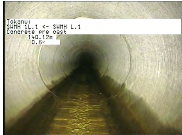
MH L.1 To MH 1L.1_1270f635-a8da-4348-895f-1a9997846ef4_20230404_12 4415_564.jpg, 00:36:59, 140.12m
