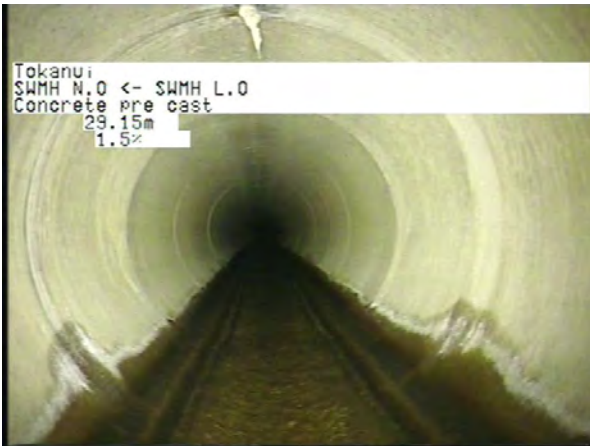
MH L.0 To MH N.0_c4d854e7-7c40-4eaf-a0d4-cc1a2f796d6c_20230406_153 239_211.jpg, 00:06:34, 29.15m
