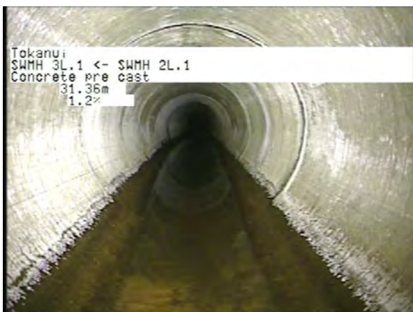
MH 2L.1 To MH 3L.1_e5591110-9edc-4d18-84b2-f6409b4e1367_20230406_1 20848_244.jpg, 00:11:03, 31.36m
