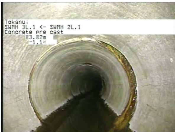
MH 2L.1 To MH 3L.1_13f3426a-5d68-482f-85e6-5cdaf74485b9_20230406_12 2629_068.jpg, 00:26:38, 83.82m
