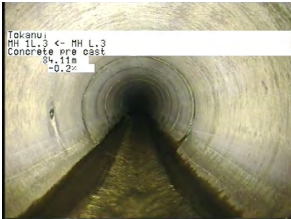
MH L.3 To MH 1L.3_c79736d4-5661-4711-8d29-eb5952b75ddd_20230404_1 05417_300.jpg, 00:22:20, 84.11m
