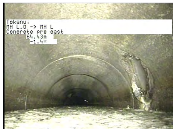
MH L.0 To MH L_673f452c-867c-44e7-b695-37a5a3c08713_20230328_124307_284.jpg, 00:14:35, 64.43m
