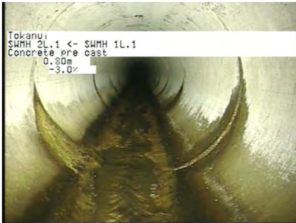
MH 1L.1 To MH 2L.1_d4559110-03d0-4742-ac00-2ab37aa6b3cb_20230406_1 31950_784.jpg, 00:00:57, 0.80m
