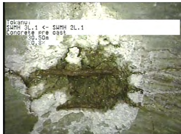
MH 2L.1 To MH 3L.1_3ef362ac-0bf4-4888-a7d1-e53af14c699f_20230406_120 742_982.jpg, 00:09:52, 29.99m
