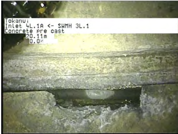
MH 3L.1 To 4L.1A Inlet_87e499ee-67c2-4bf4-9c4e-d0c141d2ad9f_20230406_14 3037_117.jpg, 00:05:22, 20.11m
