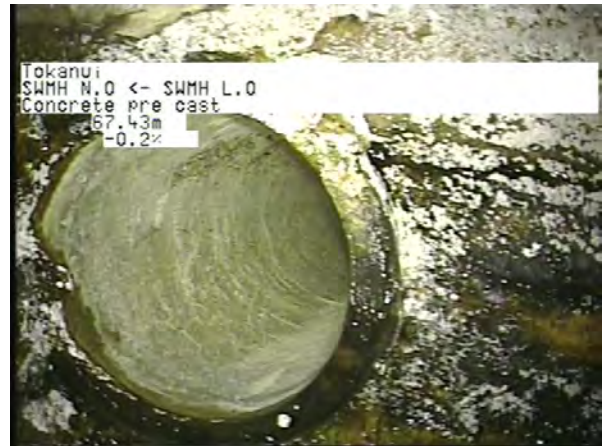
MH L.0 To MH N.0_8ef91109-dd1e-48f5-b4a7-1bee298a1b75_20230406_153811_012.jpg, 00:11:18, 67.43m
