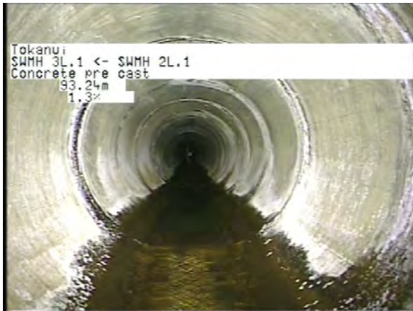
MH 2L.1 To MH 3L.1_e1d52d70-a10c-49b9-82e1-83502db2b1e9_20230406_1 22921_487.jpg, 00:29:01, 93.24m
