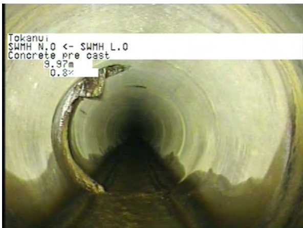
MH L.0 To MH N.O_7dc38427-e264-4876-8582-31f10e6f1f74_20230406_152 828_461.jpg, 00:03:00, 9.97m
