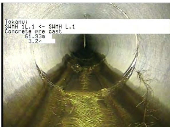
MH L.1 To MH 1L.1_3fb91a5d-147c-4c91-8f09-84a6609702d5_20230404_12 1955_441.jpg, 00:16:58, 61.93m
