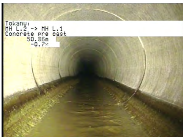
MH L.2 To MH L.1_5c75dd65-c56b-47f9-96e8-593603864276_20230328_11 5552_877.jpg, 00:15:01, 50.86m
