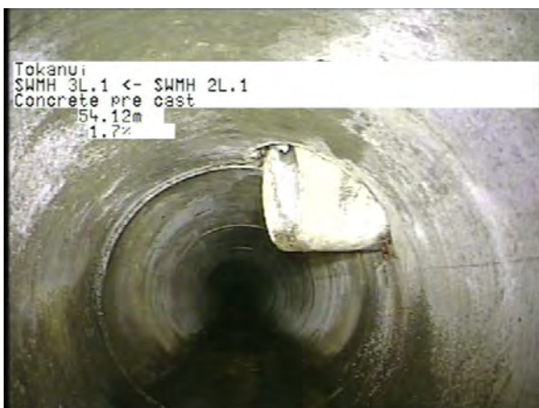
MH 2L.1 To MH 3L.1_6d6e23aa-cbe9-48e4-a1f1-a2cdcafd09a1_20230406_12 1559_281.jpg, 00:17:12, 54.13m
