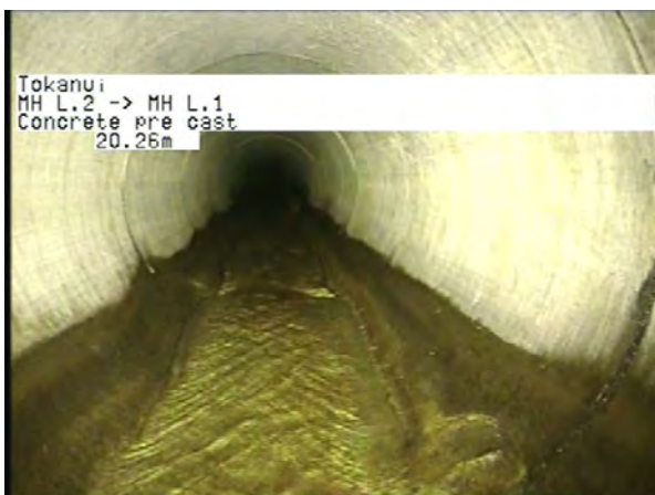
MH L.2 To MH L.1_1812caa0-d4a0-44e8-bd95-4cbe5cc6e1a2_20230328_11 4454_982.jpg, 00:06:19, 20.26m
