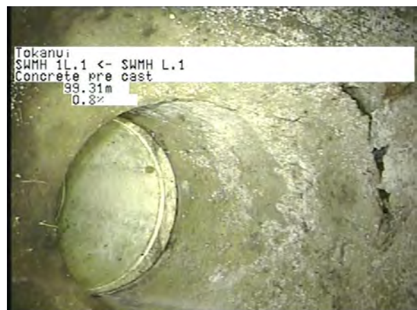
MH L.1 To MH 1L.1_dc82e9c0-edc4-4321-a016-a4ef2259fb45_20230404_12 3231_069.jpg, 00:26:42, 99.31m
