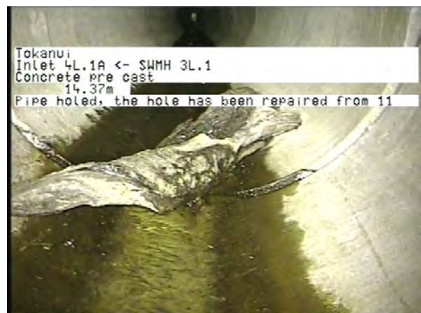
MH 3L.1 To 4L.1A Inlet_0a5fc193-8175-4f24-b7fc-62fa2161c2dc_20230406_142 911_003.jpg, 00:03:51, 14.37m
