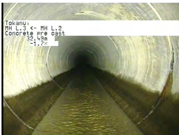
MH L.2 To MH L.3_568339f8-f189-43ca-bc6b-fe03ac71797e_20230328_14056_140.jpg, 00:10:10, 32.49m
