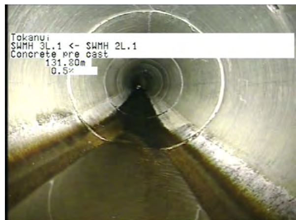
MH 2L.1 To MH 3L.1_0fb4beae-e805-4480-b9f5-c4db597143a4_20230406_12 3805_012.jpg, 00:37:05, 131.80m
