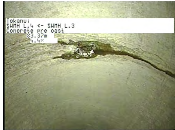
MH L.3 To MH L.4_cd437be2-9ea3-414e-b7ee-161ba26f5424_20230404_09 5133_886.jpg, 00:20:28, 83.37m
