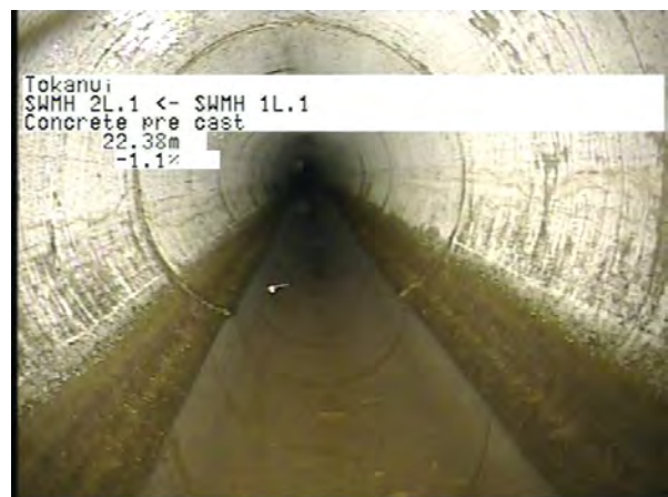
MH 1L.1 To MH 2L.1_cf8b62ef-b751-4901-9600-9a2f4e4a00fd_20230406_132 903_909.jpg, 00:08:13, 22.38m
