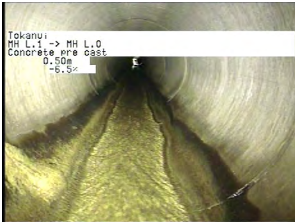
MH L.1 To MH L.O_01bfe479-5985-457c-a0fb-1c946f6e2a24_20230328_121 819_172.jpg, 00:00:21, 0.50m
