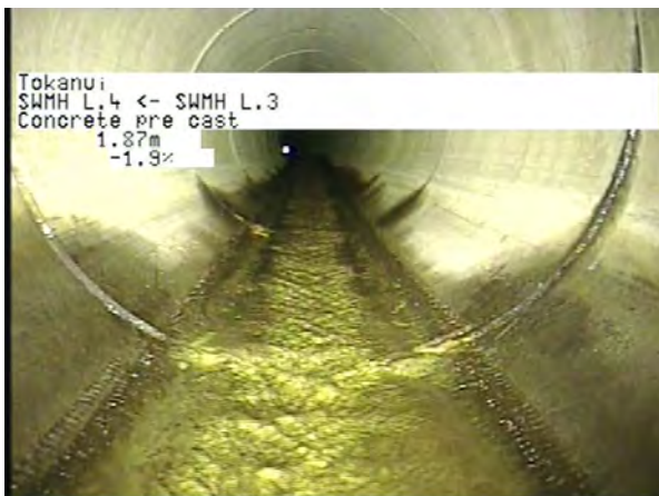
MH L.3 To MH L.4_e2f87596-29fe-4ec1-934e-0f3ccad4d5b2_20230404_093 057_865.jpg, 00:02:46, 1.87m
