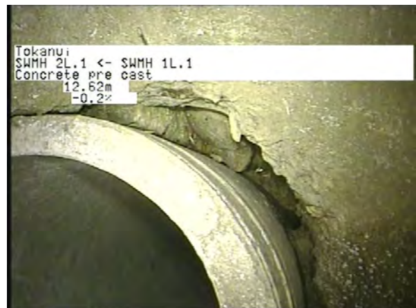
MH 1L.1 To MH 2L.1_324b1f6d-28ae-4dbf-a417-5cecea7b1012_20230404_12 5708_954.jpg, 00:03:56, 12.62m
