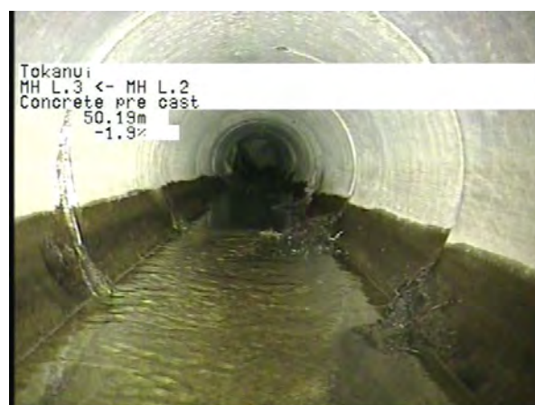
MH L.2 To MH L.3_7a485f99-6caa-477c-ae76-26ec77a4d9a1_20230328_140843_916.jpg, 00:16:16, 50.19m
