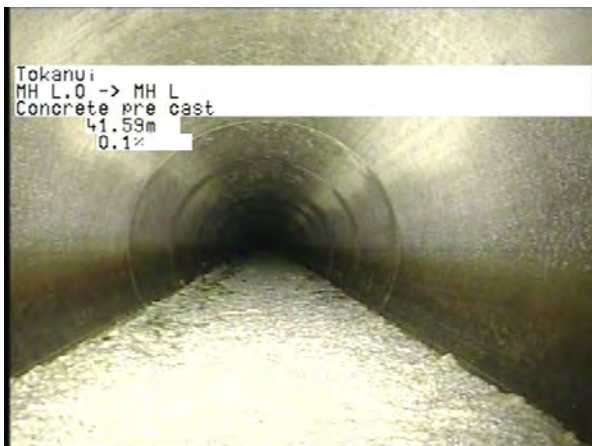
MH L.0 To MH L_c681fdcc-d3b5-4cdf-903f-81a6f0852f94_20230328_123845_352.jpg, 00:10:54, 41.59m
