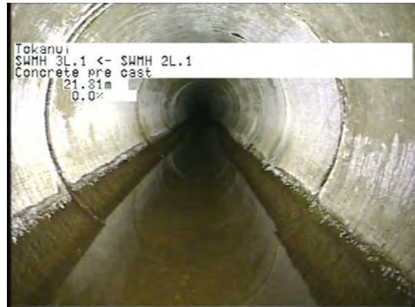
MH 2L.1 To MH 3L.1_e31beec-a341-4644-9dc6-b9bd917d6d67_20230406_1 20447_477.jpg, 00:07:18, 21.81m
