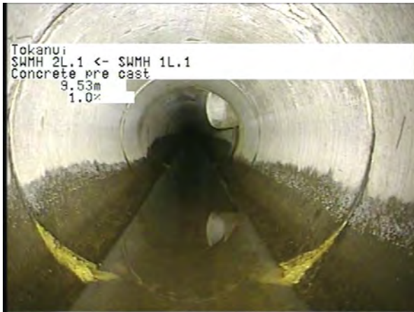
MH 1L.1 To MH 2L.1_9f3b7746-20b1-435a-bcc7-c81218aa085a_20230404_1 25500_217.jpg, 00:02:28, 9.53m
