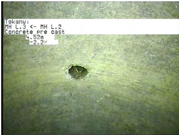
MH L.2 To MH L.3_b5486849-fbf5-4630-8596-273ccbec6469_20230328_134 815_657.jpg, 00:01:15, 4.52m
