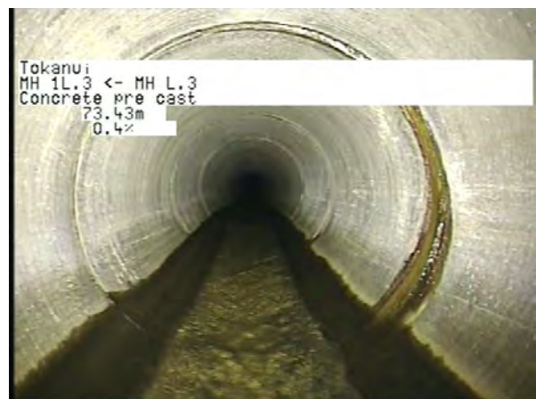
MH L.3 To MH 1L.3_86797a0e-c2d7-4d35-8631-55ad125fb115_20230404_1 05120_199.jpg, 00:19:33, 73.43m
