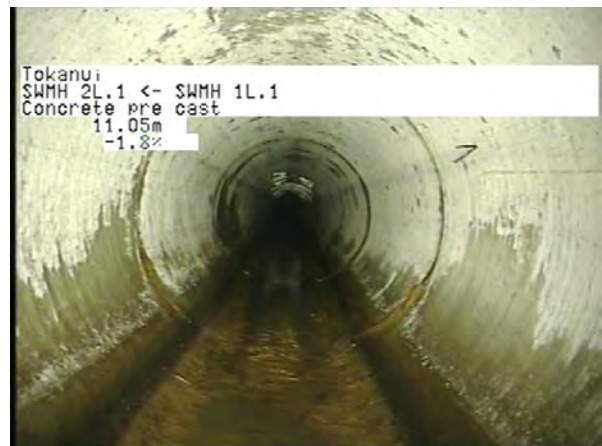
MH 1L.1 To MH 2L.1_a2ecf20a-1bbc-4f12-b816-bc1f694962aa_20230406_13 2511_680.jpg, 00:04:44, 11.05m
