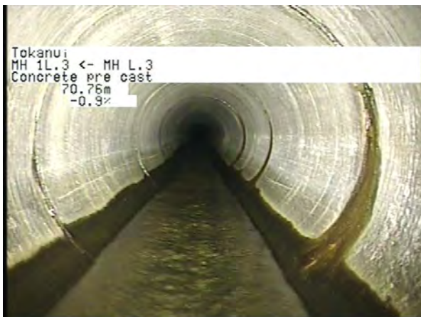
MH L.3 To MH 1L.3_1250d530-7bdd-418a-b5fe-2f673034d37f_20230404_10 5017_902.jpg, 00:19:01, 70.76m
