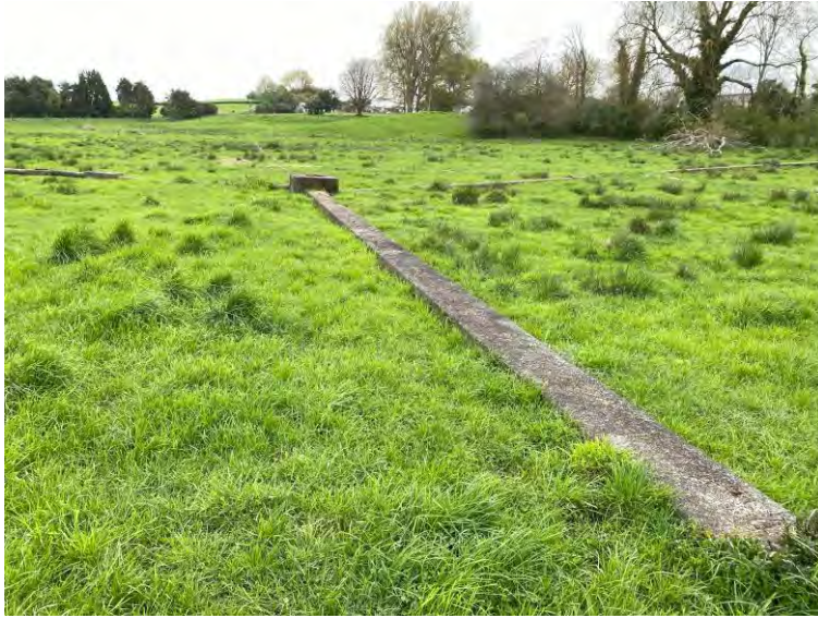
Eastern pipeline within concrete chamber
