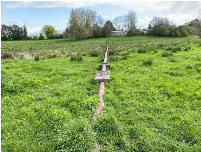
Southern pipeline with concrete casing
