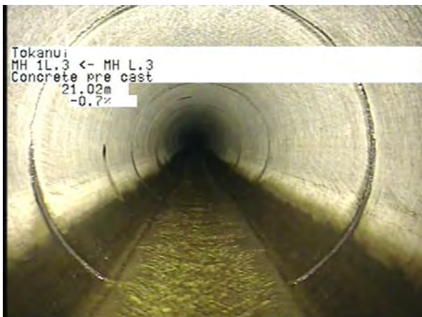
MH L.3 To MH 1L.3_29ce032d-9b10-4b6c-b26b-c9792552ccf2_20230404_10 3814_801.jpg, 00:07:50, 21.02m
