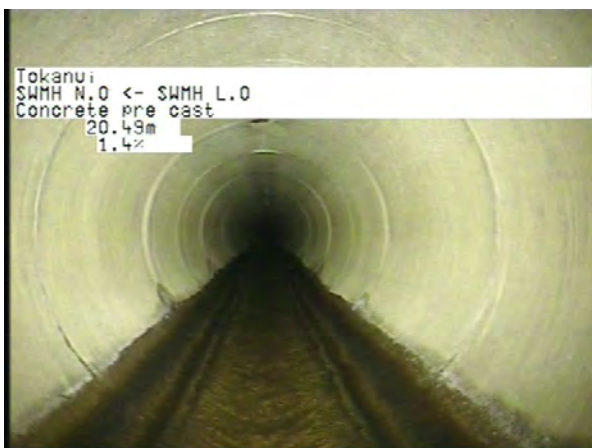
MH L.0 To MH N.O_d65ad6a2-e3ab-4f0f-81eb-6eaac14ceb03_20230406_15 3109_779.jpg, 00:05:17, 20.49m
