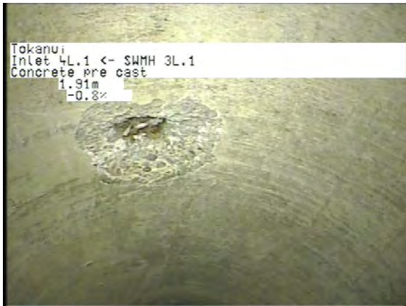
MH 3L.1 To Outlet 4L.1_1abac5b6-8670-4230-94b7-bd4fef31e91e_20230406_12 4535_589.jpg, 00:00:56, 1.91m
