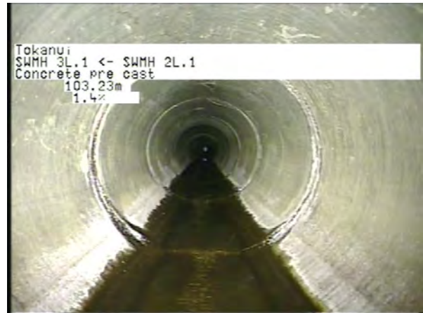
MH 2L.1 To MH 3L.1_155a9132-91b5-4f1b-97ed-c7b638091c30_20230406_1 23152_268.jpg, 00:31:26, 103.23m
