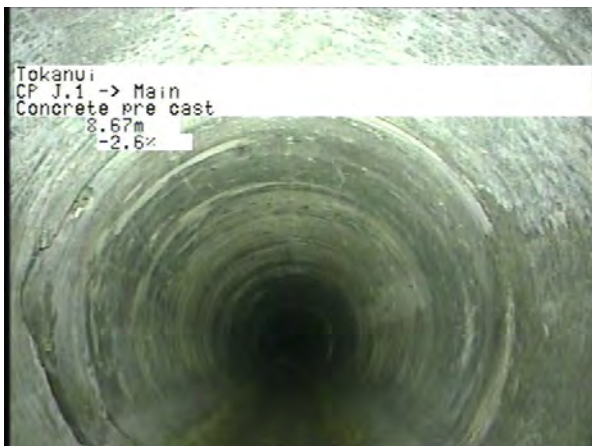
CP J.1 To Main_5be21a3c-ac2a-4955-96c5-c1514c1df63f_20230327_125954_613.jpg, 00:03:06, 8.67m
