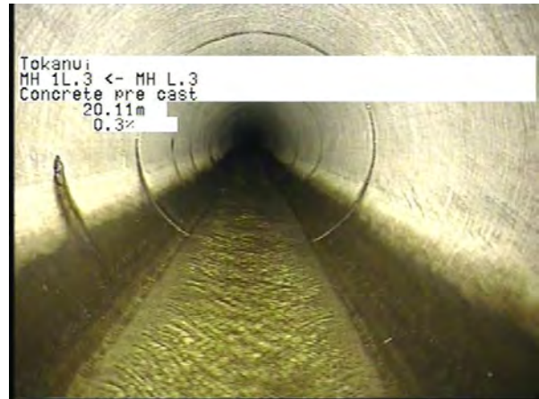
MH L.3 To MH 1L.3_0be531a1-51f3-4133-92f4-60a50cd26c59_20230404_10 3749_262.jpg, 00:07:37, 20.11m
