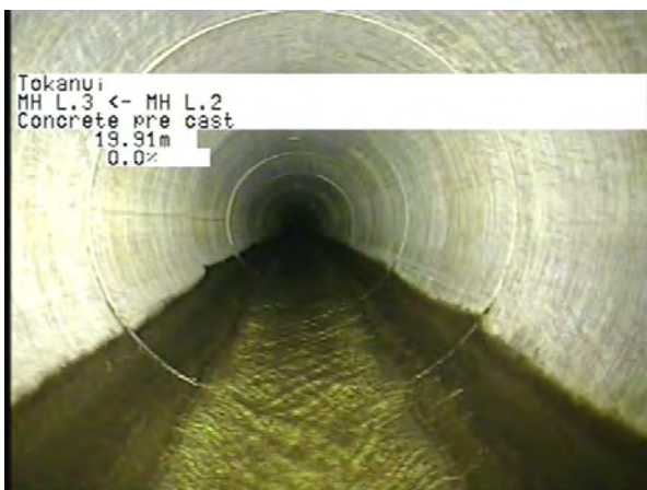
MH L.2 To MH L.3_4e1ad88c-6513-485a-8ae7-f95aea91eb4e_20230328_13 5616_257.jpg, 00:06:49, 19.91m
