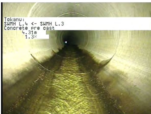
MH L.3 To MH L.4_a4b88312-16c3-479b-aef9-69c133b0f164_20230404_093 233_851.jpg, 00:03:51, 4.33m
