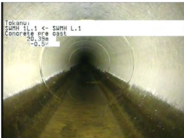
MH L.1 To MH 1L.1_4d264062-72ec-4b23-9a35-fa8798e3465f_20230404_12 0907_321.jpg, 00:07:47, 20.39m
