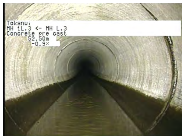
MH L.3 To MH 1L.3_e3136017-e4c8-4a80-871b-724d2b483ce9_20230404_1 04516_055.jpg, 00:14:27, 52.50m
