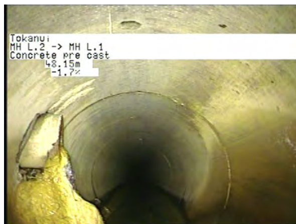
MH L.2 To MH L.1_2b036aa8-bd7c-4b10-ac49-301e16fa4047_20230328_11 5220_452.jpg, 00:12:53, 48.15m
