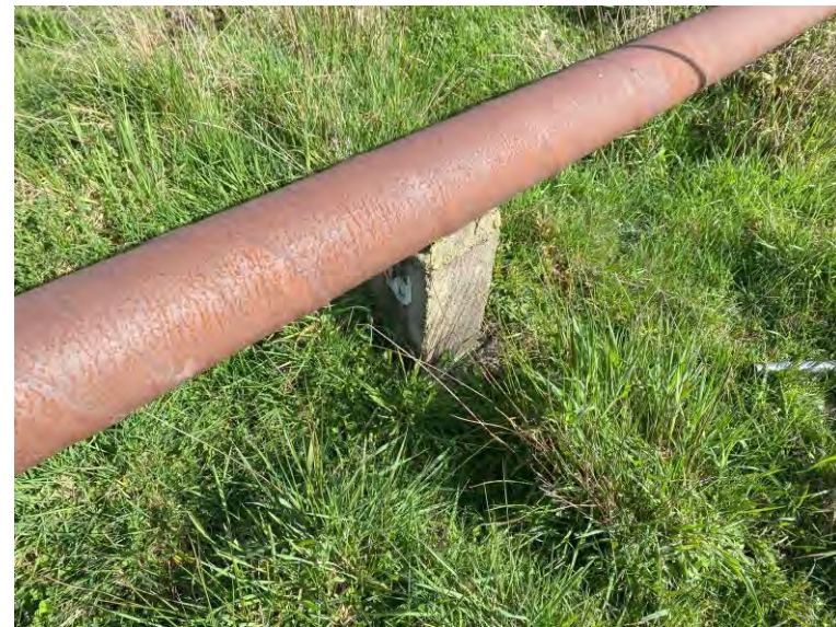
Southern pipeline with concrete pile
