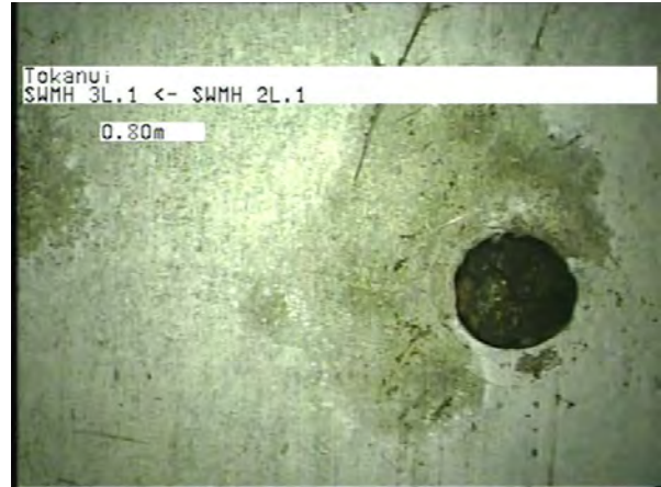
MH 2L.1 To MH 3L.1_f3e577a9-28ba-4560-b89e-0da46a5d7ccd_20230406_1 15700_124.jpg, 00:00:19, 0.80m
