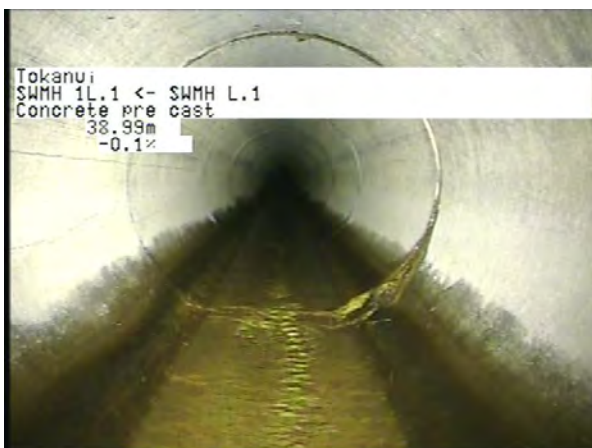
MH L.1 To MH 1L.1_5cd2019c-ff89-4b03-994a-e4ca7ae62175_20230404_12 1318_924.jpg, 00:11:39, 38.99m
