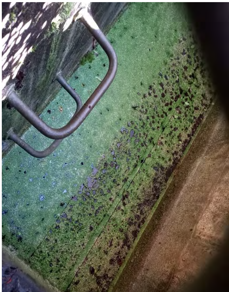
Figure 28: Inside of grit chamber
