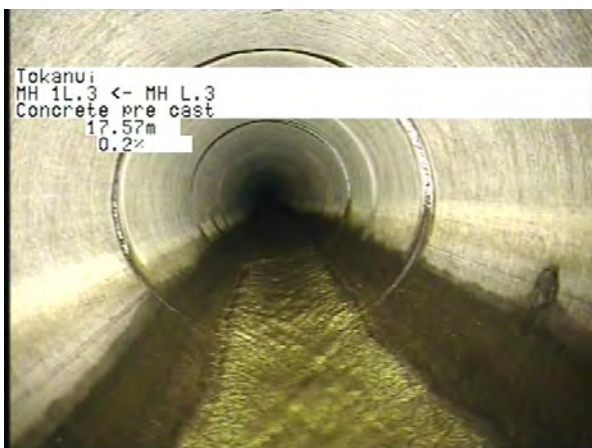
MH L.3 To MH 1L.3_81ca6150-c54d-46d4-87ae-a1ad59e814ac_20230404_1 03641_628.jpg, 00:06:57, 17.57m
