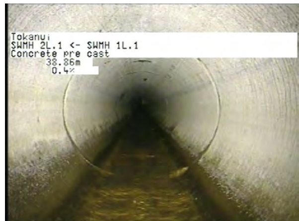
MH 1L.1 To MH 2L.1_6eebb0b5-4458-4d8c-be4b-18553b91225f_20230404_1 30447_801.jpg, 00:10:42, 38.86m
