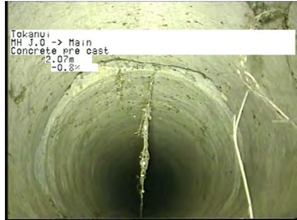
CP J.0 To Main_7587a93c-4c5c-4505-bc90-22155f335ad2_20230327_1 33718_936.jpg, 00:01:30, 2.07m
