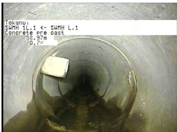
MH L.1 To MH 1L.1_35d0d170-0f81-4417-84fc-51ead01dbb7a_20230404_12 1828_648.jpg, 00:16:02, 58.97m
