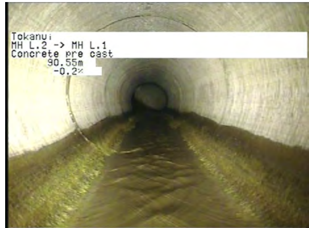
MH L.2 To MH L.1_7b631029-85b6-4662-a0aa-34b32d2fd38b_20230328_12 1032_751.jpg, 00:28:10, 90.55m
