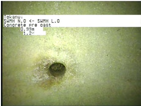
MH L.0 To MH N.O_d86cde5e-42e8-4368-8579-a99ad8755ca5_20230406_15 2537_334.jpg, 00:00:25, 0.99m
