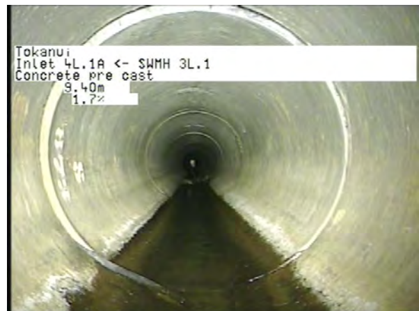
MH 3L.1 To 4L.1A Inlet_47aebede-4187-4981-a74e-e369e4ee9c31_20230406_1 42704_666.jpg, 00:02:26, 9.40m
