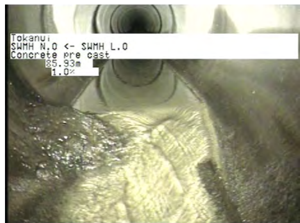
MH L.0 To MH N.0_788a8711-d5b1-4c5f-aaa8-4dbfa7651d49_20230406_154224_533.jpg, 00:14:48, 85.93m
