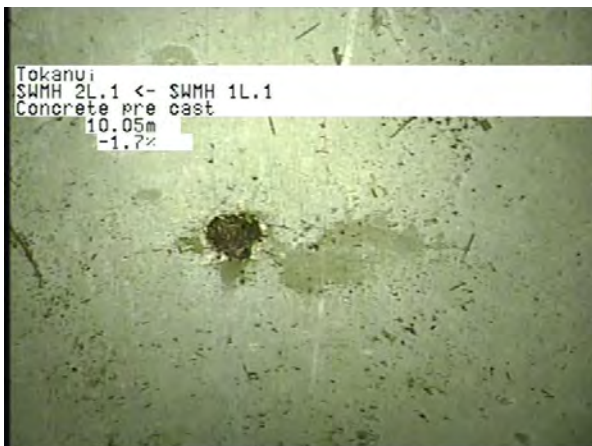
MH 1L.1 To MH 2L.1_eda2b90a-1d1c-4106-9b4f-754491419473_20230406_1 32413_569.jpg, 00:03:53, 10.05m
