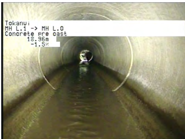
MH L.1 To MH L.O_57ddf494-7e4a-4875-9188-35cb15678539_20230328_12 222_671.jpg, 00:04:06, 18.96m
