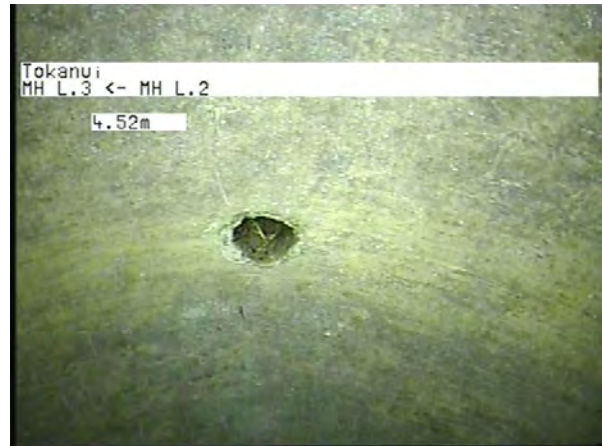
MH L.2 To MH L.3_f987bf23-4756-4827-ae23-684241dcd8ca_20230328_134 826_521.jpg, 00:01:15, 4.52m
