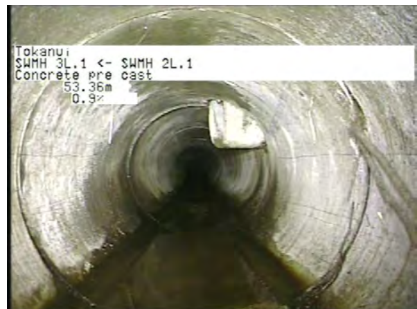
MH 2L.1 To MH 3L.1_da89f198-a029-4dd7-9e50-f13d7dbff8b4_20230406_121 540_689.jpg, 00:17:02, 53.36m
