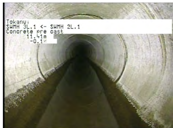
MH 2L.1 To MH 3L.1_c3161c03-8bab-4901-adc5-2b3b1994c4df_20230406_12 0147_401.jpg, 00:04:30, 11.41m
