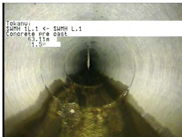
MH L.1 To MH 1L.1_217acfb7-81a1-48f4-9c33-f982301366d5_20230404_12 2102_027.jpg, 00:17:54, 63.11m
