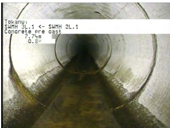
MH 2L.1 To MH 3L.1_ad2d04a8-5c22-4e96-a7b5-048c418ce6a8_20230406_1 20026_135.jpg, 00:03:17, 7.74m
