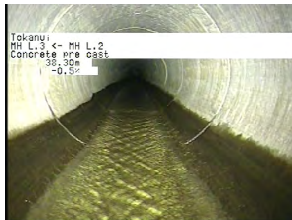
MH L.2 To MH L.3_20816295-8f31-4580-ae7c-6c200e2ecbbd_20230328_140247_469.jpg, 00:11:54, 38.30m
