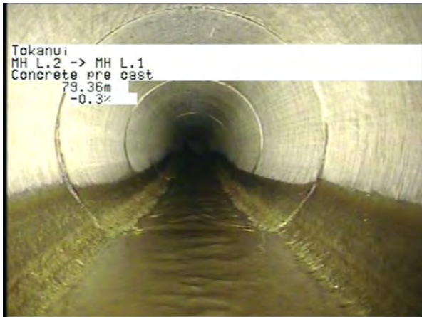
MH L.2 To MH L.1_992a1c25-3d75-46ce-a01f-b7ca6963de68_20230328_12 0814_157.jpg, 00:25:58, 79.36m
