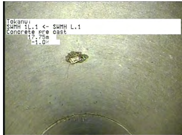
MH L.1 To MH 1L.1_f79701cd-4f67-44d8-b66a-579e775648a5_20230404_12 0734_042.jpg, 00:06:47, 17.75m
