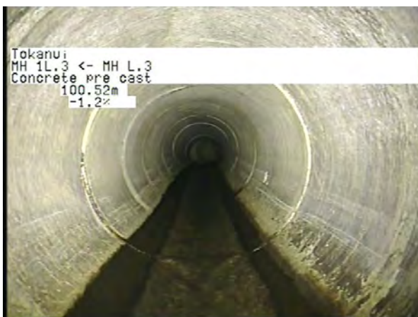
MH L.3 To MH 1L.3_2f22ebd9-a633-4f45-98d5-41e8c925061f_20230404_10 5946_440.jpg, 00:26:54, 100.52m
