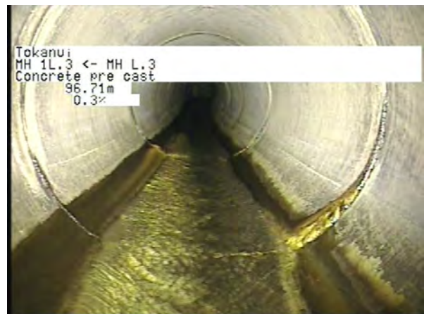
MH L.3 To MH 1L.3_f5160bf1-0893-409a-93c1-d7c758f5e3a8_20230404_10 5820_973.jpg, 00:25:40, 96.71m
