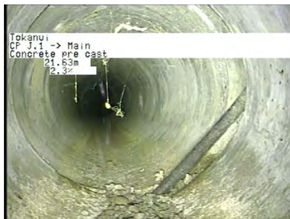
CP J.1 To Main_be7a1704-4782-4de7-878e-bddef75a6674_20230327_1 30558_456.jpg, 00:07:42, 21.63m
