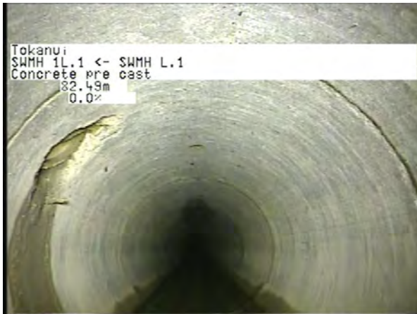
MH L.1 To MH 1L.1_44b9a4b4-8ea3-4557-abc0-f63d0688fcb3_20230404_12 2745_592.jpg, 00:22:53, 82.49m
