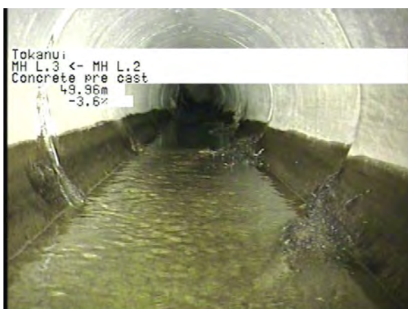
MH L.2 To MH L.3_e372af21-6ca6-4a1f-ac4a-0894e8a8c844_20230328_140718_267.jpg, 00:15:12, 49.96m
