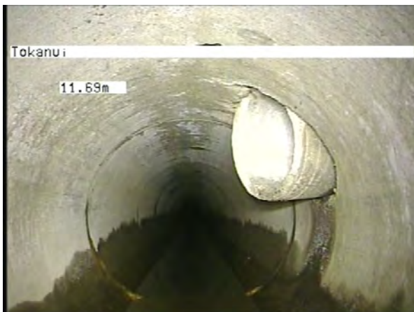
MH 1L.1 To MH 2L.1_ddc7b103-169d-44bc-a0cb-142f49ae2616_20230404_1 25634_590.jpg, 00:03:25, 11.69m
