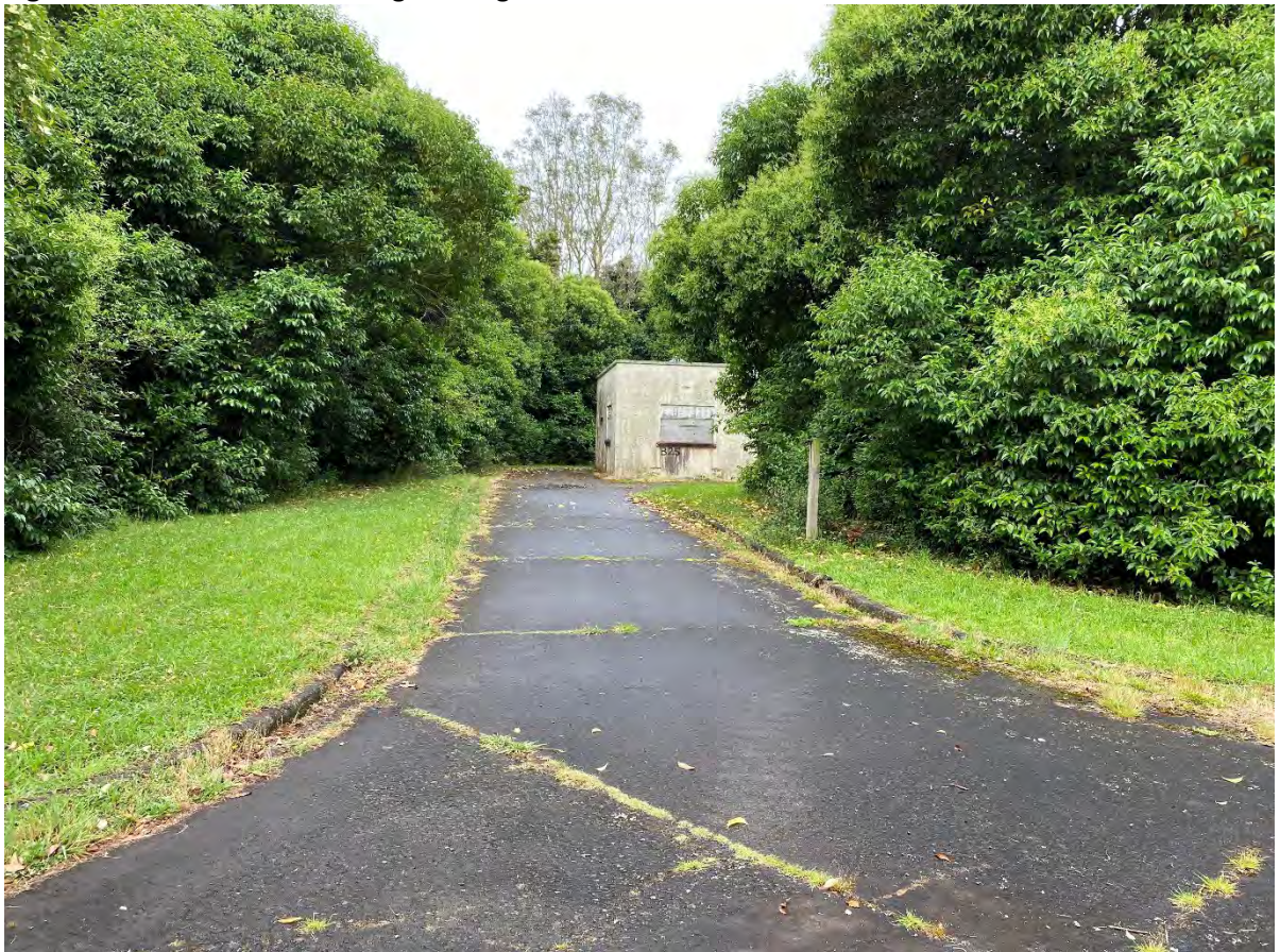
Figure 18: Site Photo of existing roading on site
