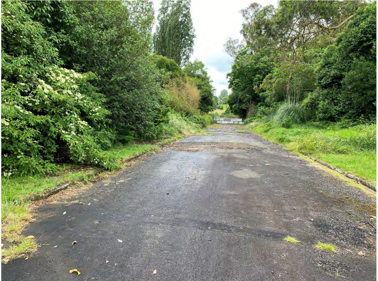
Figure 17: Site Photo of existing roading on site
