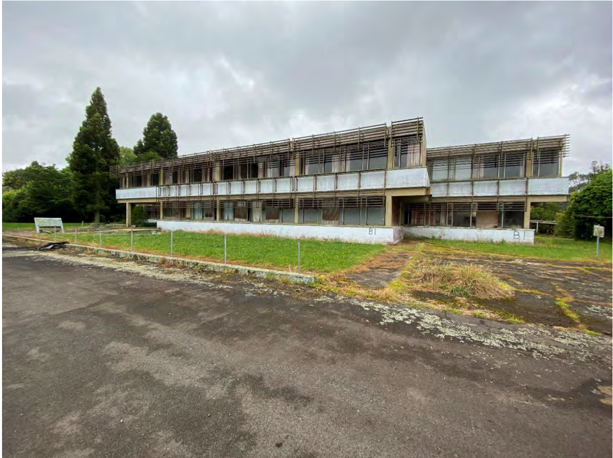
Figure 5: Site Photo of Existing Building on site
