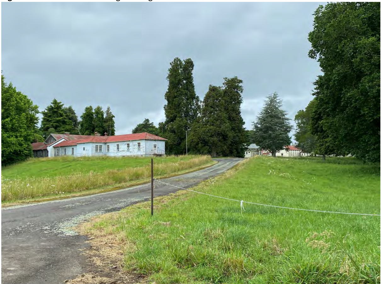
Figure 14: Site Photo of Existing Building on site
