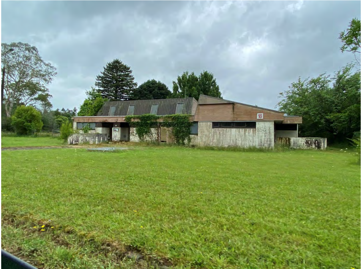
Figure 13: Site Photo of Existing Building on site
