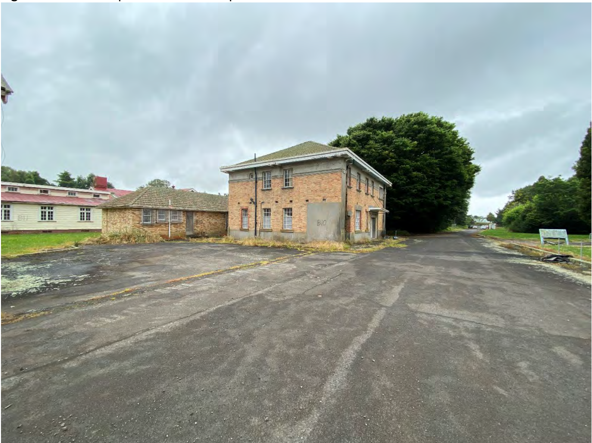
Figure 4: Site Photo of Existing Building on site
