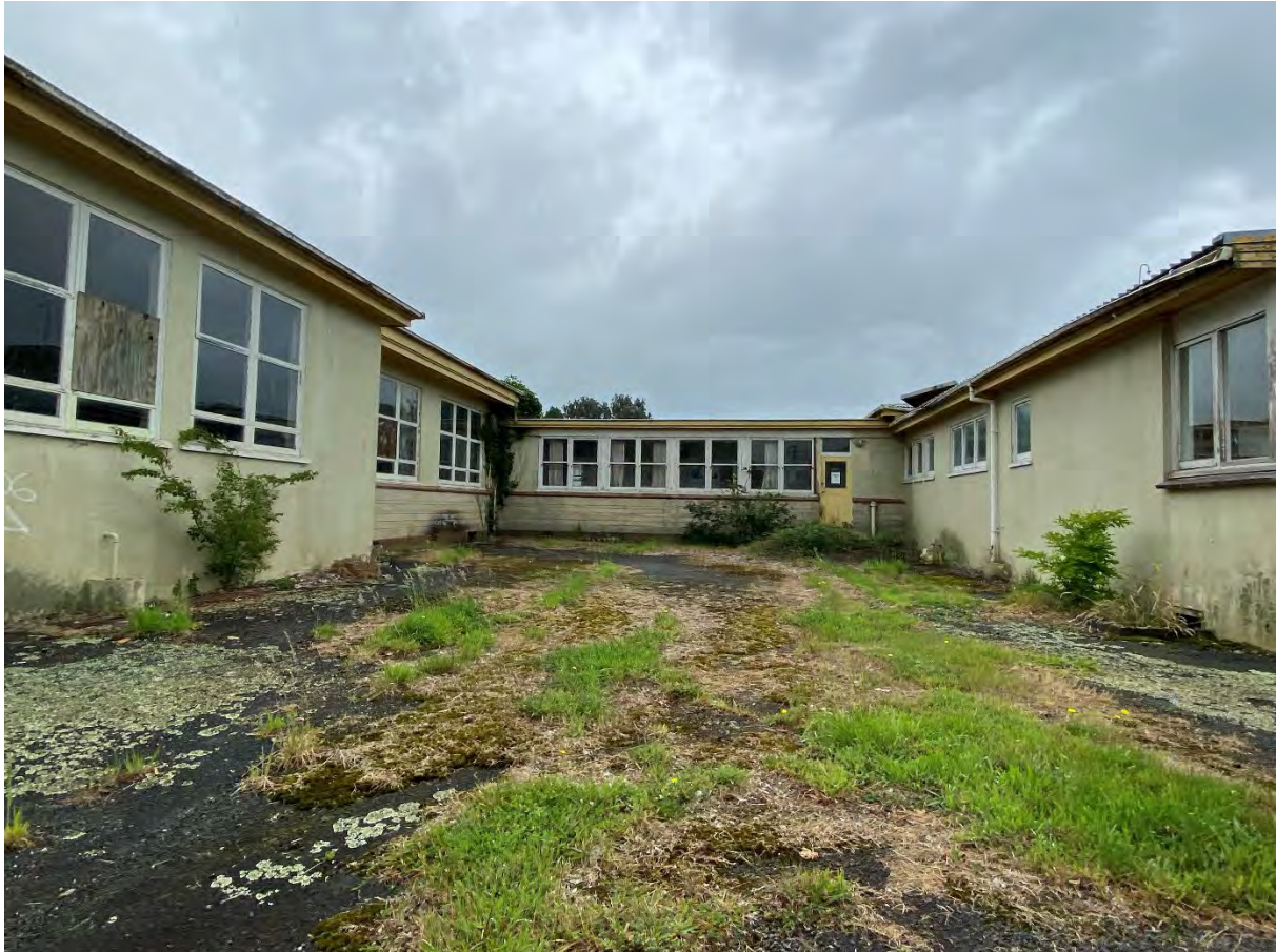
Figure 15: Site Photo of existing building on site
