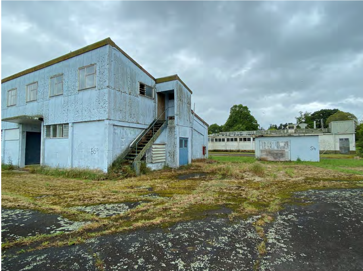
Figure 11: Site Photo of Existing Building on site
