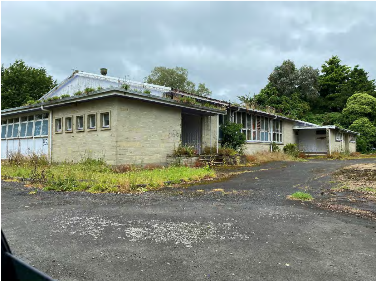
Figure 12: Site Photo of Existing Building on site
