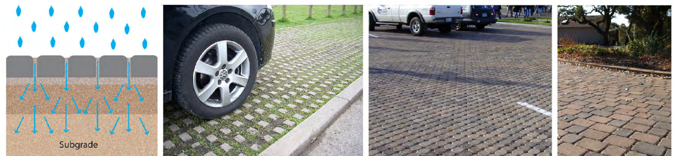
Figure 33: Permeable paving stones allow filtration of rain water into the earth, reducing pressure on stormwater infrastructure.
