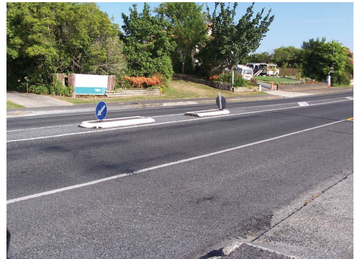
Figure 9: Existing informal pedestrian crossing across the State Highway north of Ohaupo town centre. Traffic calming measures should be undertaken throughout Ohaupo to create safe pedestrian crossings for all people.
