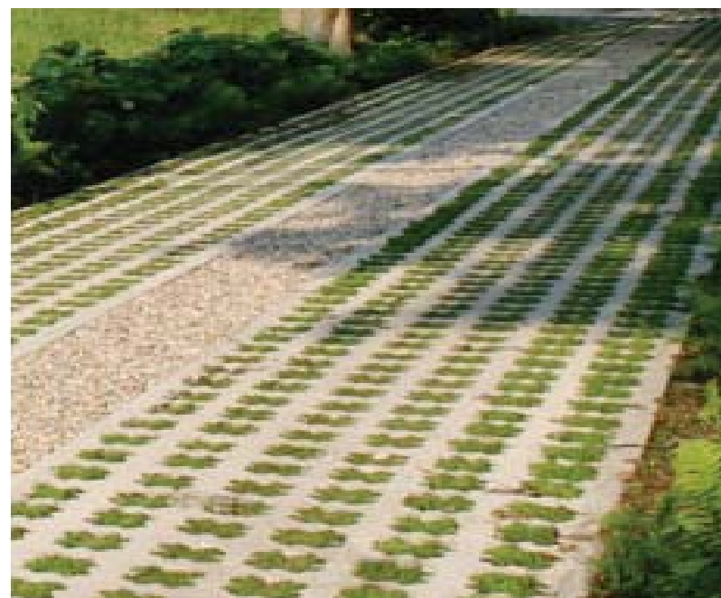
Figure 15: Example of permeable paving surface
