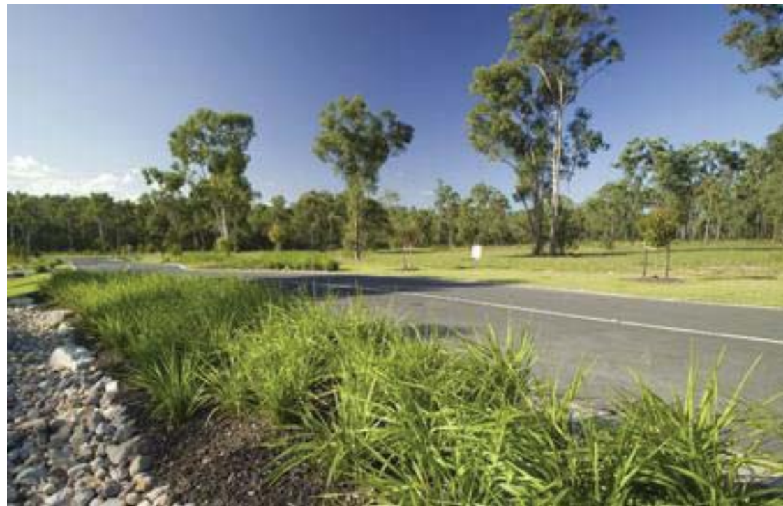
Figure 16: Example of a roadside swale.
