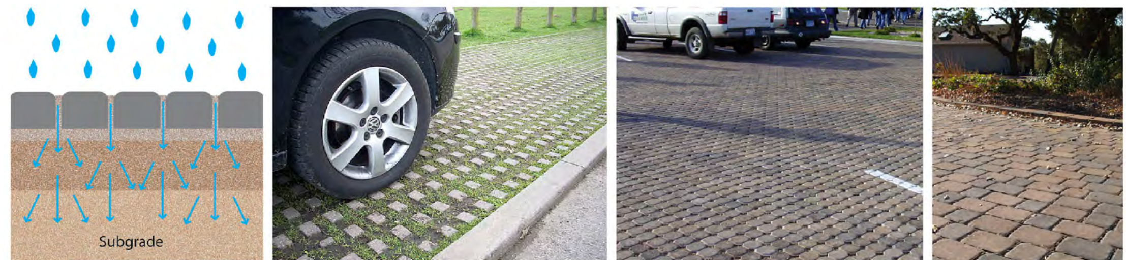
Figure 10: use of permeable paving surfaces in residential, commercial and street parking areas will decrease the impact on stormwater infrastructure.
