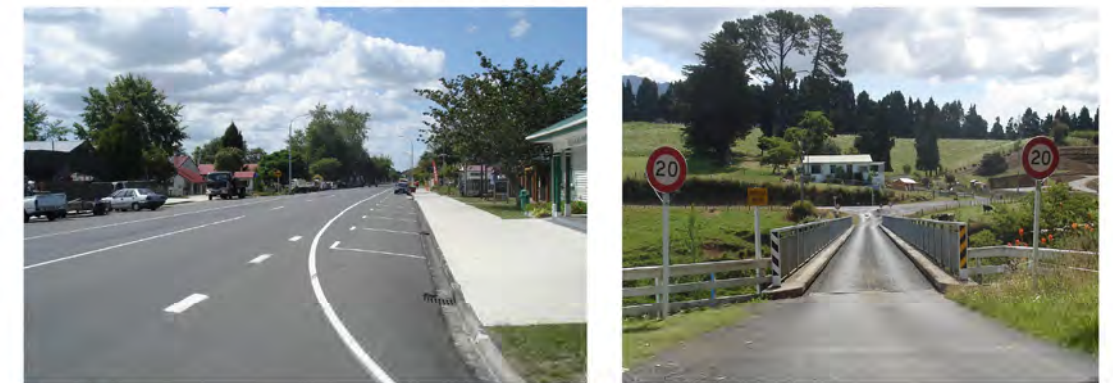
Figure 5: State Highway 39 and bridge crossing over the Waipa River
