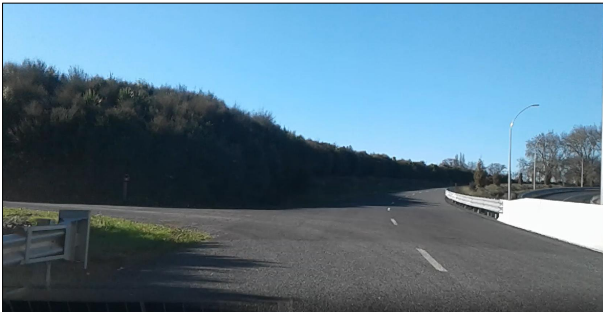
Figure 4: Vehicle Crossing to Site
