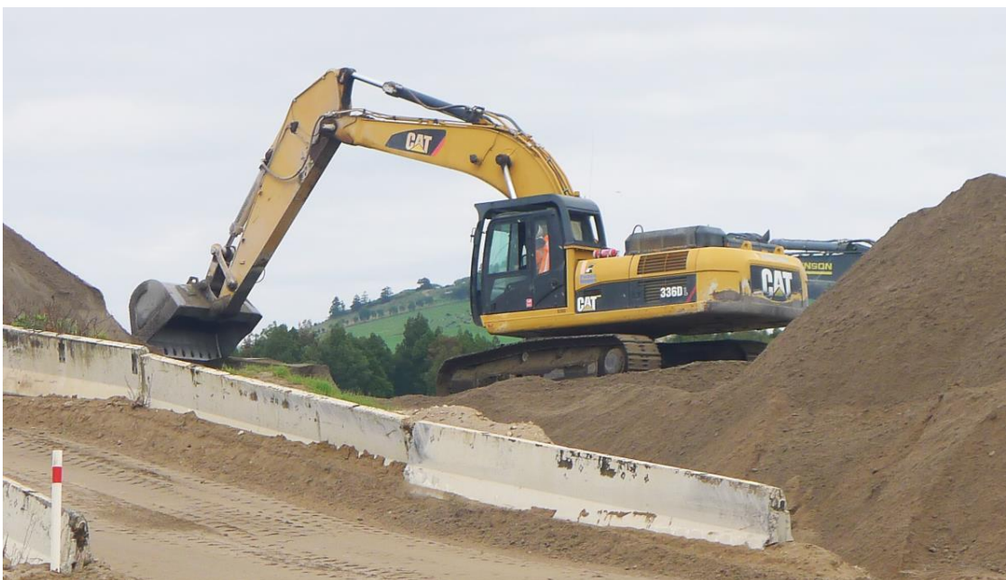
Figure 9. Cat 336D excavator
