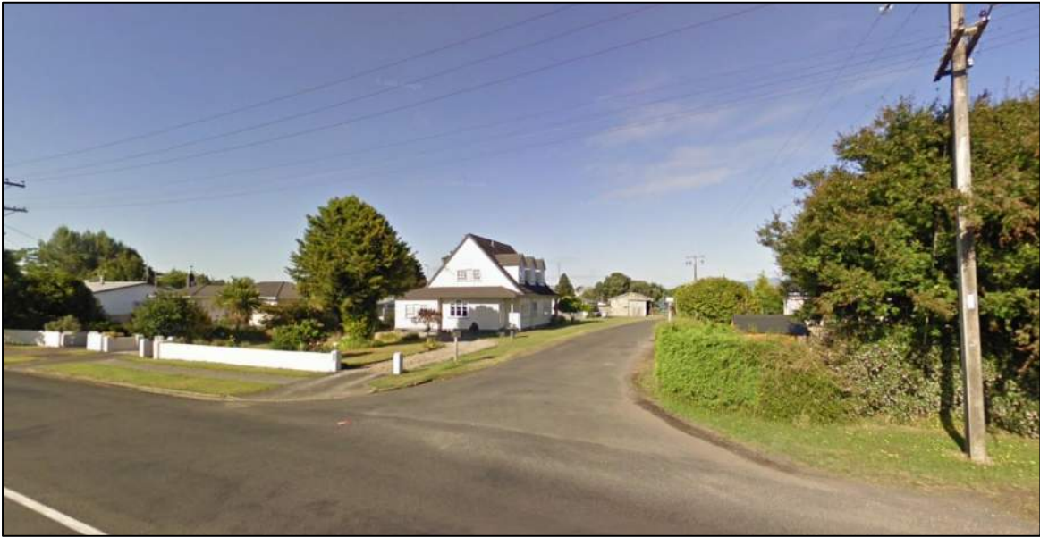
Figure 6: Existing access entrance
