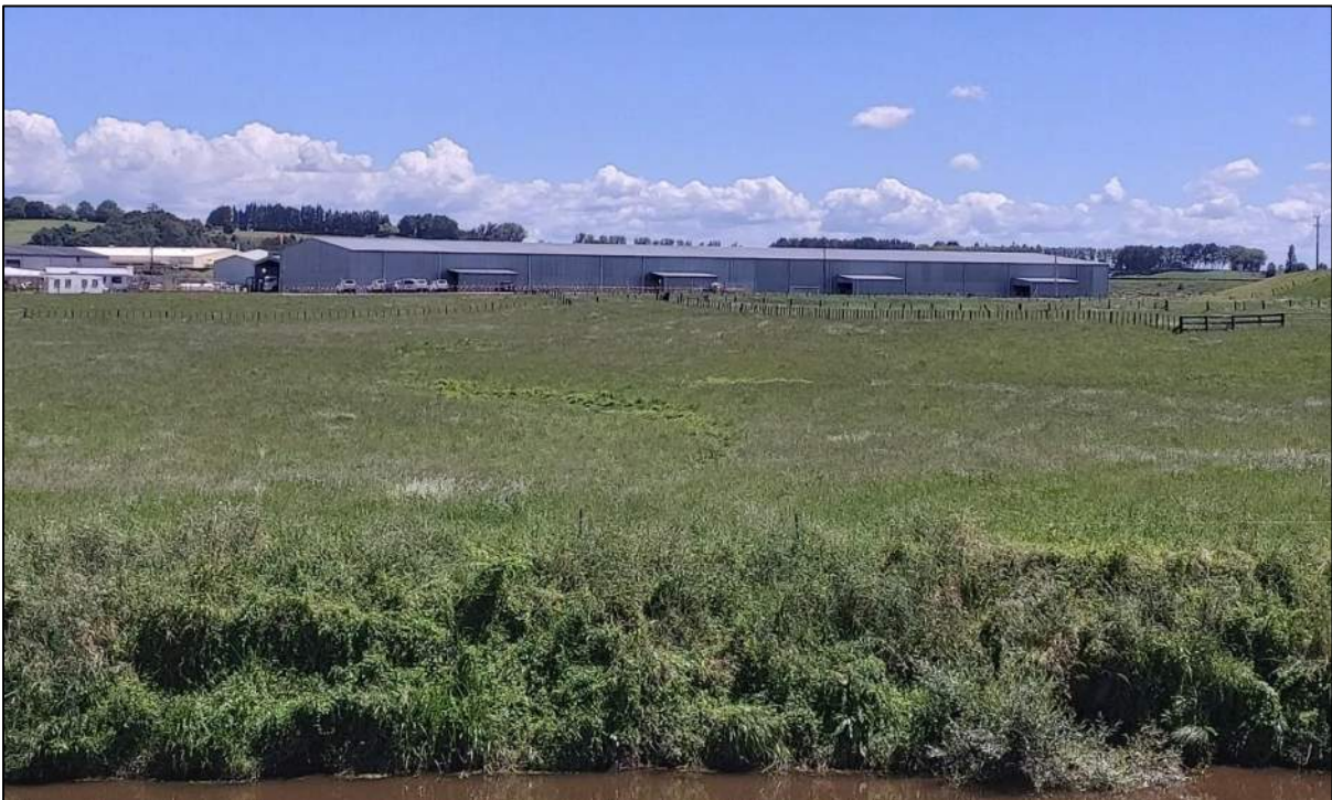
Figure 59: Fonterra Dry Goods Store
