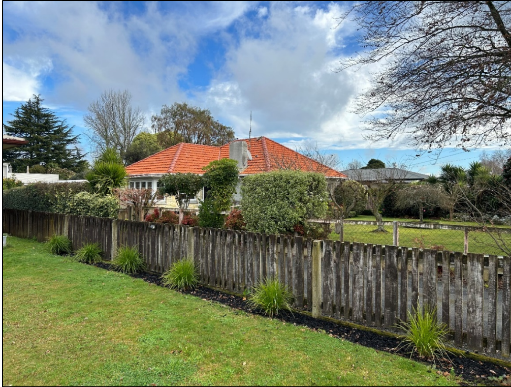
Figure 14: Site visit photo showing adjoining dwelling at 153 Taylor St.
