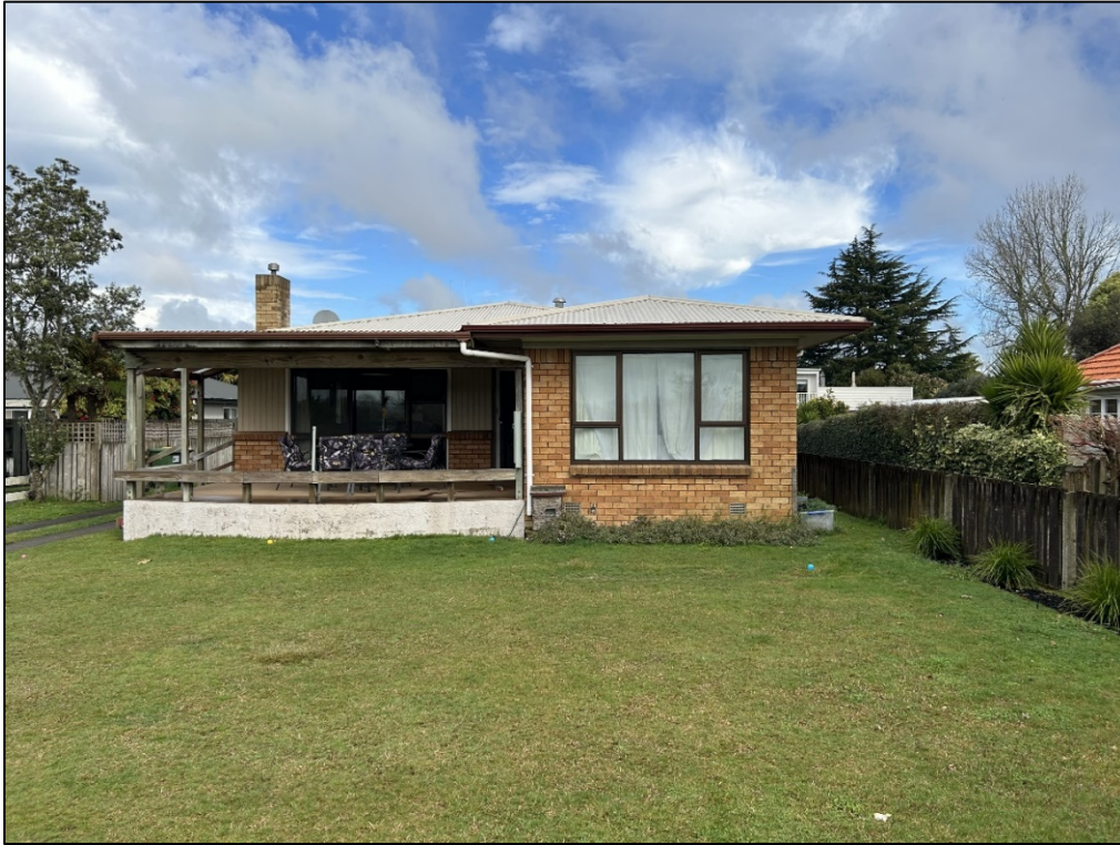
Figure 7: Site visit photo showing front yard of subject site and existing dwelling.
